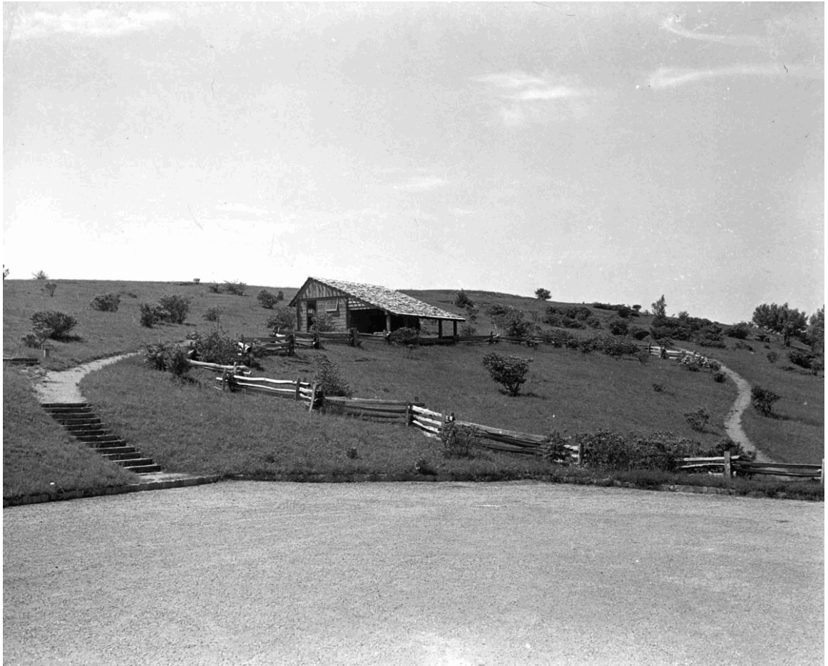
Picnic Area Comfort Station and Shelter - building # 102 (pre-1956)
