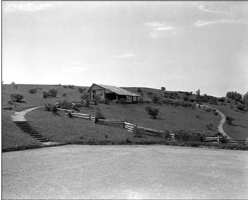
Fig 8-14. Picnic Area Comfort Station and Shelter - Building # 102 (pre-1956)
