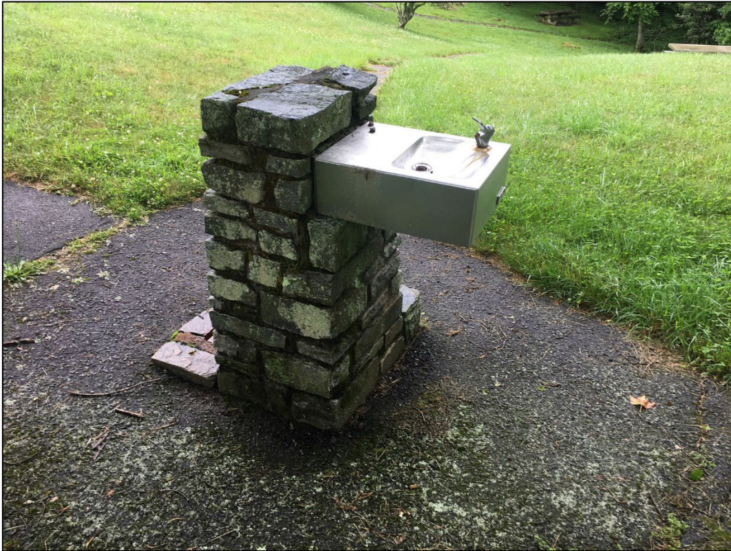
Fig 8-19. Stone drinking fountain near Mission 66-era picnic sites. Camera facing south (2021)
