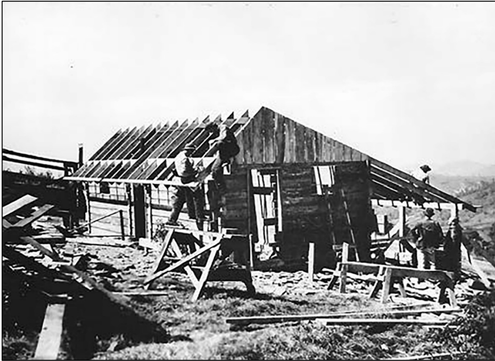
Fig 6-6. Construction of comfort station, Bluffs Picnic Area, 1940, Neg. #10,004, Class. #069.24, BLRI Archives.
