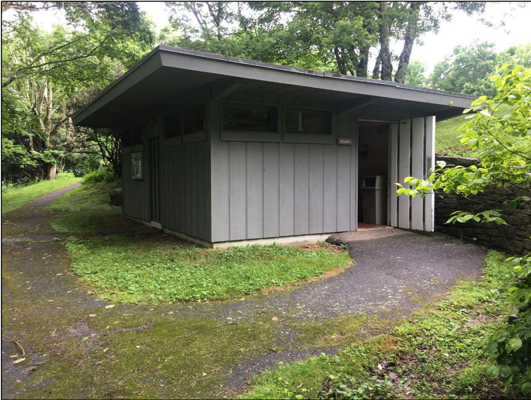
Fig 8-15. Oblique view of Comfort Station # 104. Camera facing north (2021)
