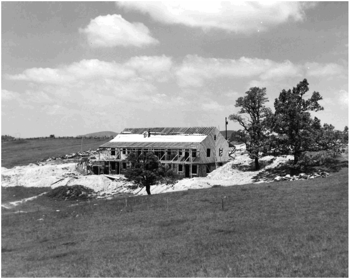
Bluffs Lodge during construction circa 1949
