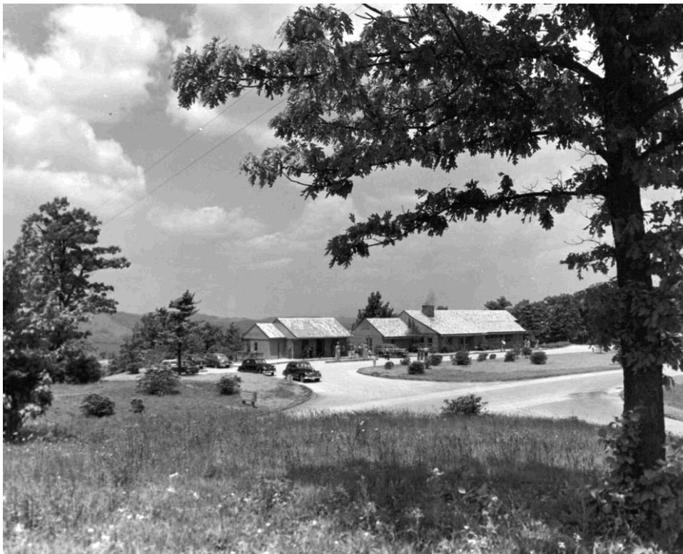
Bluffs Coffee Shop and Service Station area circa 1949
