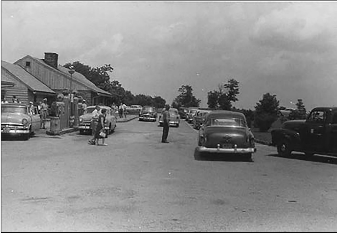
Fig 6-6. Bluffs Coffee Shop and Service Station Parking, 1956, Neg. #575, Class. #306.1, BLRI Archives.
