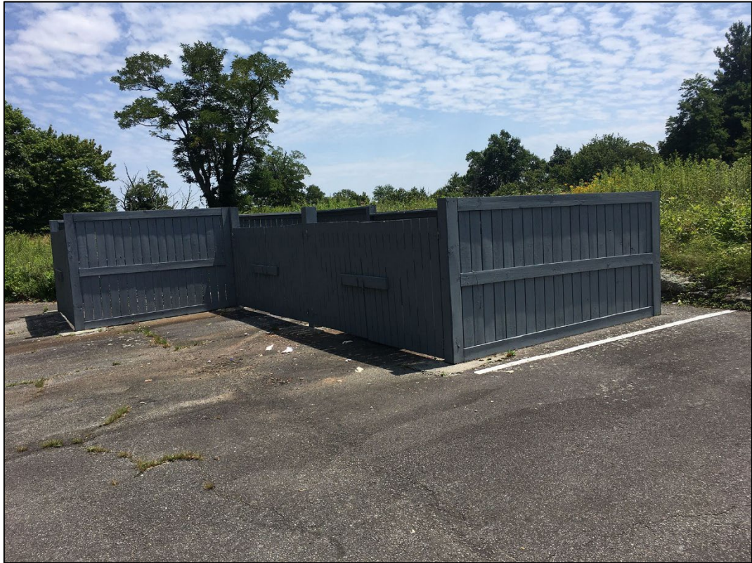
Fig 8-27. Refuse containment area at east end of east parking lot (2021)
