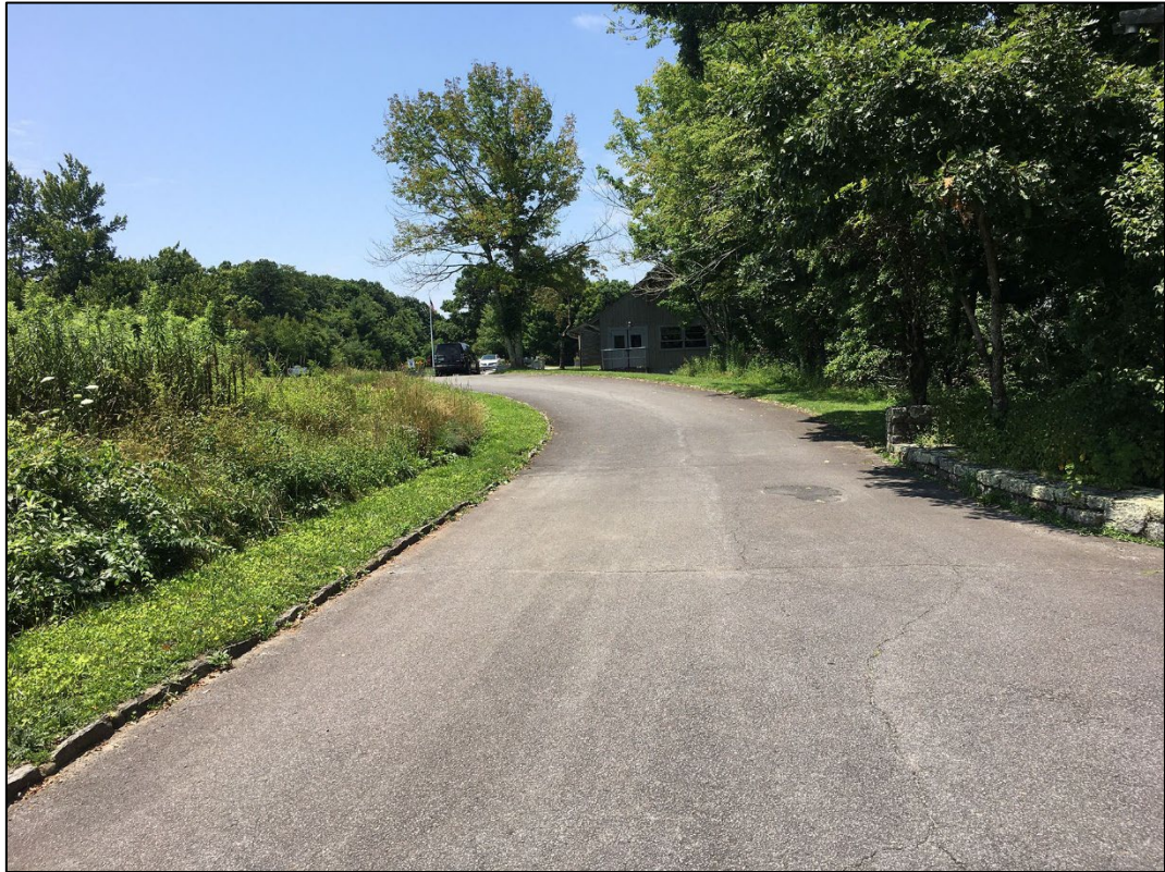
Fig 8-12. View of entrance to east parking lot, facing west (2021)
