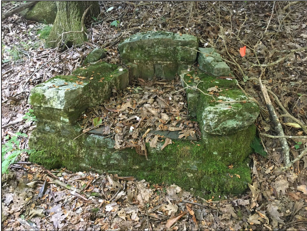
Fig 8-28. Structurally intact stone fireplace in abandoned segregated picnic area (2021)
