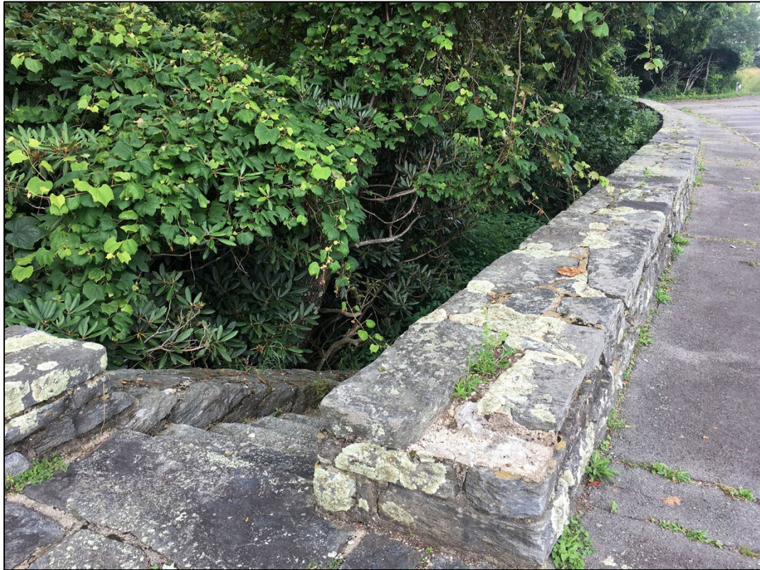
Fig 8-22. West end of stone retaining wall with view down stone steps leading to abandoned segregated picnic area (2021)
