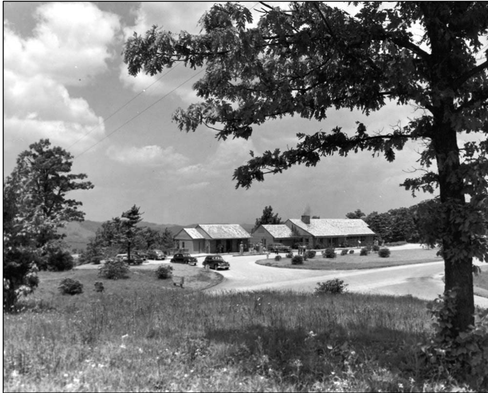
Fig 8-16. Bluffs Coffee Shop and Service Station area circa 1949
