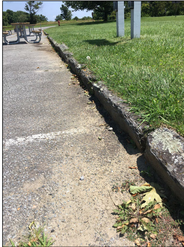
Fig 8-14. Stone curbing on south side of central access lane near Bluffs Coffee Shop (2021)
