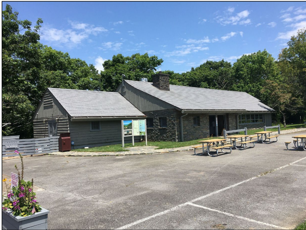
Fig 8-18. Oblique view of Bluffs Coffee Shop, south façade, facing northeast (2021)
