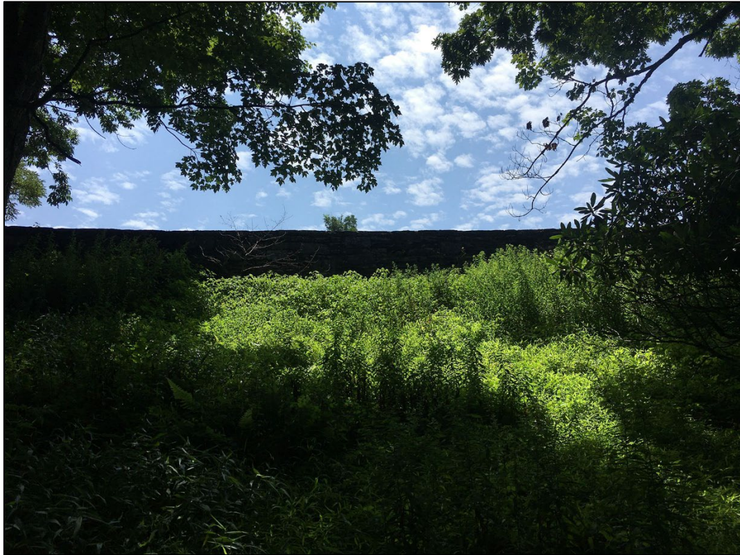
Fig 8-1. View of stone retaining wall from abandoned segregated picnic area, facing south (2021)
