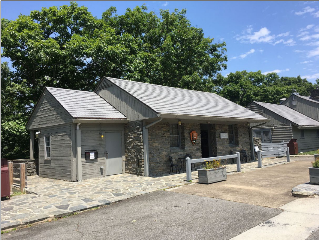
Fig 8-19. Oblique view of Bluffs Gift Shop, south façade, facing northeast (2021)
