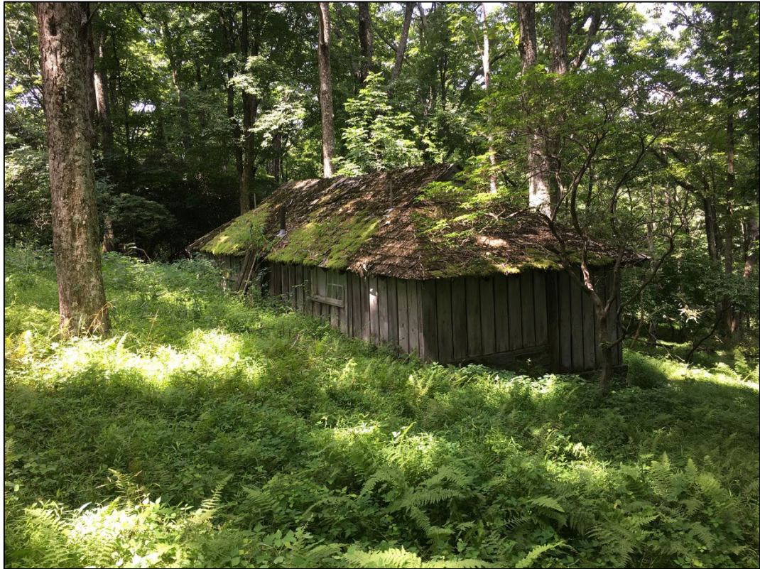
Fig 8-20. Oblique view of Comfort Station #101, south façade, facing northwest. Mature specimen mountain laurel visible on left side of frame (2021)
