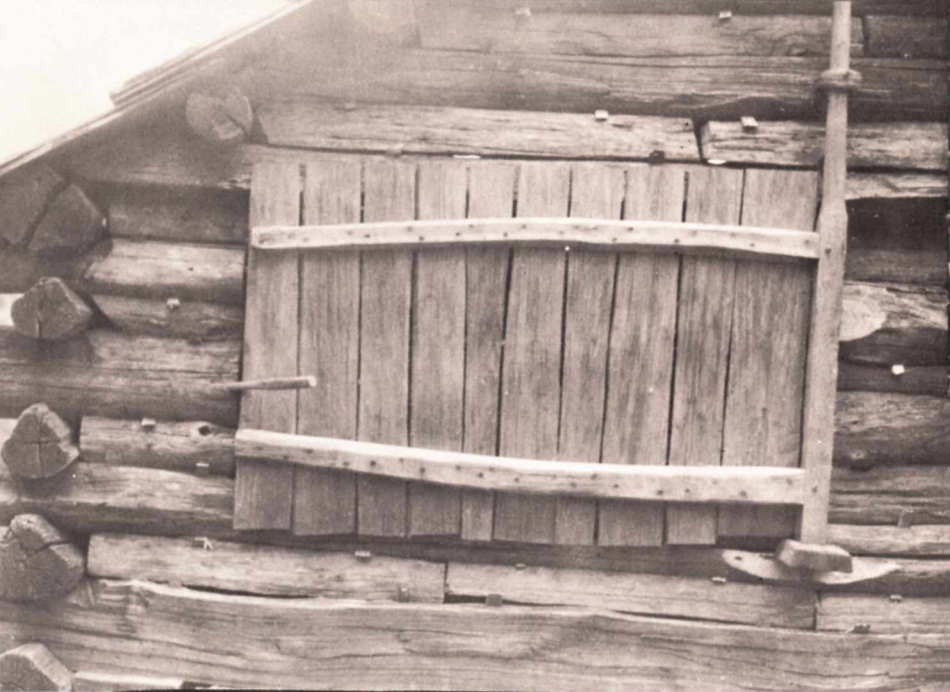
Gear loft door, note locust pegs and method of hinging.
