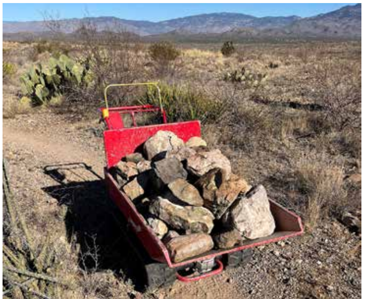
Utilizing a power carrier for transporting heavy rocks to repair the AZT along Las Cienegas (Passage 7)
