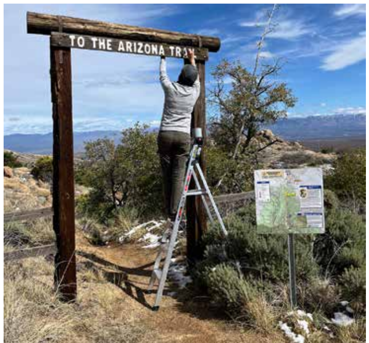
Improvements at High Jinks Ranch along Oracle Ridge (Passage 12), including interpretive sign installation and wooden sign repainting
