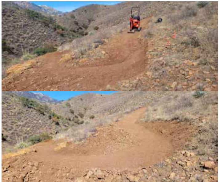
Top: Flagline Trails performing mechanized trail construction and maintenance along Casa Blanca Canyons (Passage 4) Bottom: Finished trail!
