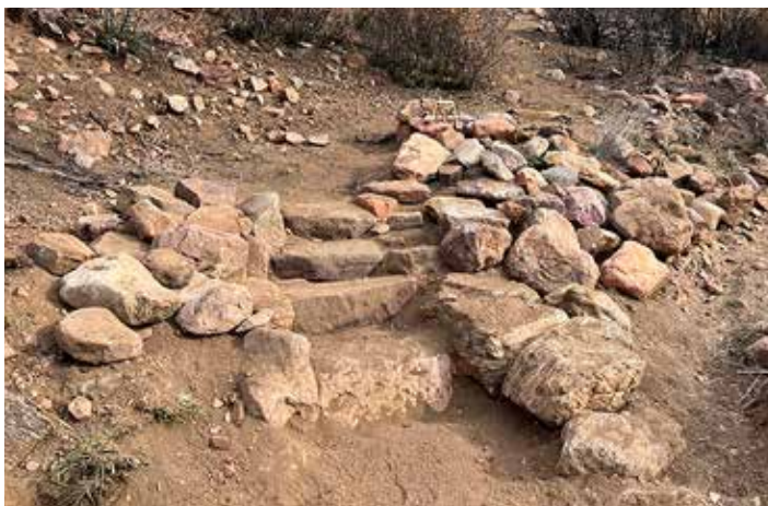
Installation of rock steps and rock armoring by ACE along Passage 19 in Cottonwood Canyon
