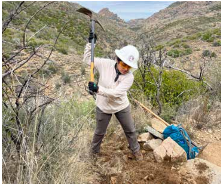
American Conservation Experience (ACE) crew performing tread maintenance along Passage 19 in the Superstition Wilderness
