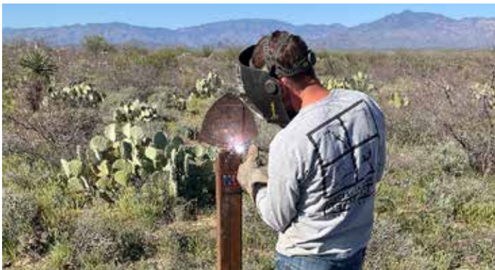
Remote field welding to repair signs along Las Cienegas (Passage 7)
