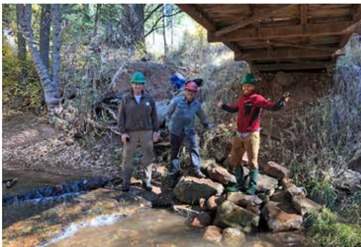
ATA volunteers performing rock armoring to protect trail bridge along Highline (Passage 26)
