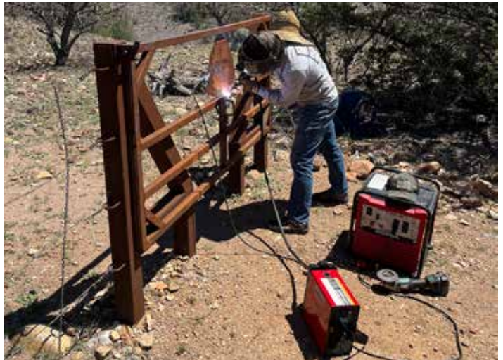
Remote field welding of AZT supergate along Casa Blanca Canyons (Passage 4)
