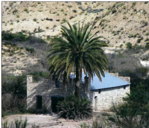
Hot Springs Post Office
