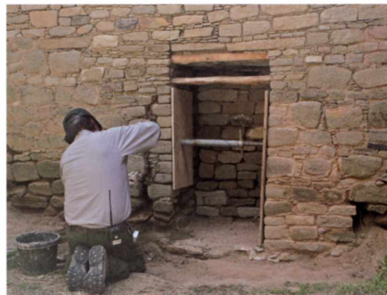
Masonry worker Ernest Harrison repairing an ancient doorway
