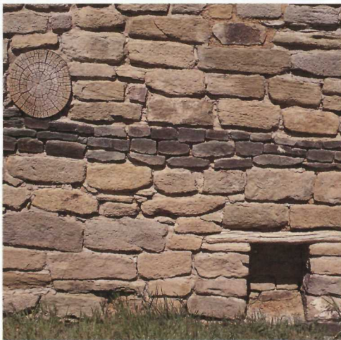
Two bands of green sandstone—at ground level and waist high—run along a West Ruin wall. Their purpose remains a mystery.
