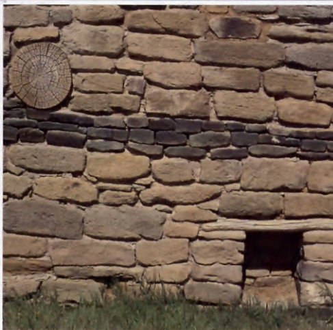
Two bands of green sandstone—at ground level and waist high—run along a wall of the West Ruin.
