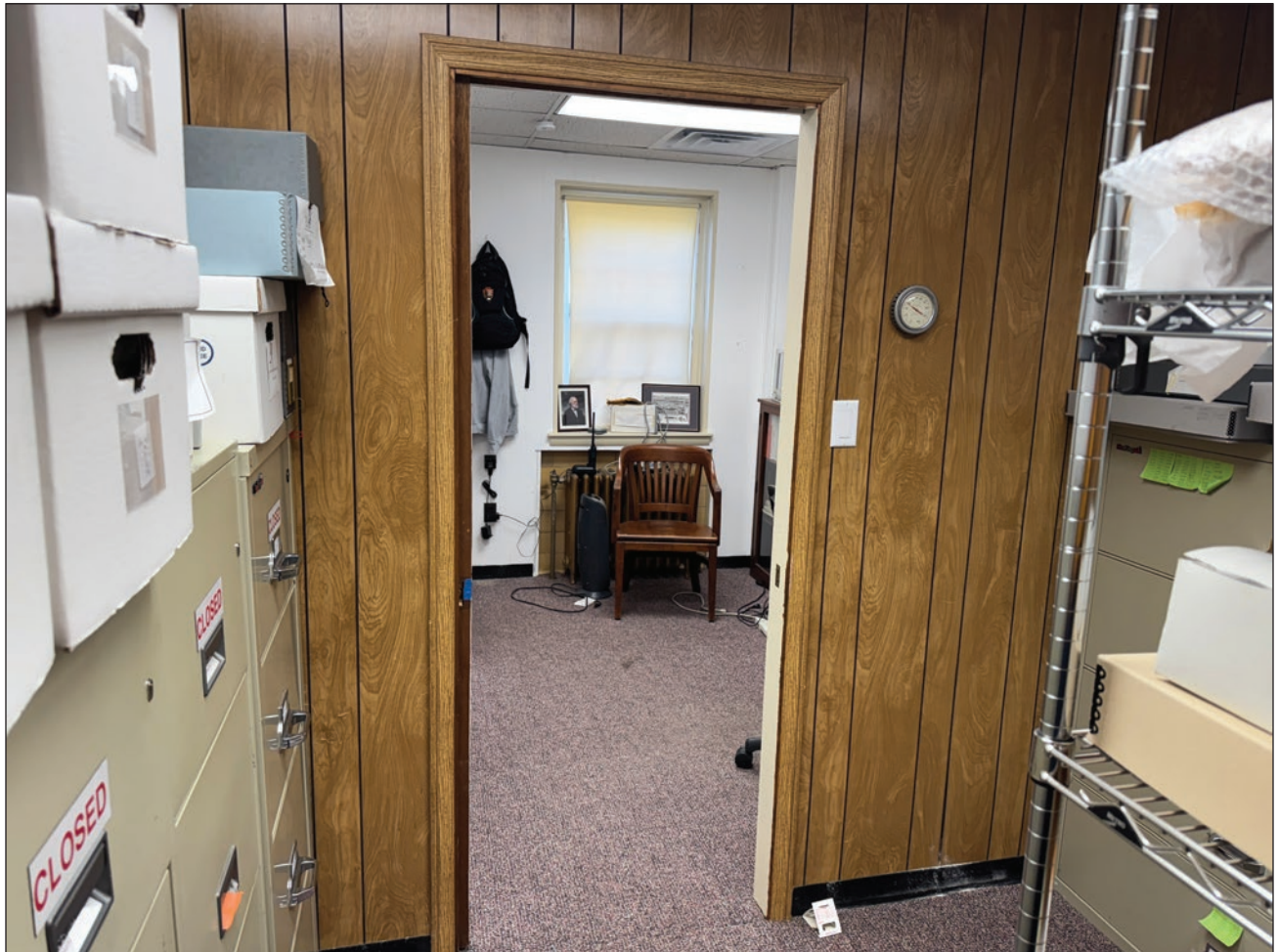
Figure 192. Unpainted HDF paneling and door frame in east section of north room. Building Conservation Associates, 2025.
