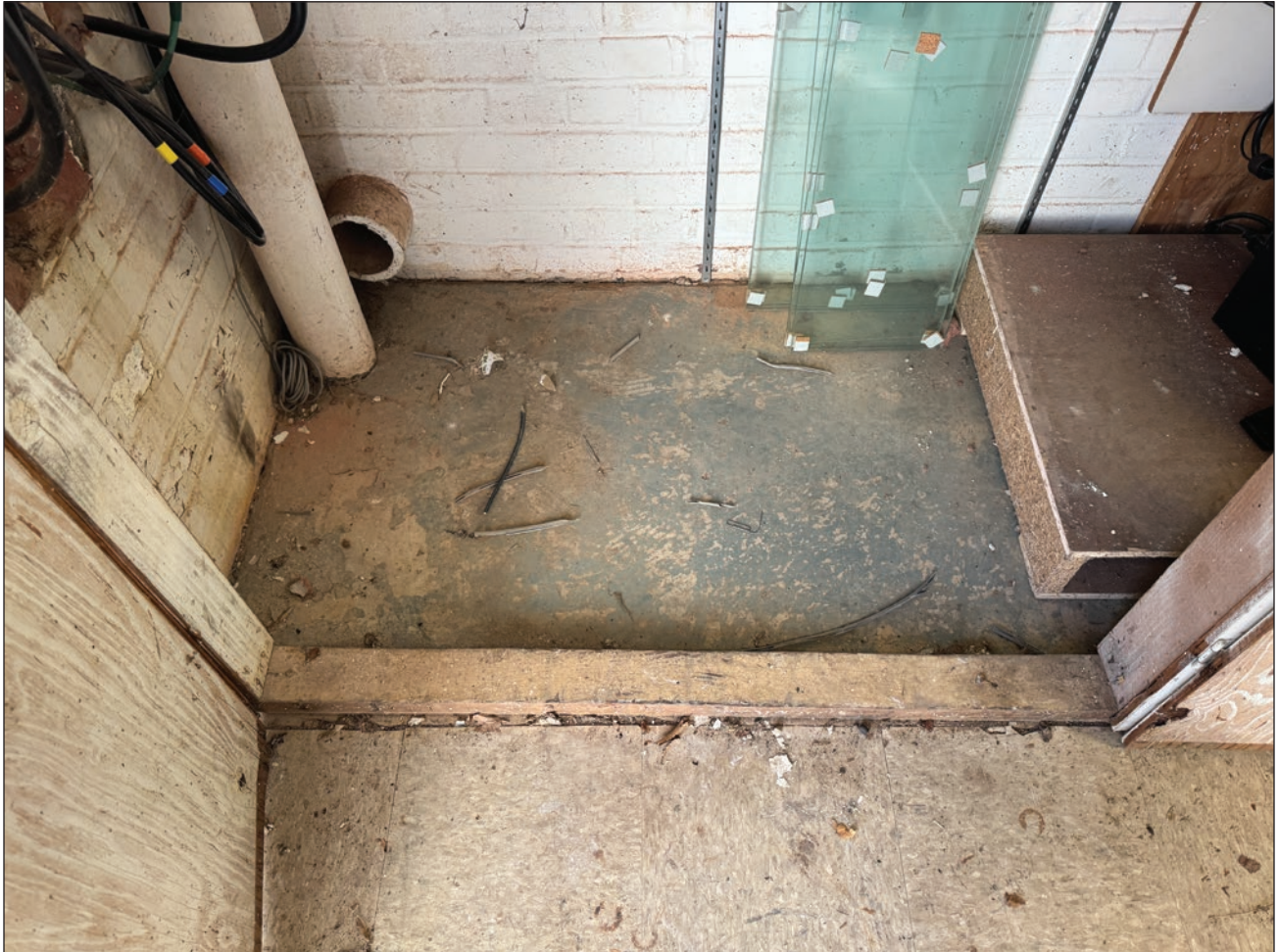
Figure 256. Exposed concrete floor in north basement room. Building Conservation Associates, 2025.
