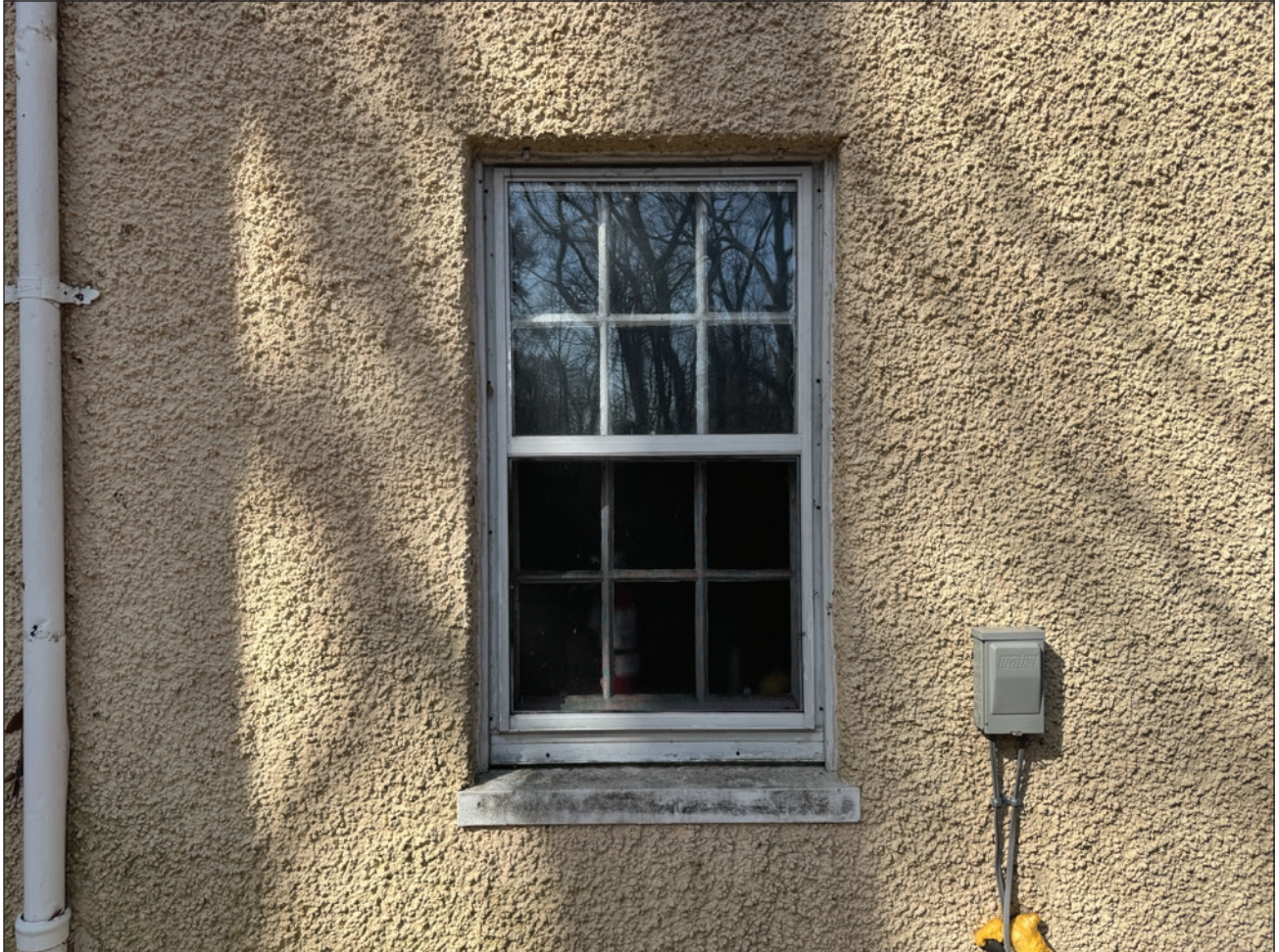
Figure 122. Basement window at east elevation. Building Conservation Associates, 2025.
