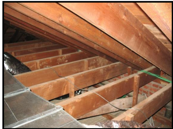
Photo P-6: Roof rafter and tie beam framing
