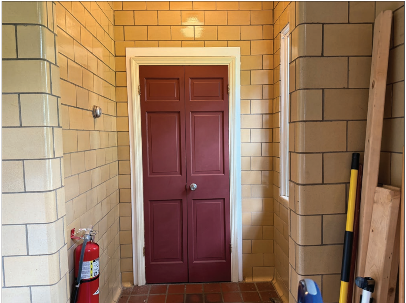
Figure 186. South door in the vestibule. Building Conservation Associates, 2025.
