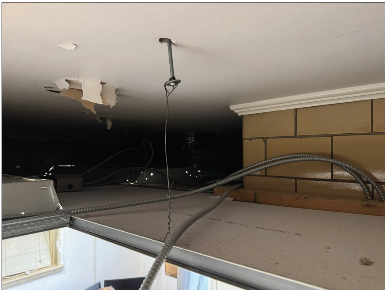
Figure 181. View above the suspended ceiling in the south room. Building Conservation Associates, 2025.
