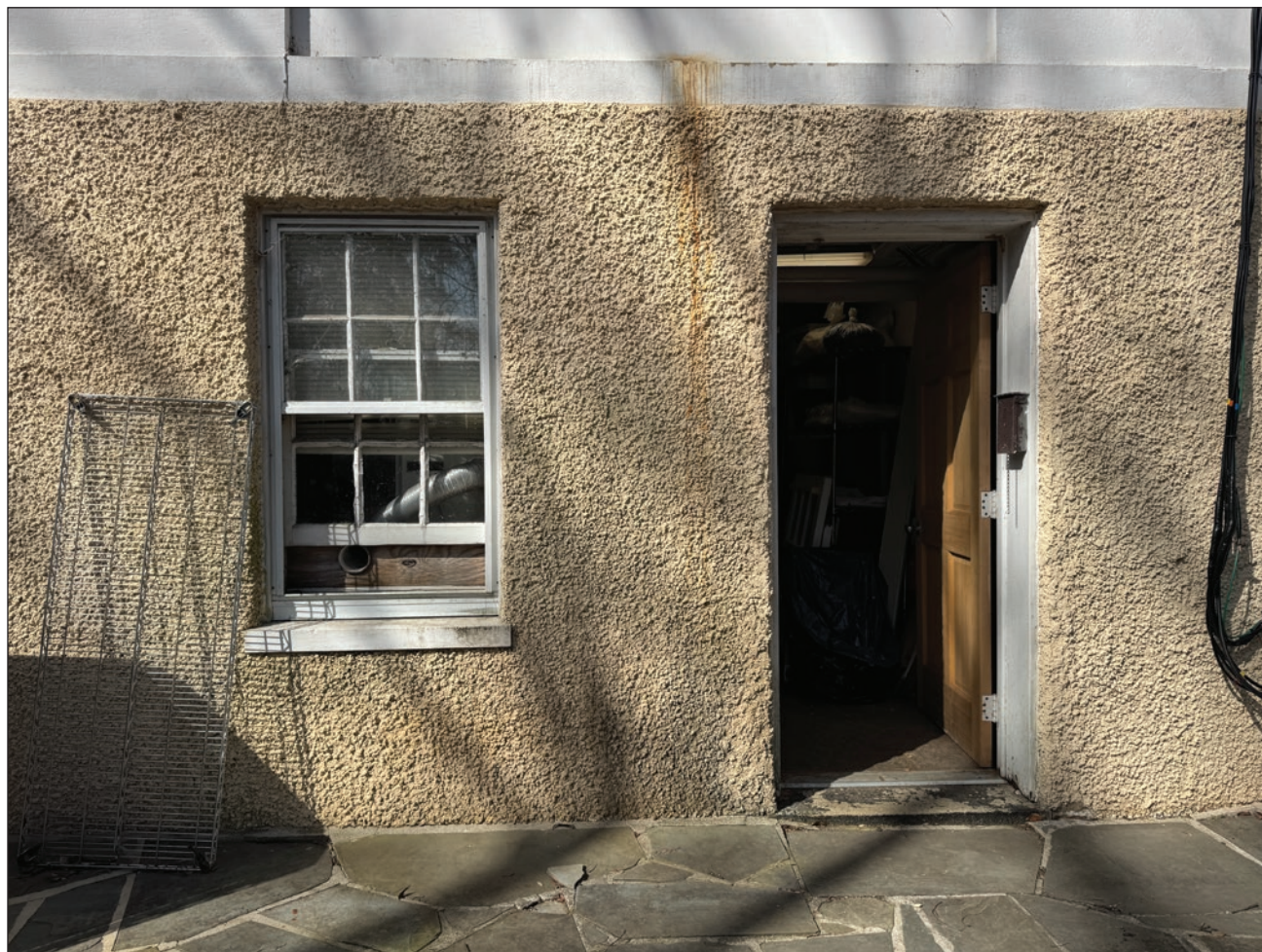
Figure 148. The center of the east elevation showing modifications made to the original windows. Building Conservation Associates, 2025.
