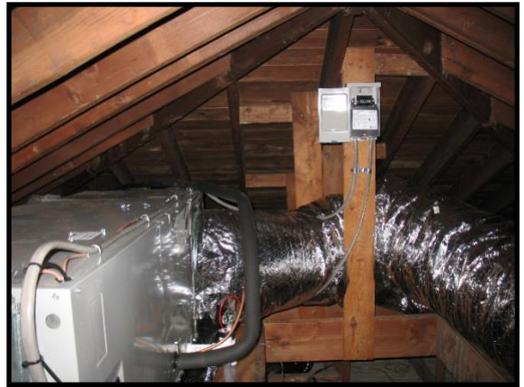
Photo P-10: Roof tie beam hangers – looking south
