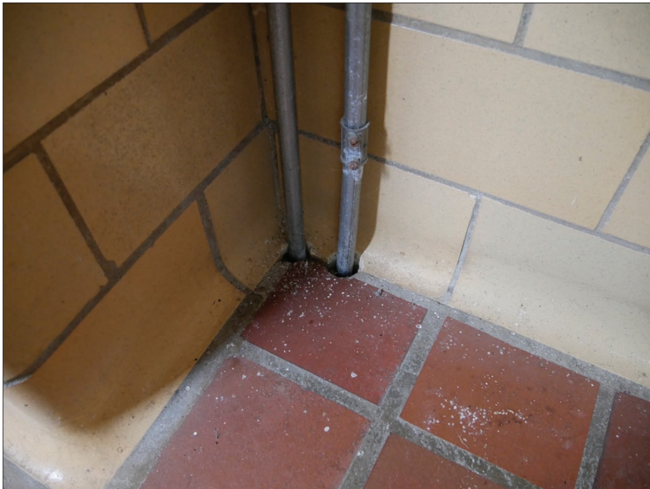
Figure 257. Holes for conduit in tile floor in vestibule. Building Conservation Associates, 2025.
