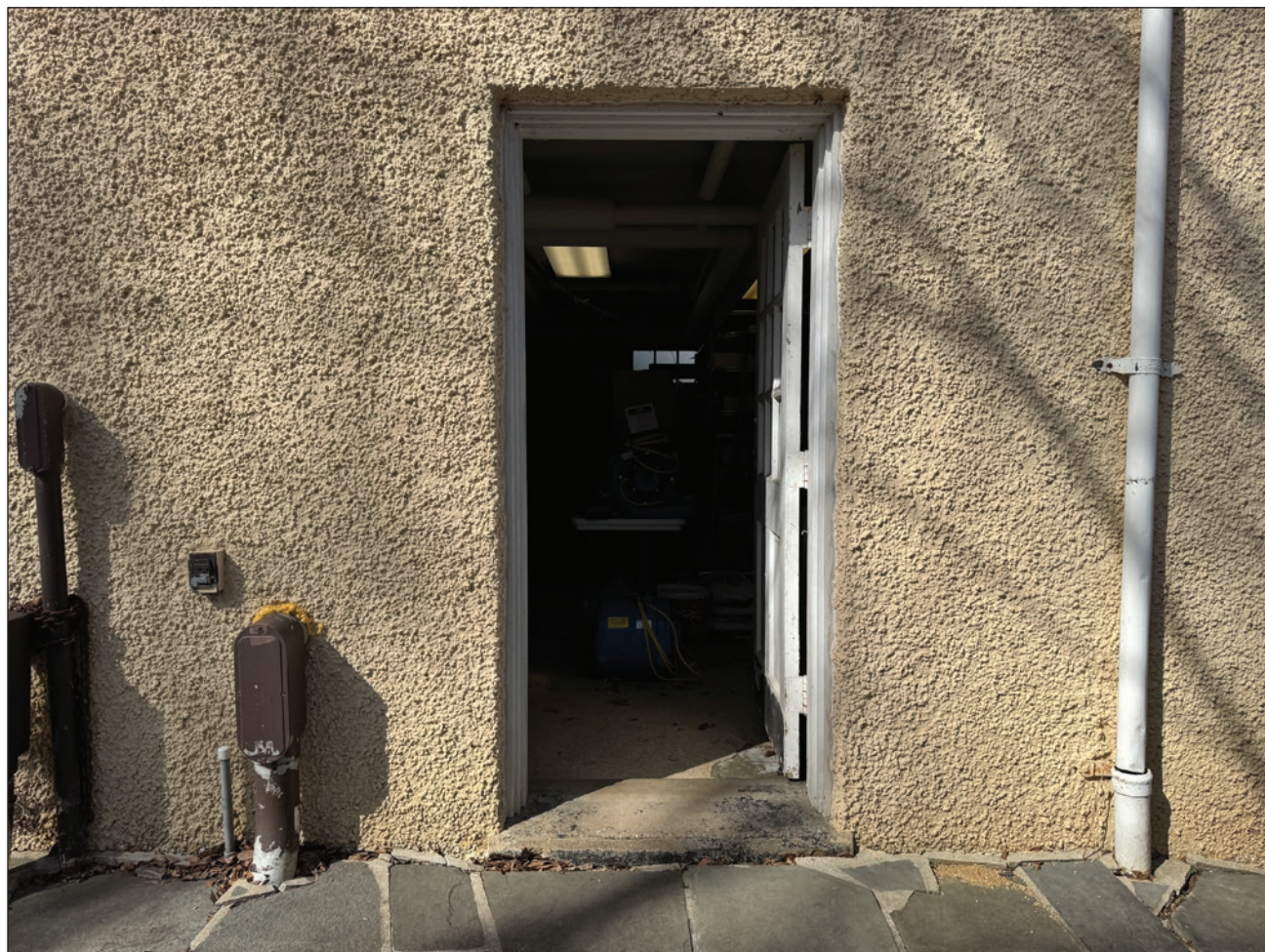
Figure 154. North door on the east elevation. Building Conservation Associates, 2025.
