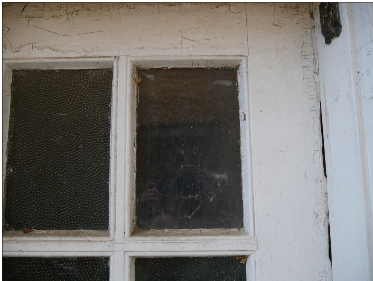
Figure 233. Replacement glass pane at southwest basement door. Building Conservation Associates, 2025.
