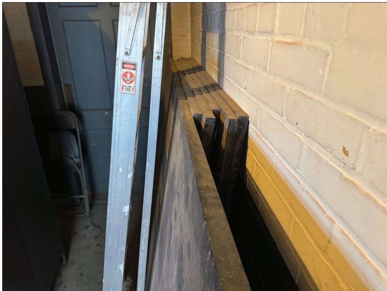
Figure 168. Slate toilet stall partitions in the southwest basement room. Building Conservation Associates, 2025.
