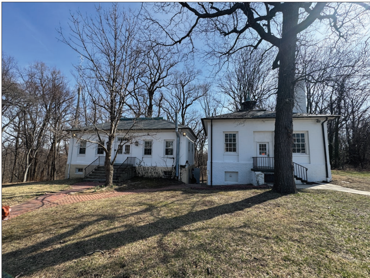
Figure 101. View looking east at Buildings #313 (left) and #314 (right). Building Conservation Associates, 2025.
