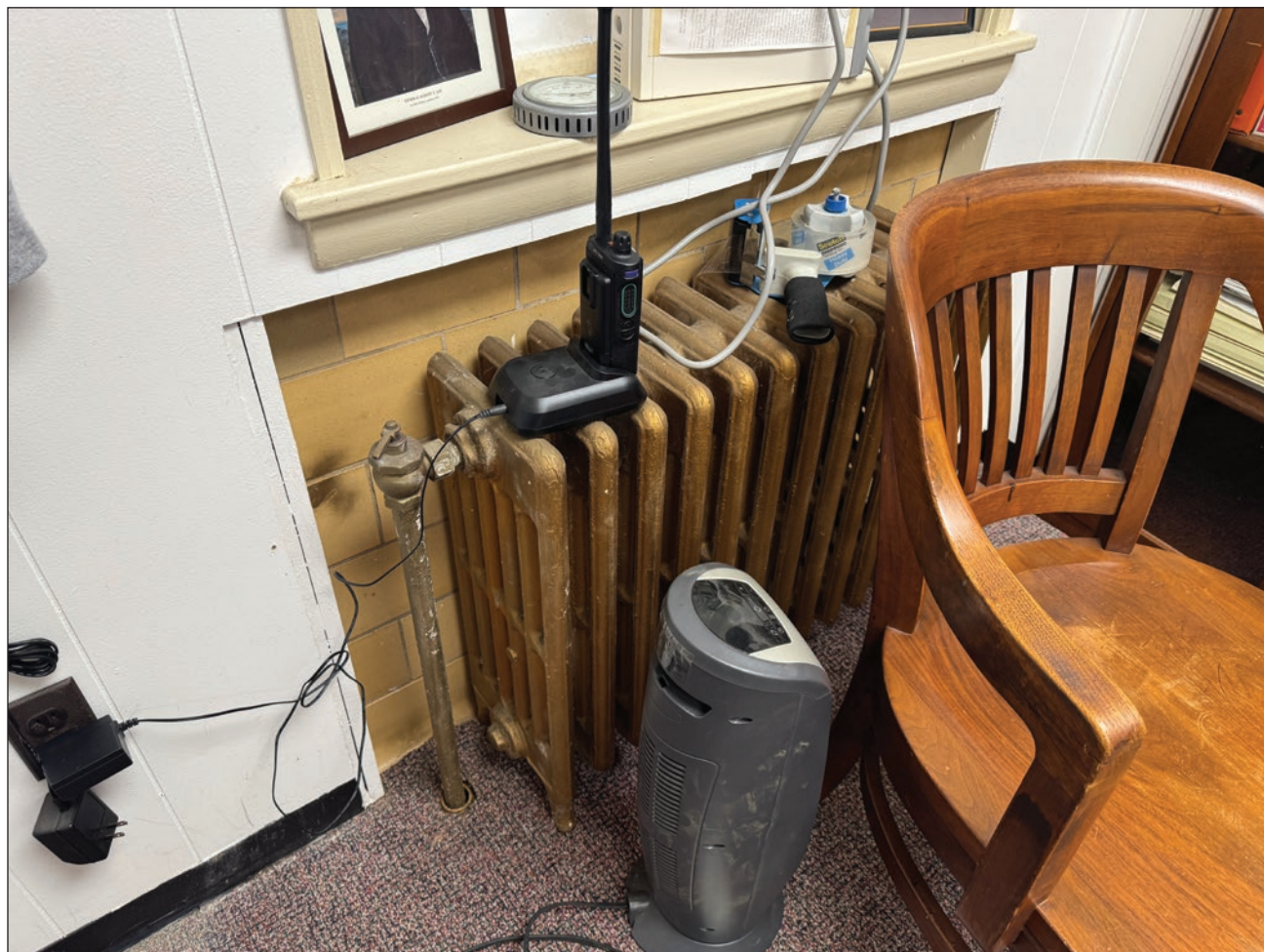
Figure 191. Original glazed tile wall on behind radiator in north room. Building Conservation Associates, 2025.
