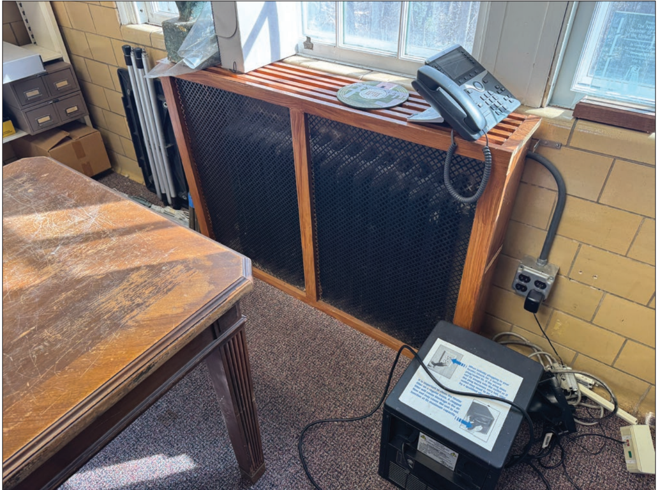
Figure 273. Wood and metal mesh radiator enclosure in first-floor east room. Building Conservation Associates, 2025.
