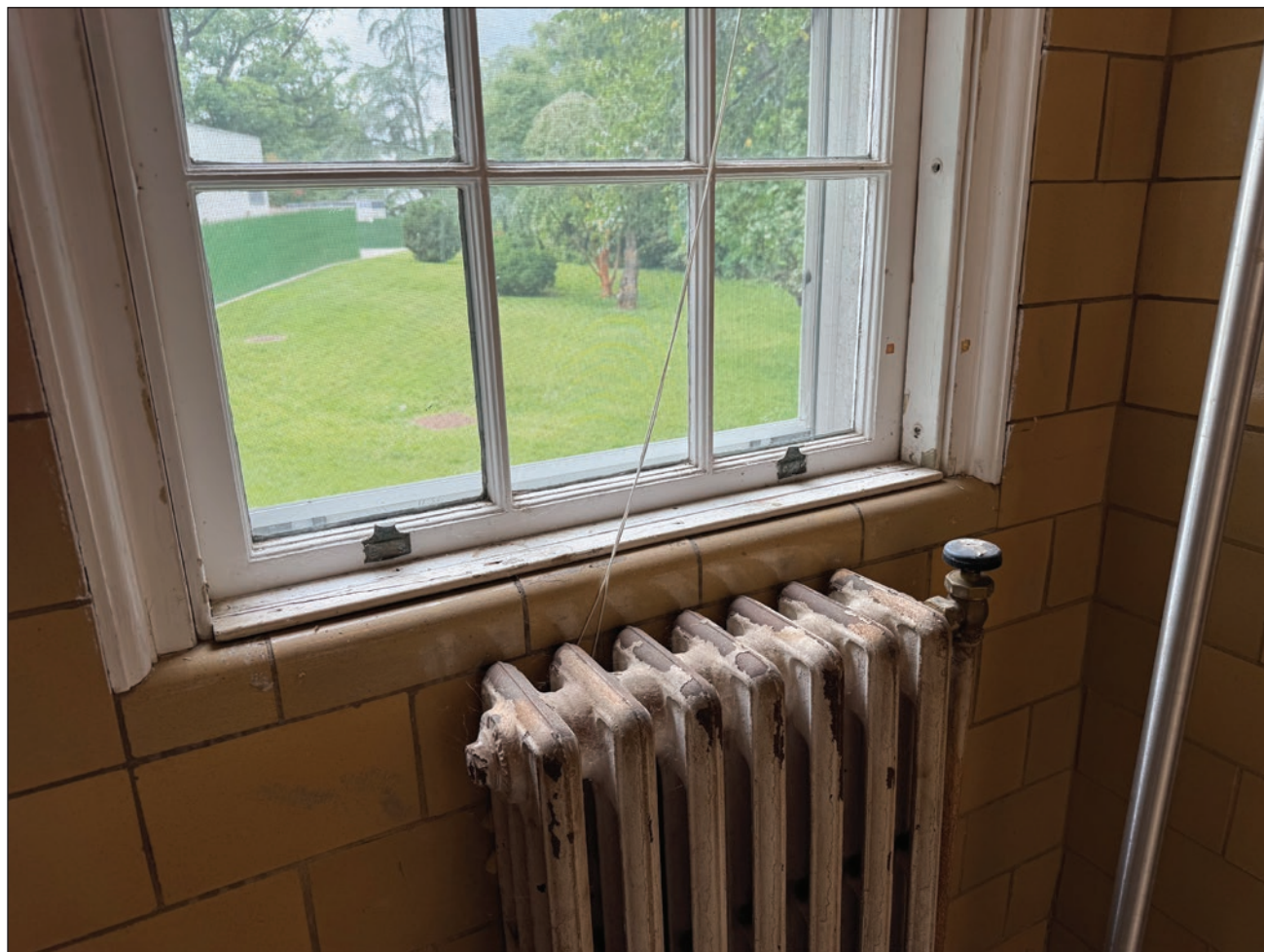
Figure 131. Bullnose glazed tile sill at west elevation window. Building Conservation Associates, 2025.
