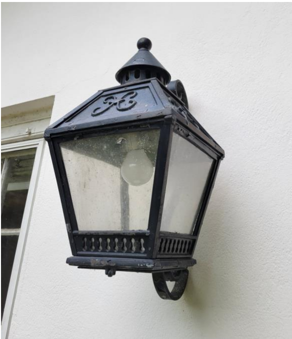
Photo E25: Front entrance wall sconces retrofitted with LED lamps.
