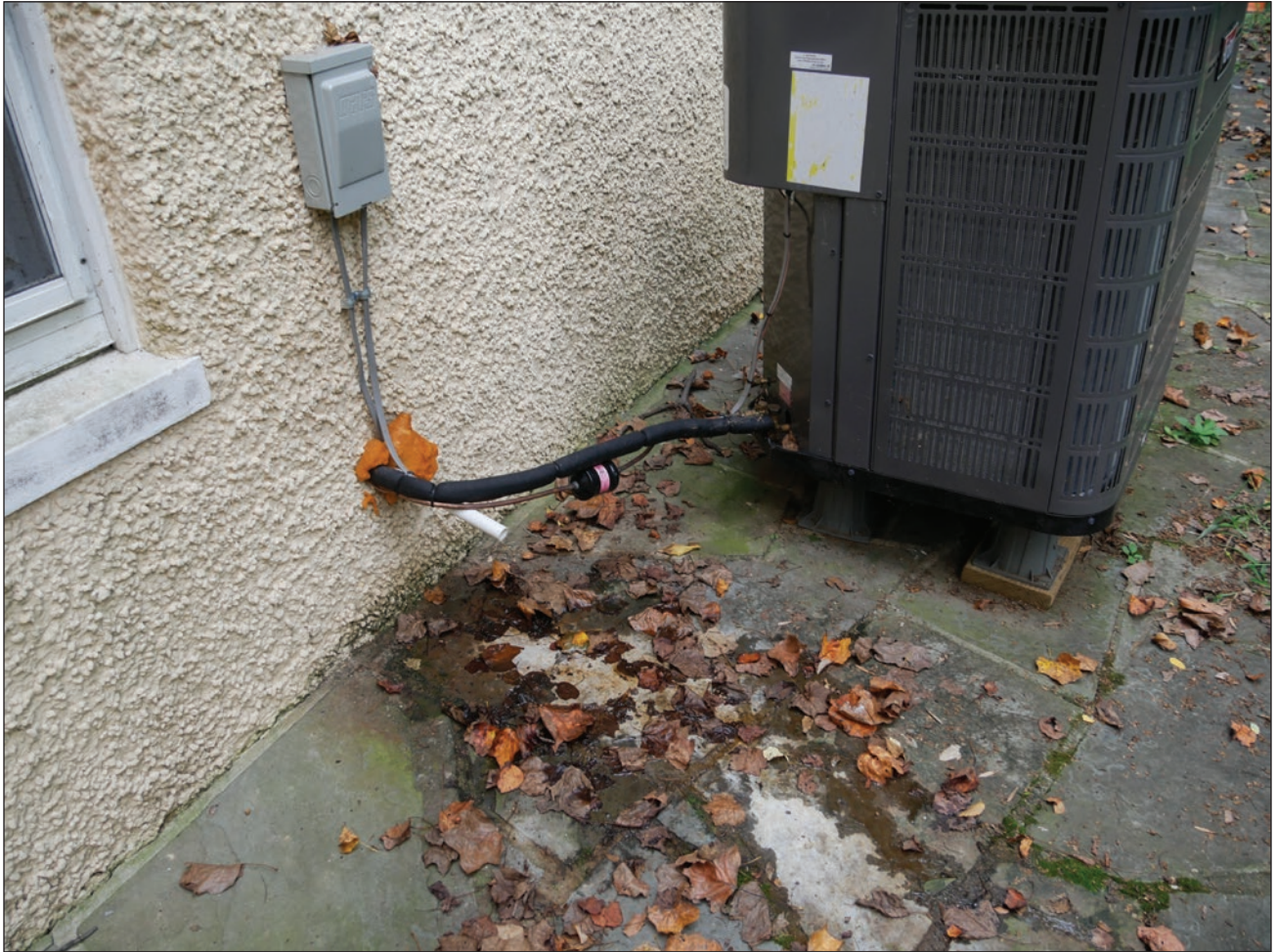
Figure 204. Foam sealant at the HVAC penetration in the pebble dash stucco at the east elevation. Building Conservation Associates, 2025.
