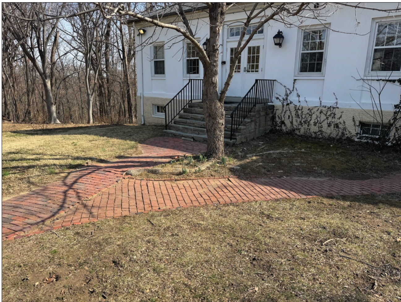
Figure 141. Brick walkways and large hackberry tree west of Building #313. View looking northeast. Building Conservation Associates, 2025.
