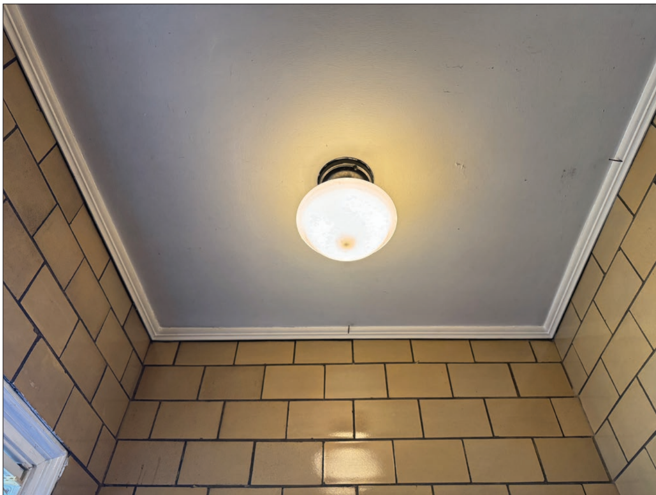
Figure 127. Suspended plaster ceiling with wood cornice in first-floor vestibule. Building Conservation Associates, 2025.
