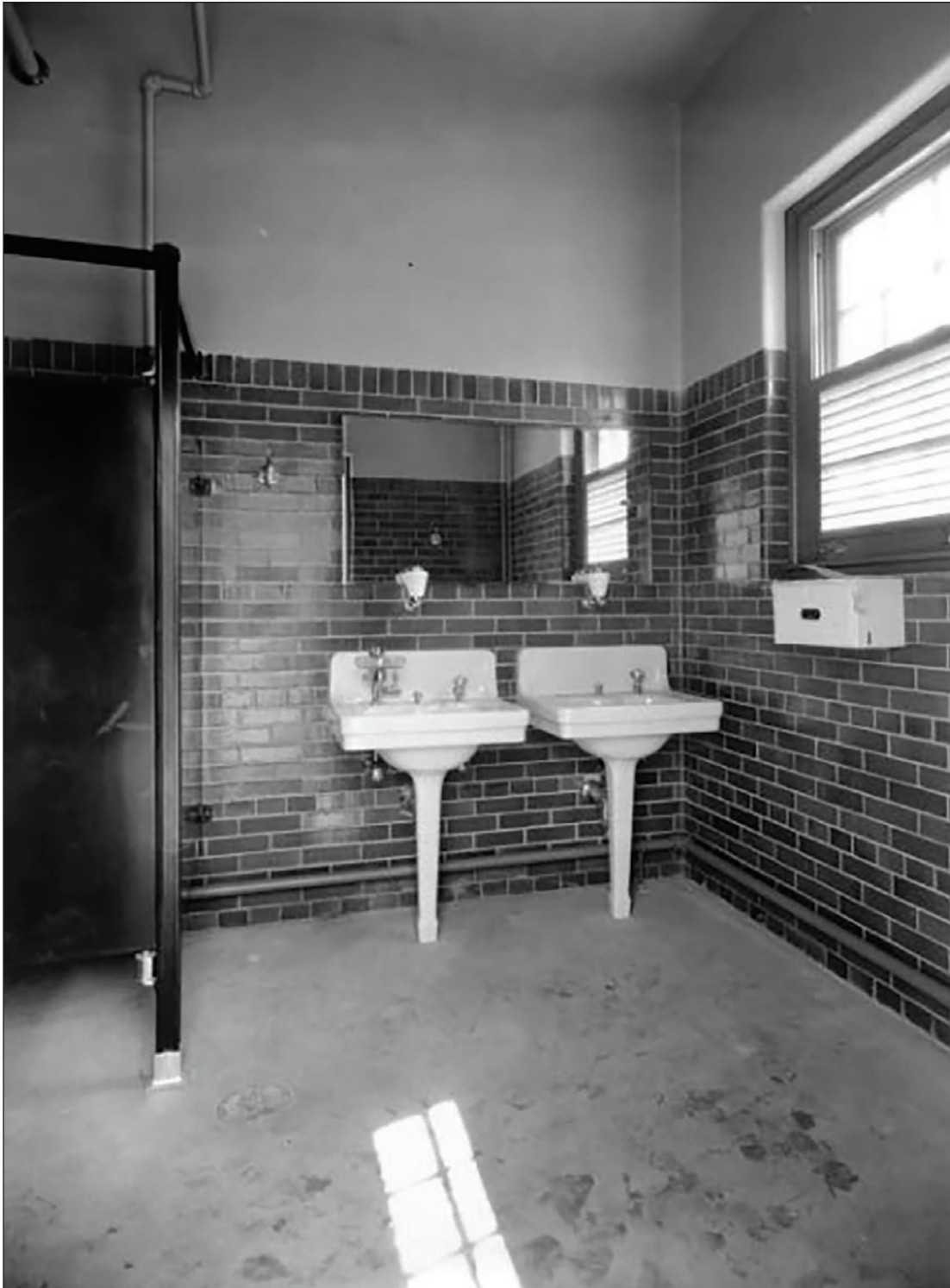
Figure 80. The "Colored men's toilet room" at Fredericksburg and Spotsylvania National Military Park, 1936. "Colored Men's Toilet Service Building," construction completion photograph, 14 April 1936, Chatham Manor Archives. Fredericksburg and Spotsylvania National Military Park, Fredericksburg, VA.
