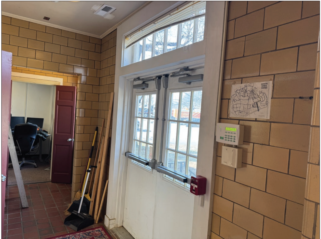
Figure 182. Main (west) entrance door. Building Conservation Associates, 2025.
