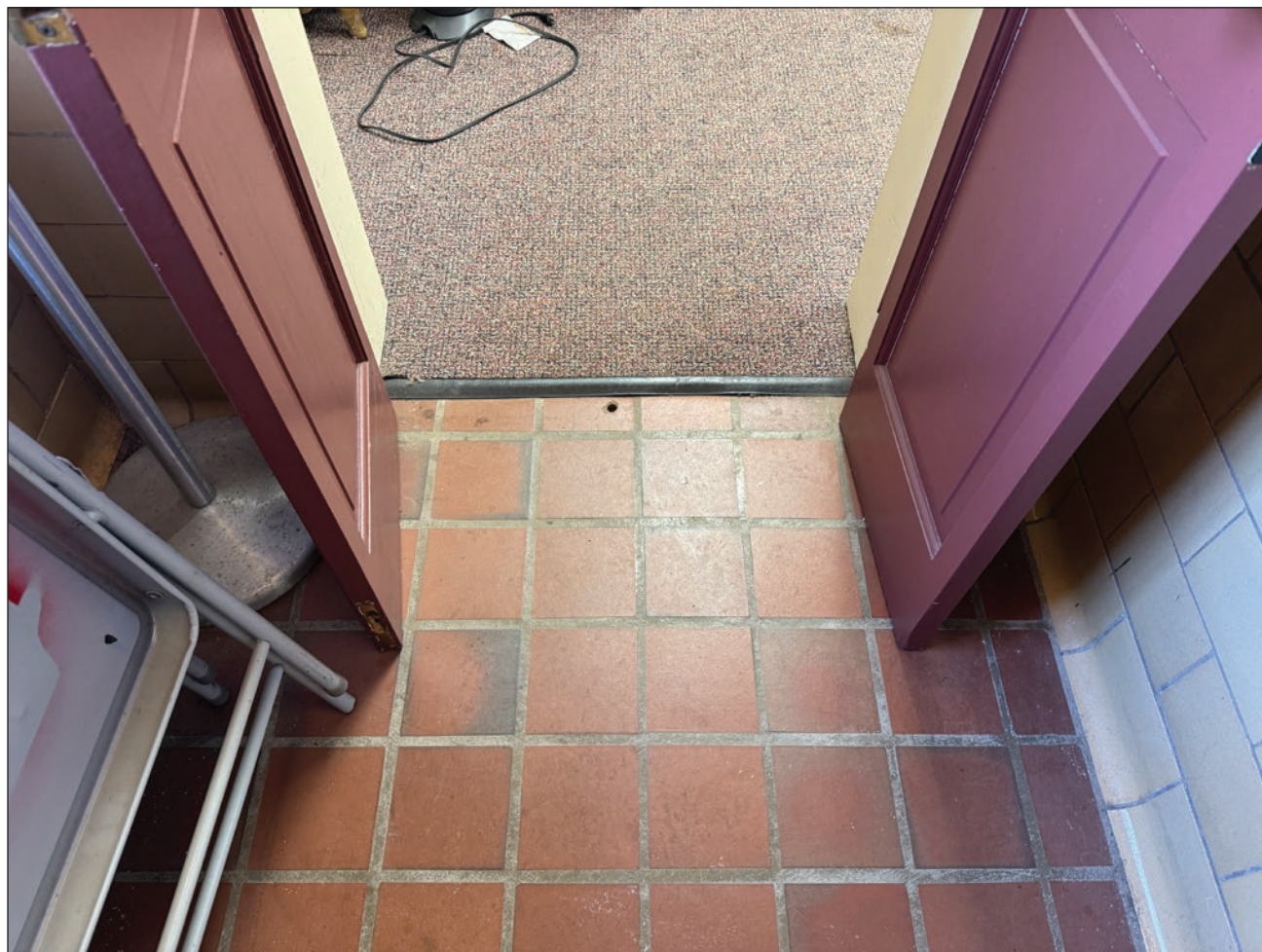
Figure 179. Quarry tile floor in vestibule and carpeting in the north room. Note also the hole in the floor for the flush bolt. Building Conservation Associates, 2025.
