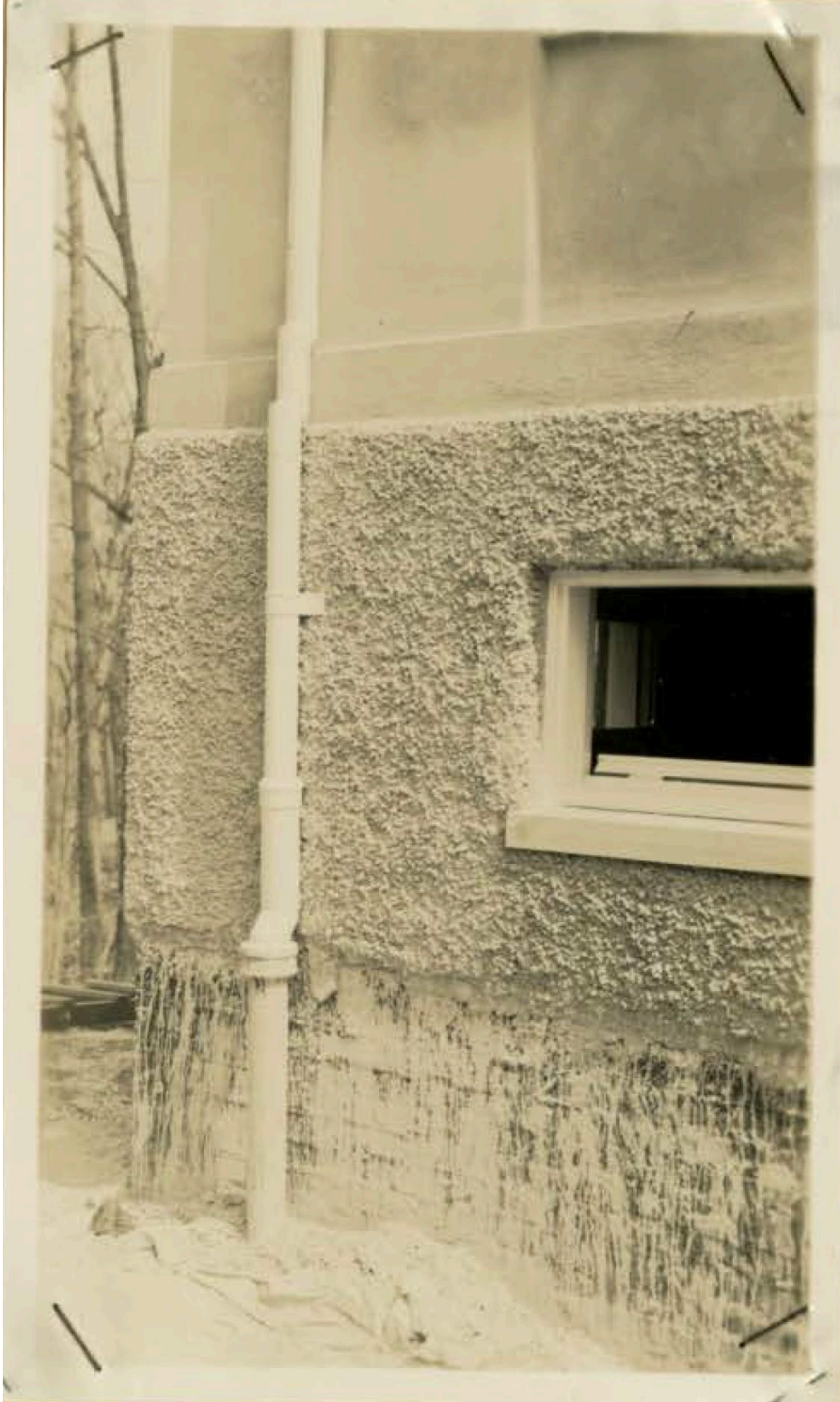
Figure 5. Photograph of exterior pebble dash finish after construction in 1941. Note the painted appearance of the pebble dash and the drip marks on the foundation below the pebble dash water table. (First Lt. Howard D. Nottingham, QMC, Completion Report for the Construction and Completion of the Comfort Station at Arlington National Cemetery, Fort Myer, Virginia, War Department, 1941, appendix.)
