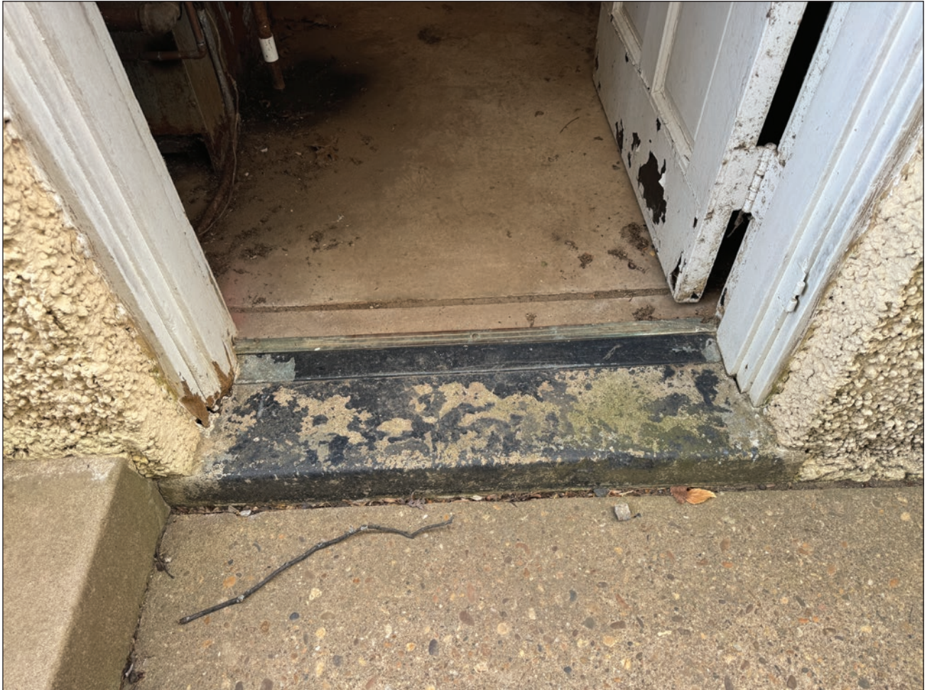
Figure 153. Black-painted concrete threshold at the entrance to the former segregated women's restroom. Building Conservation Associates, 2025.
