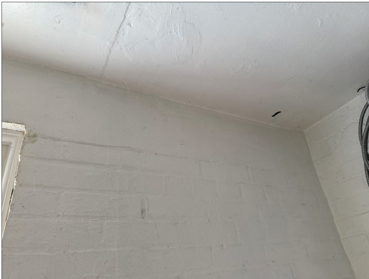
Figure 111. Concrete spandrel at the top of the basement south brick wall in the southeast former segregated toilet room. Building Conservation Associates, 2025.
