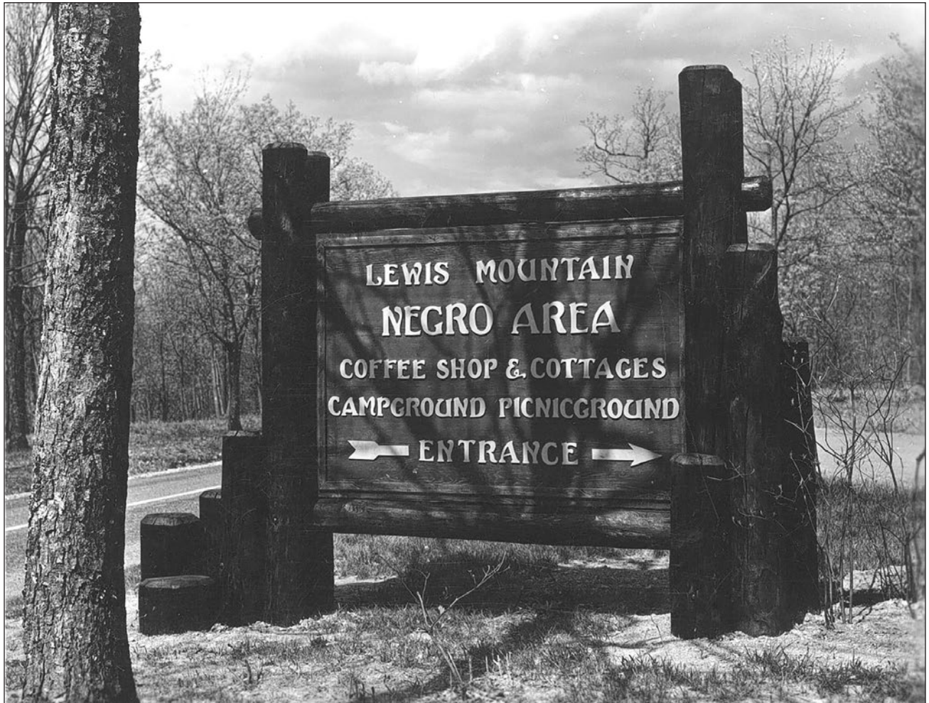
Figure 85. Sign for the segregated Lewis Mountain campground, 1936. Signs reading "For White Only" were posted elsewhere throughout the park. "Directional Sign, Shenandoah Resource Management Records, Luray, VA.
