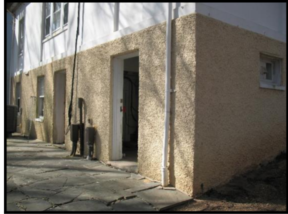
Photo P-4: Partial northeast building corner
