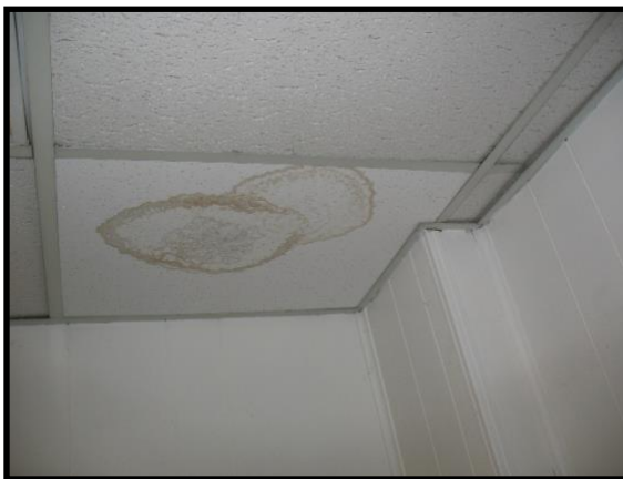
Photo P-15: Ceiling tile below location of repaired roof leak
