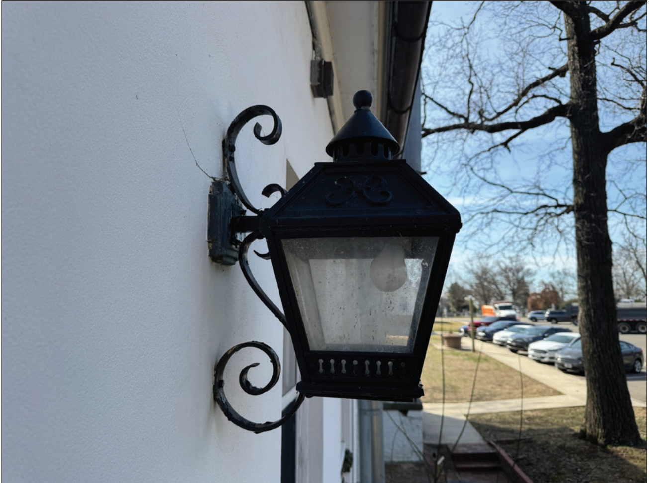
Figure 155. Decorative lantern sconce on west elevation. Building Conservation Associates, 2025.
