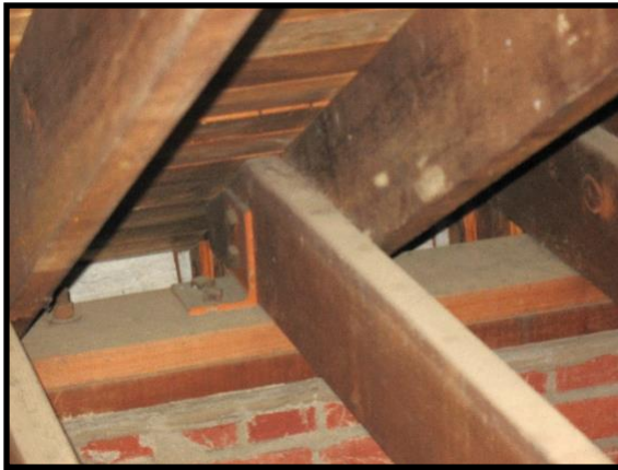
Photo P-9: Roof rafter and tie beam bearing at exterior wall
