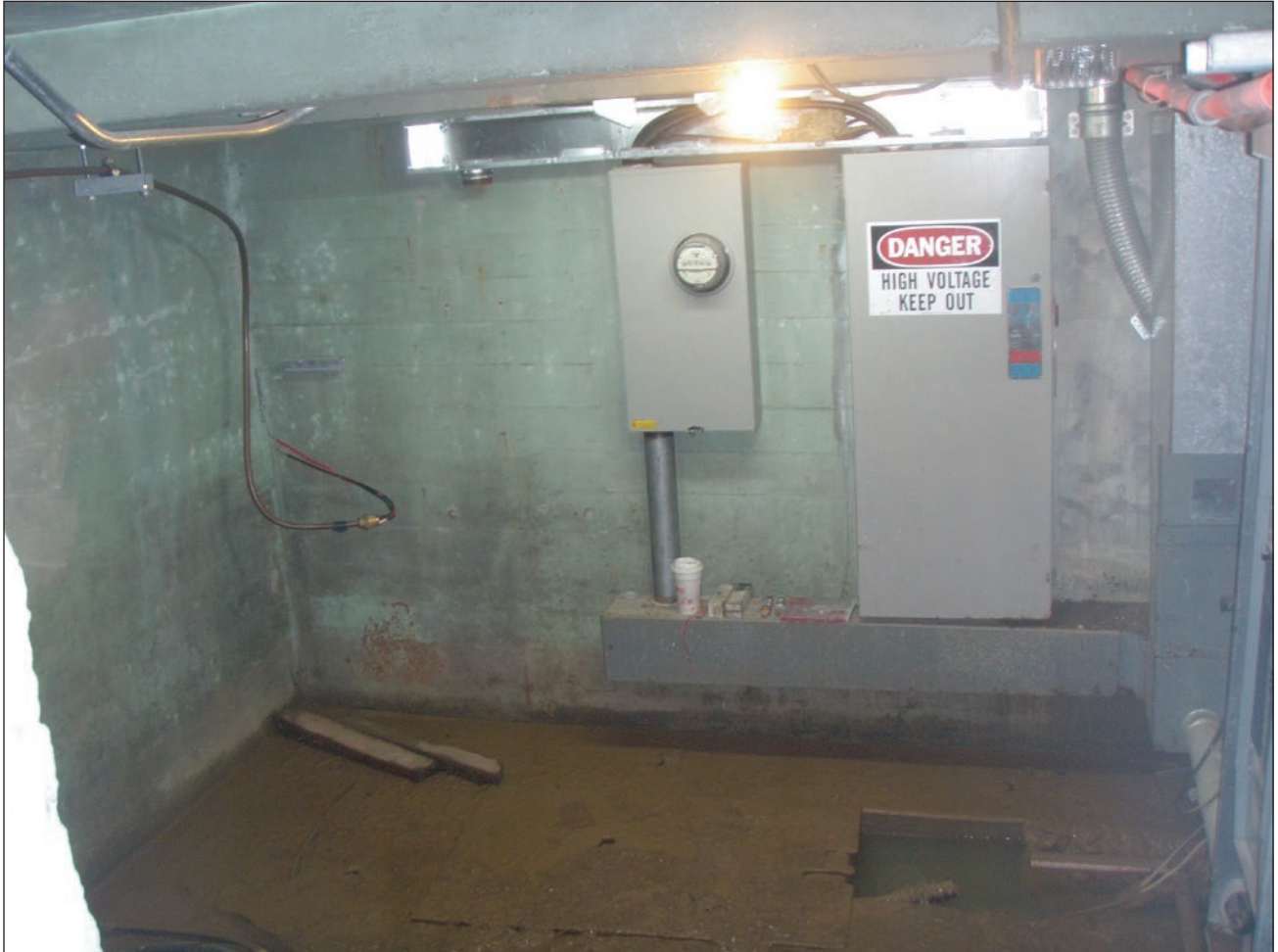
Figure 62. Basement of the 1921 comfort station. ARHO Archives.
