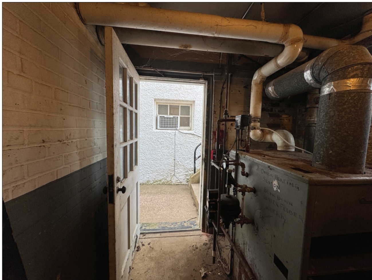
Figure 170. Southwest basement room. View looking south. Note the two-tone paint scheme on the brick wall. Building Conservation Associates, 2025.
