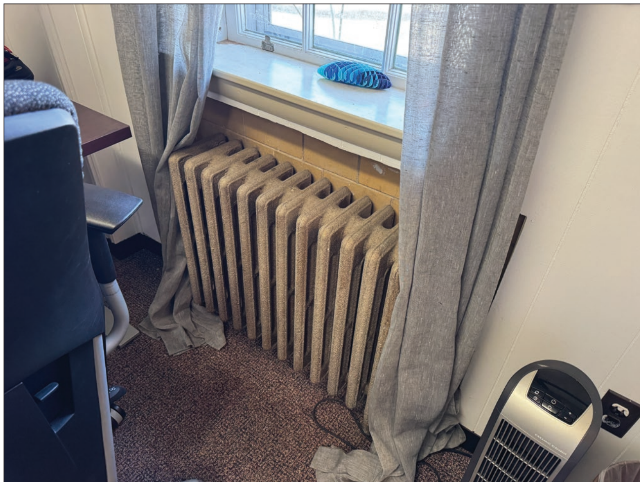
Figure 135. Radiator in first-floor south room, site of former white men's toilet room. Building Conservation Associates, 2025.
