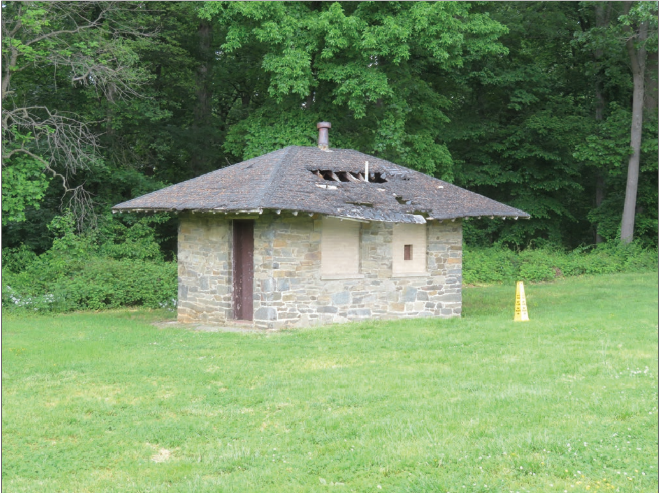
Figure 54. Comfort station at Picnic Grove 24 in Rock Creek Park, designed by NPS architect A.M. Jones and constructed between 1925 and 1926. Building Conservation Associates, Inc., 2021.
