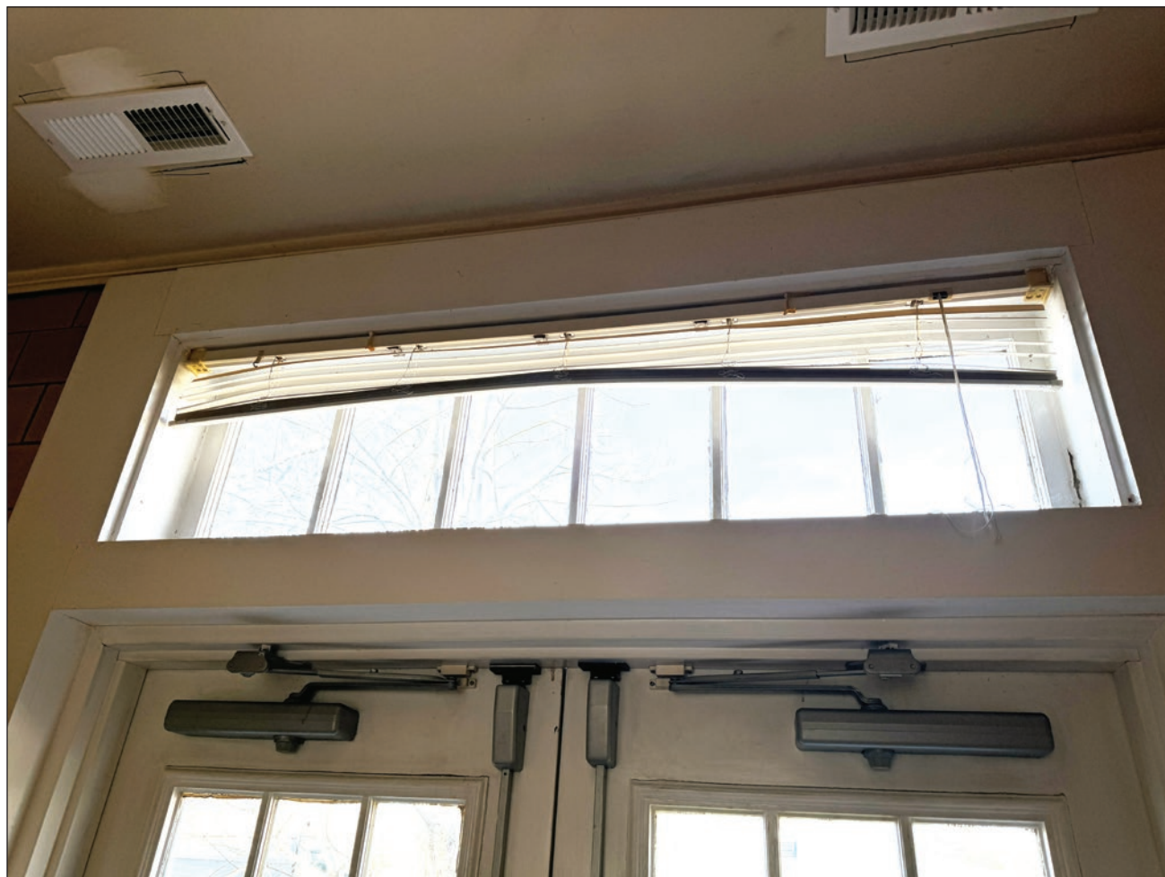
Figure 185. Transom above main (west) entrance door. Building Conservation Associates, 2025.
