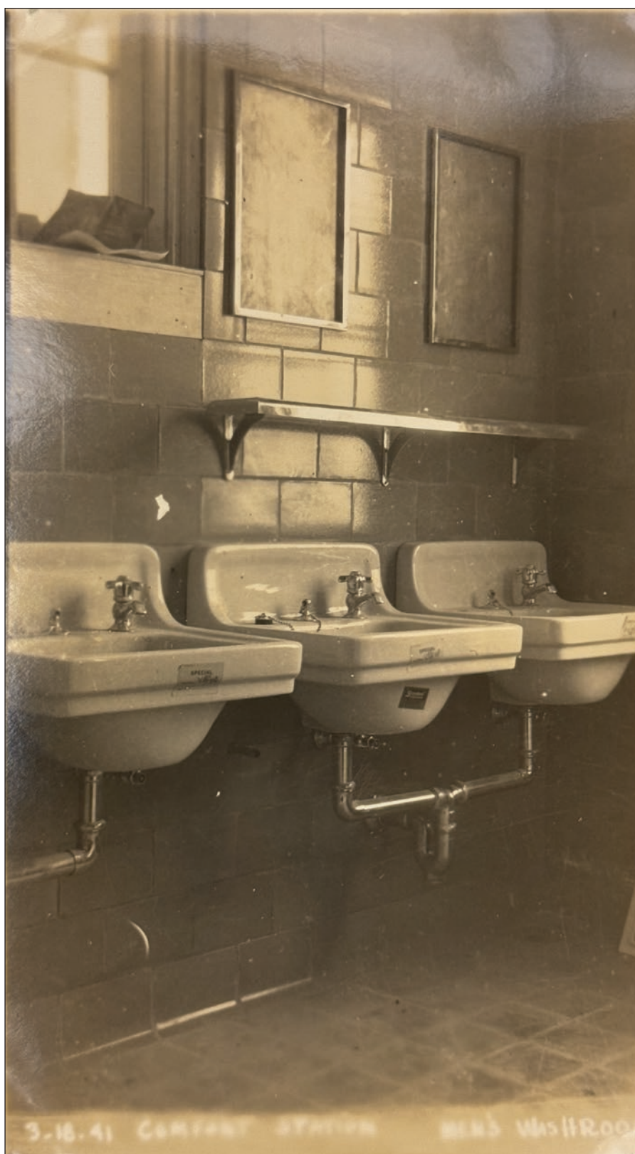
Figure 117. "Corner of Men's Toilet Room, showing tile walls, chromium plated shelves and mirrors," 1941. Nottingham, Completion Report, appendix.
