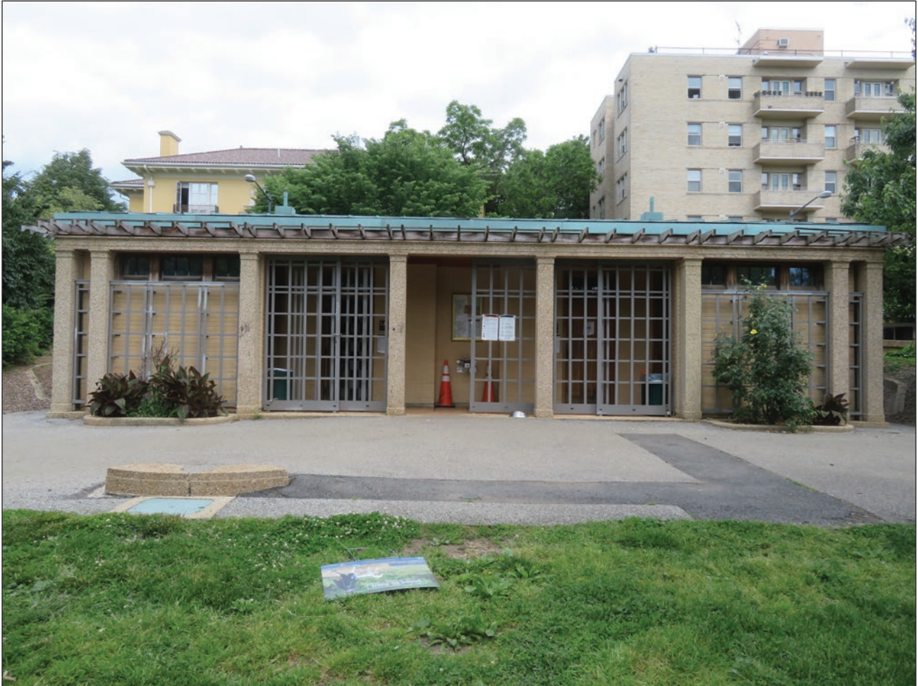
Figure 52. Lodge in Meridian Hill Park, designed by Horace Peaslee in 1917 and completed in 1924. Building Conservation Associates, Inc., 2021.
