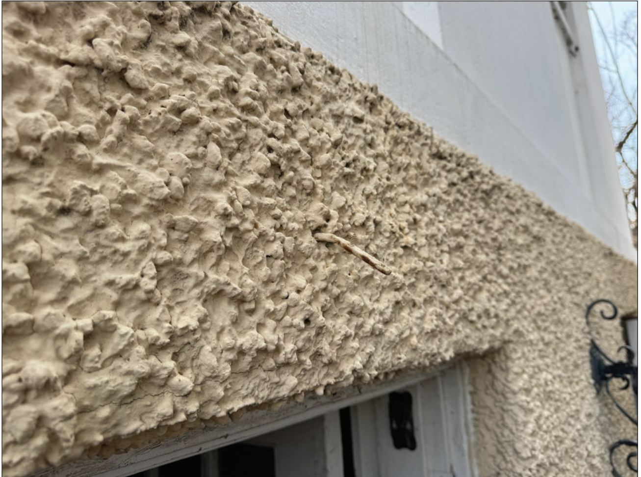
Figure 159. Small metal anchor for former segregation signage over south entrances. Building Conservation Associates, 2025.
