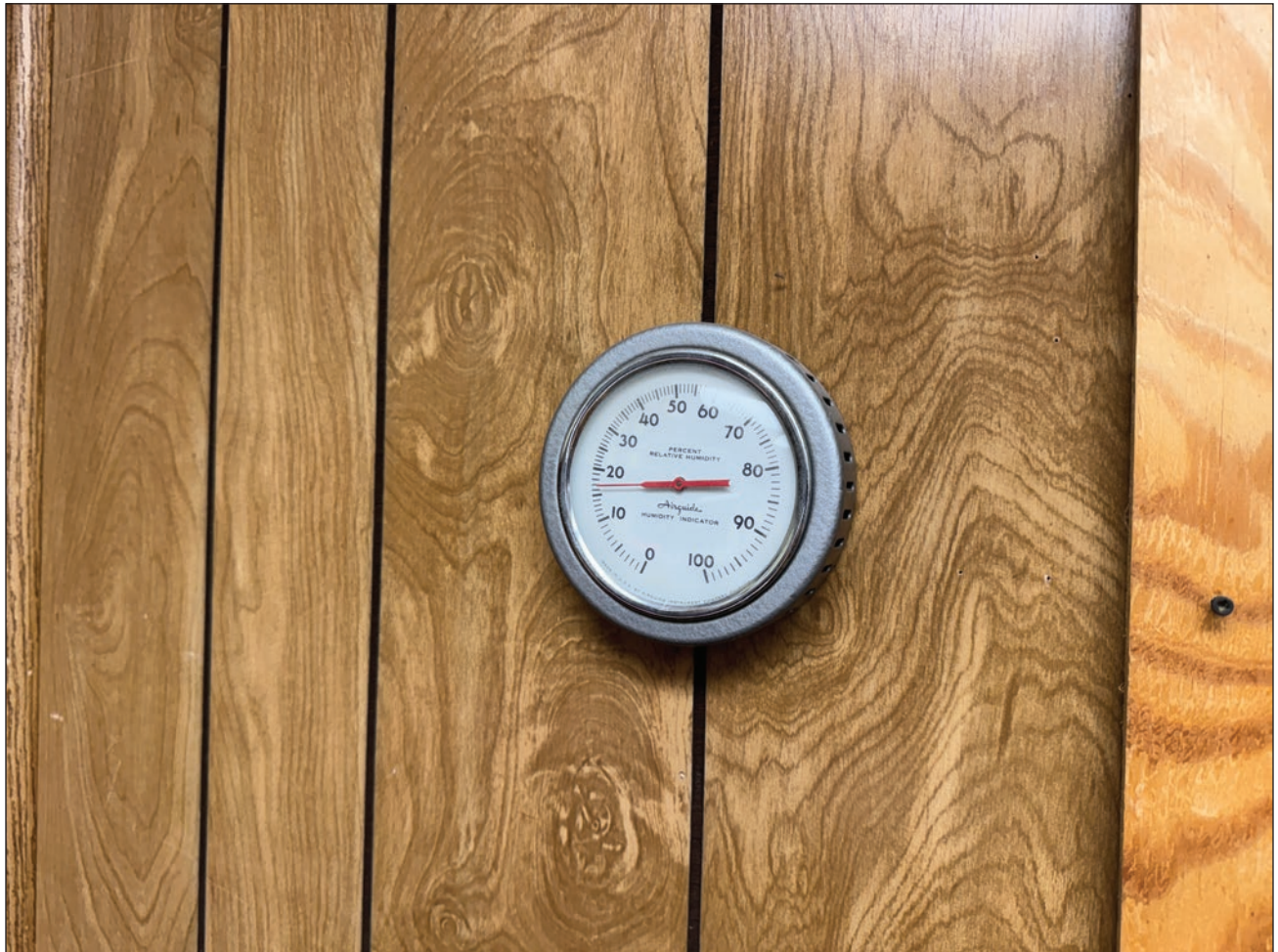
Figure 194. Airguide humidity indicator in east side of north room. Building Conservation Associates, 2025.
