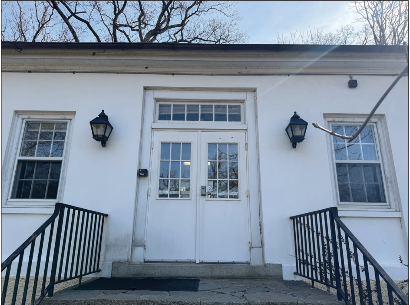
Figure 149. Double-hung windows flanking the main (west) entrance. Building Conservation Associates, 2025.
