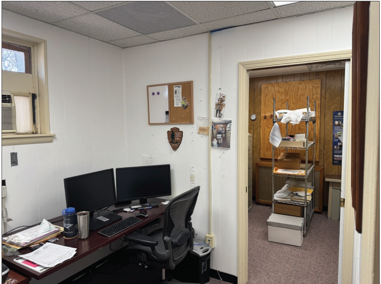
Figure 178. Partition wall added to divide the north room on the first floor into two spaces. View looking northeast. Building Conservation Associates, 2025.
