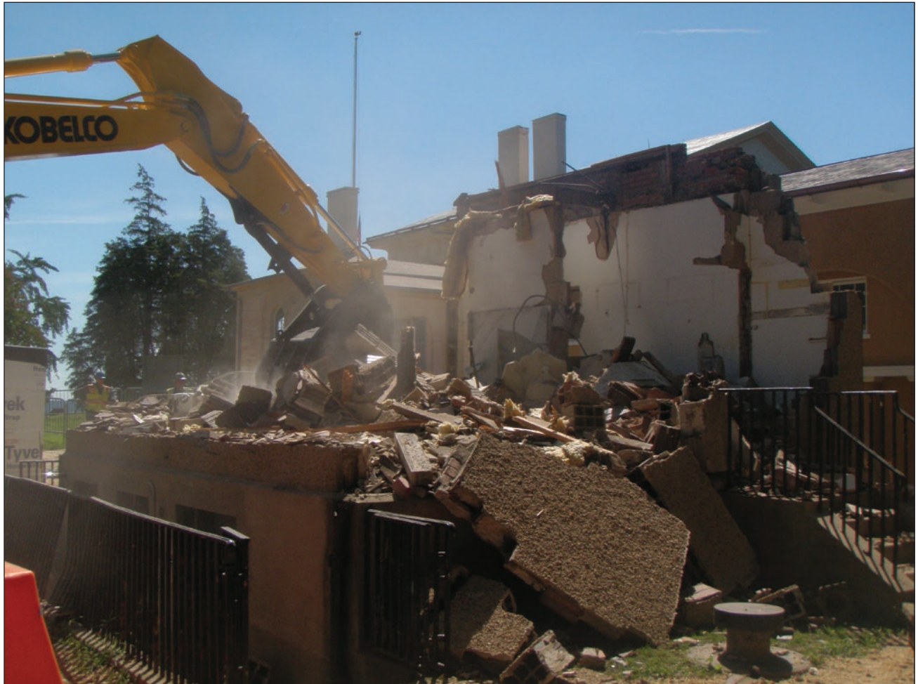
Figure 65. Demolition of the 1921 comfort station, 2009. ARHO Archives.
