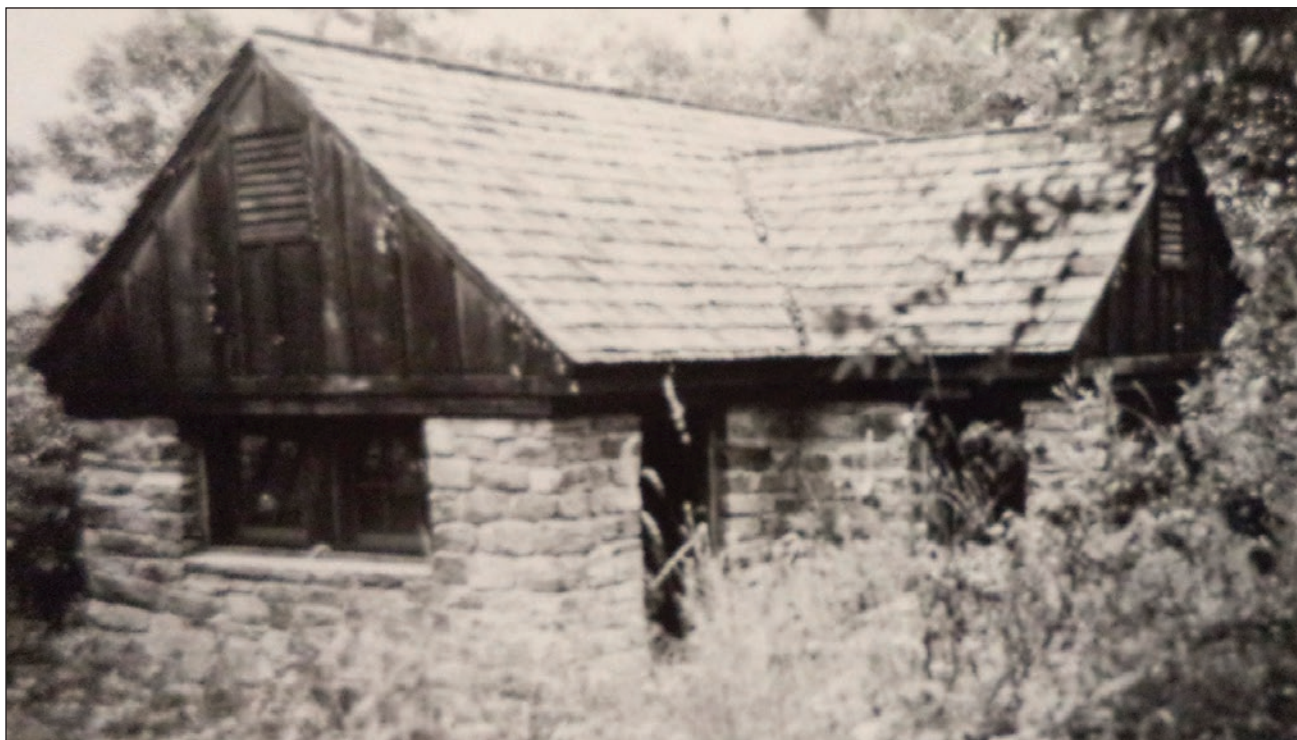
Figure 84. Photograph of the segregated Hughes River Gap comfort station using the standard layout from the drawing above. Building File, Box XI-8, Shenandoah Resource Management Records, Luray, VA.
