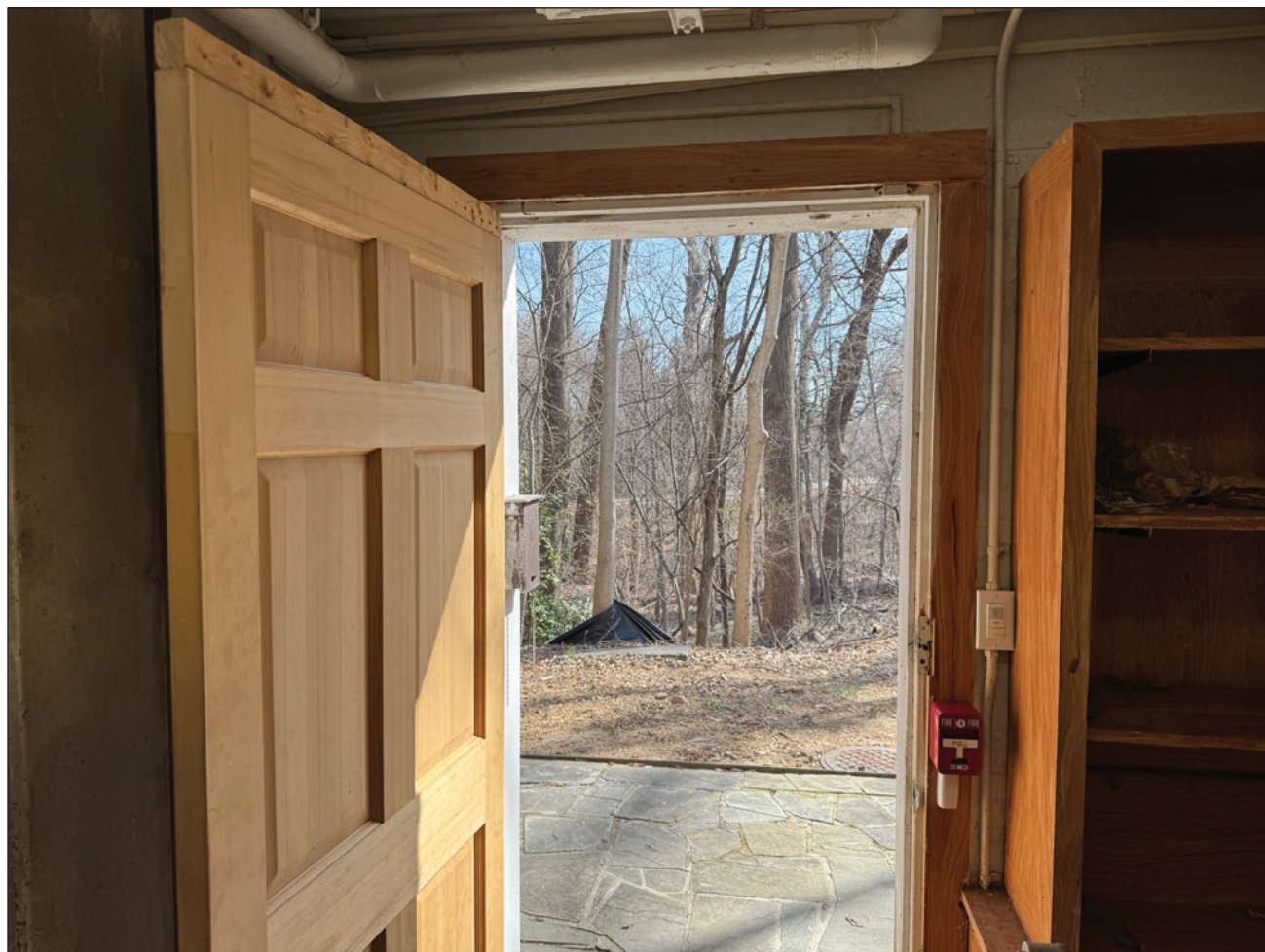
Figure 146. Unpainted wood door at center of east elevation. Also note the extra piece of wood to fit the new door to the existing frame. Building Conservation Associates, 2025.
