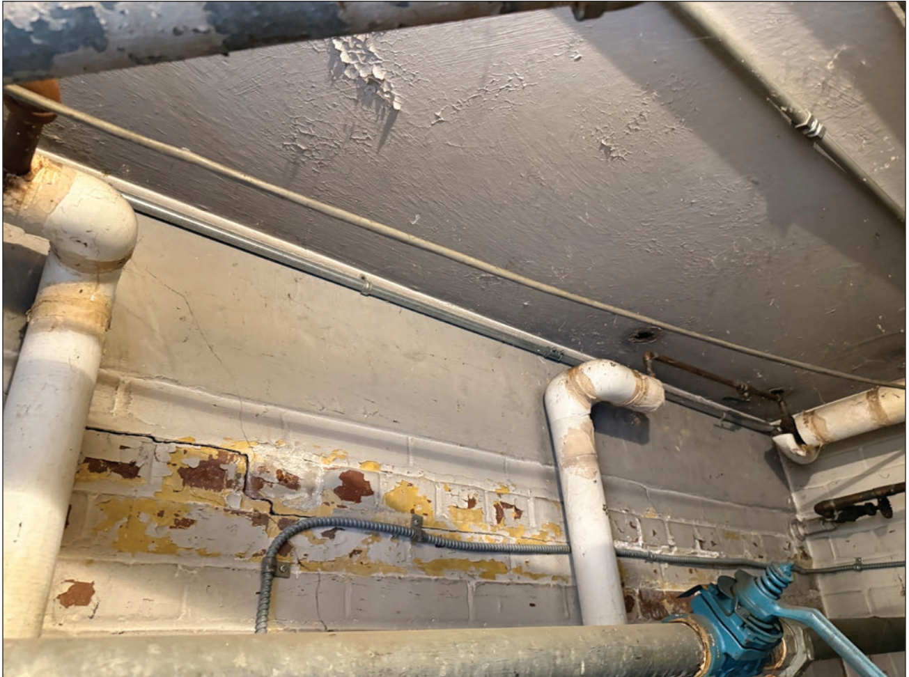
Figure 165. Painted concrete spandrel at the top of the west wall in the former segregated women's restroom. Building Conservation Associates, 2025.
