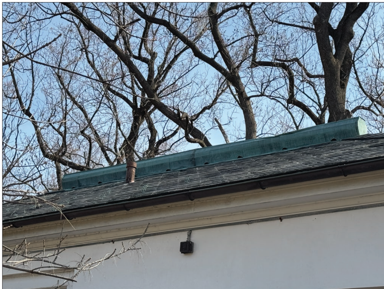
Figure 107. Copper ridge vent on center of roof. Building Conservation Associates, 2025.
