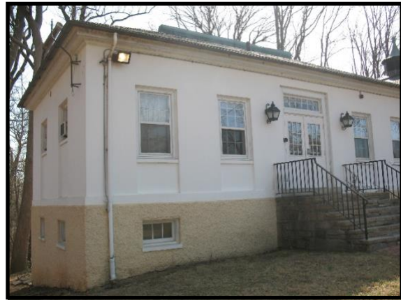
Photo P-2: Northwest building corner
