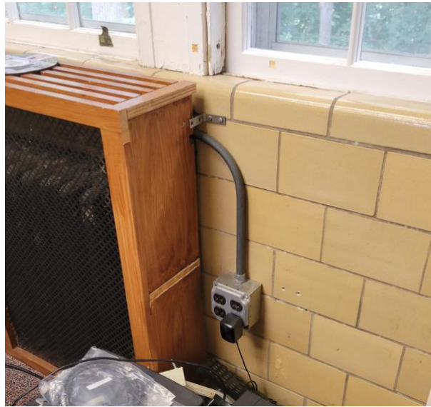
Photo E07: Surface-mounted receptacle installed on finished wall.
