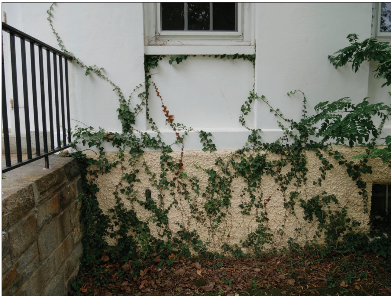
Figure 203. Scandent vines climbing the exterior pebble dash and flat stucco at the southwest corner. Building Conservation Associates, 2025.
