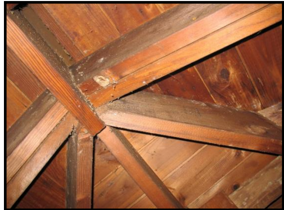
Photo P-8: South roof ridge beam and hip framing
