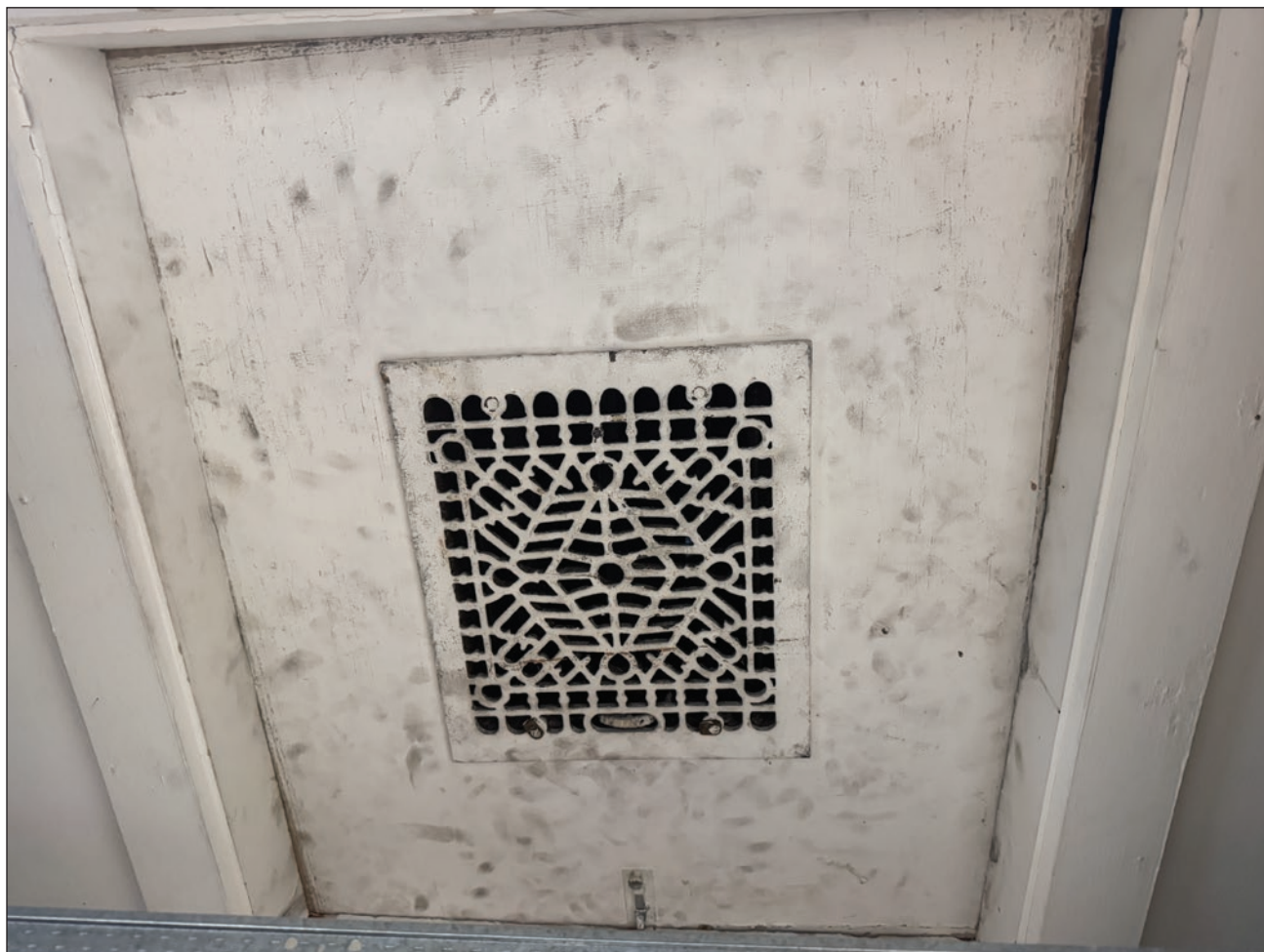
Figure 196. Attic scuttle door in south room. Building Conservation Associates, 2025.
