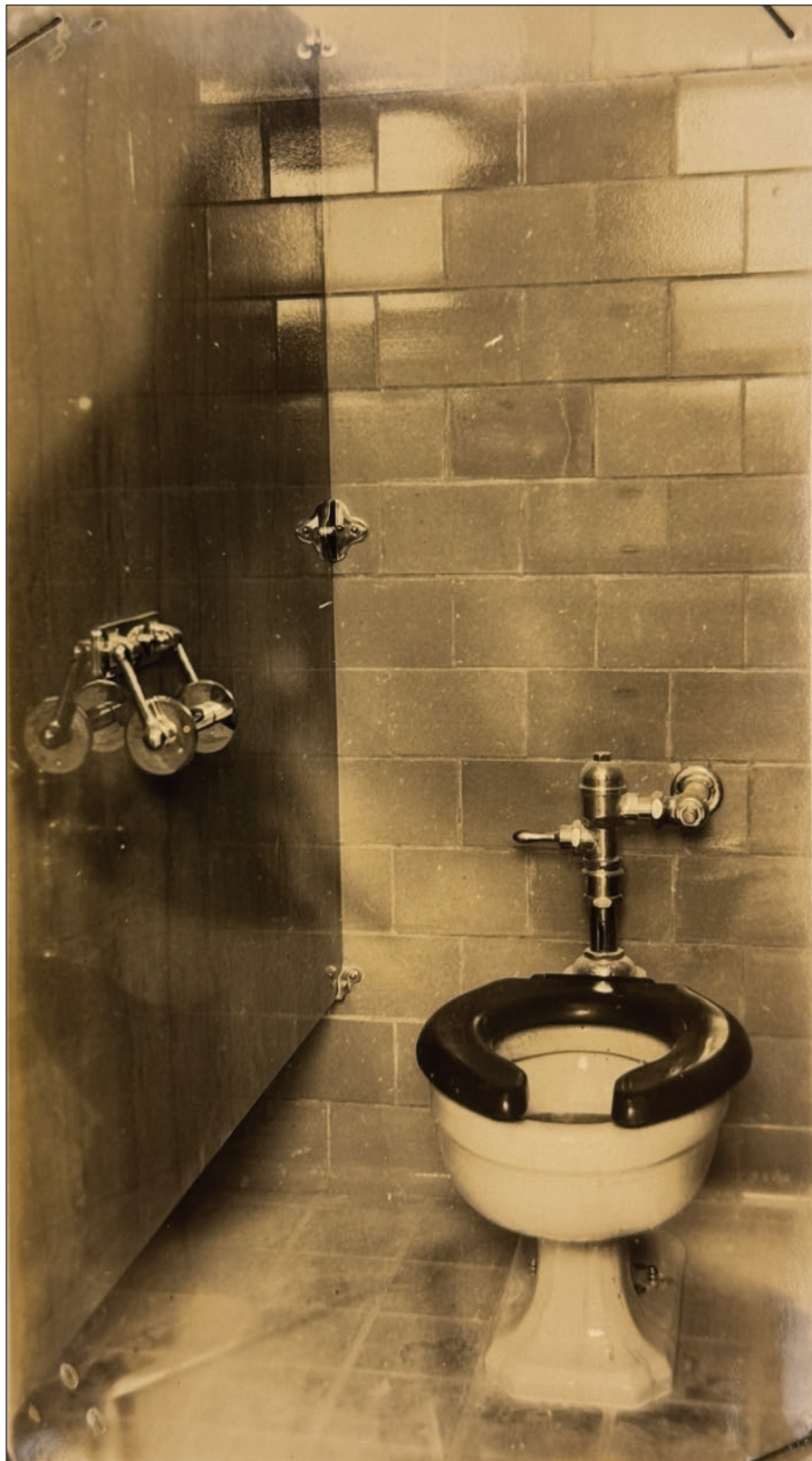
Figure 118. "Water closets tile walls and slate partitions," 1941. Nottingham, Completion Report, appendix.
