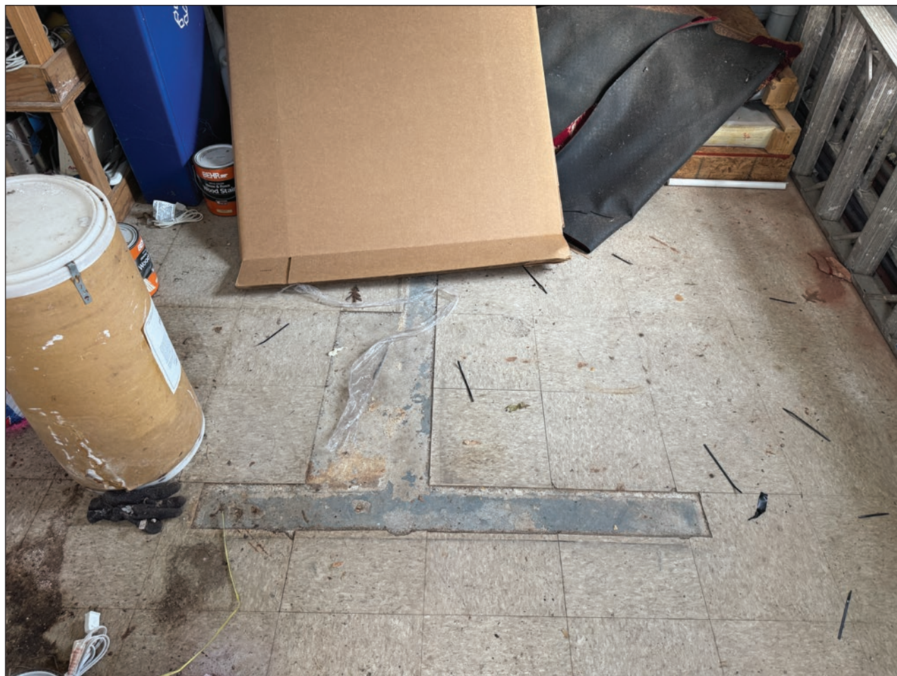
Figure 255. Vinyl floor tile in southeast basement room. Building Conservation Associates, 2025.
