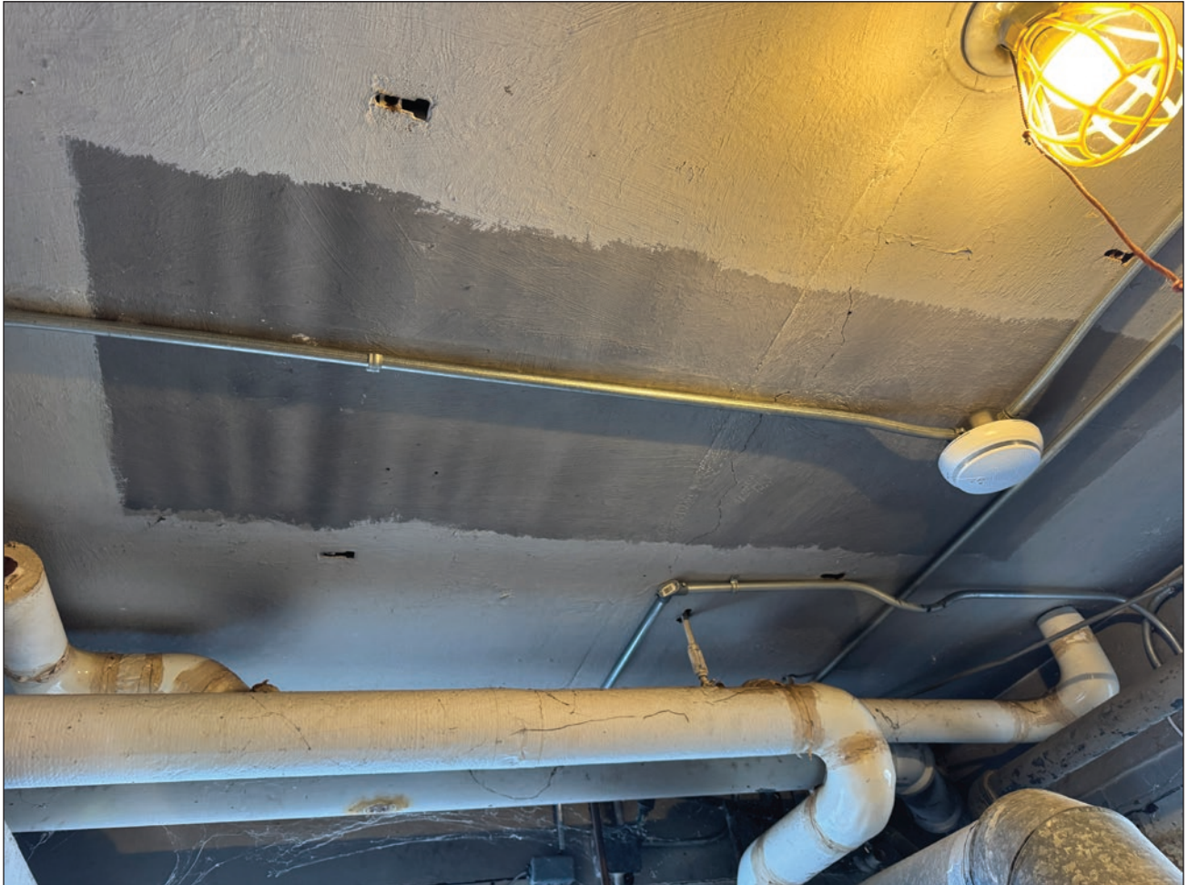
Figure 171. Location of the non-extant overhead radiator in the southeast basement room is marked with gray paint. Building Conservation Associates, 2025.
