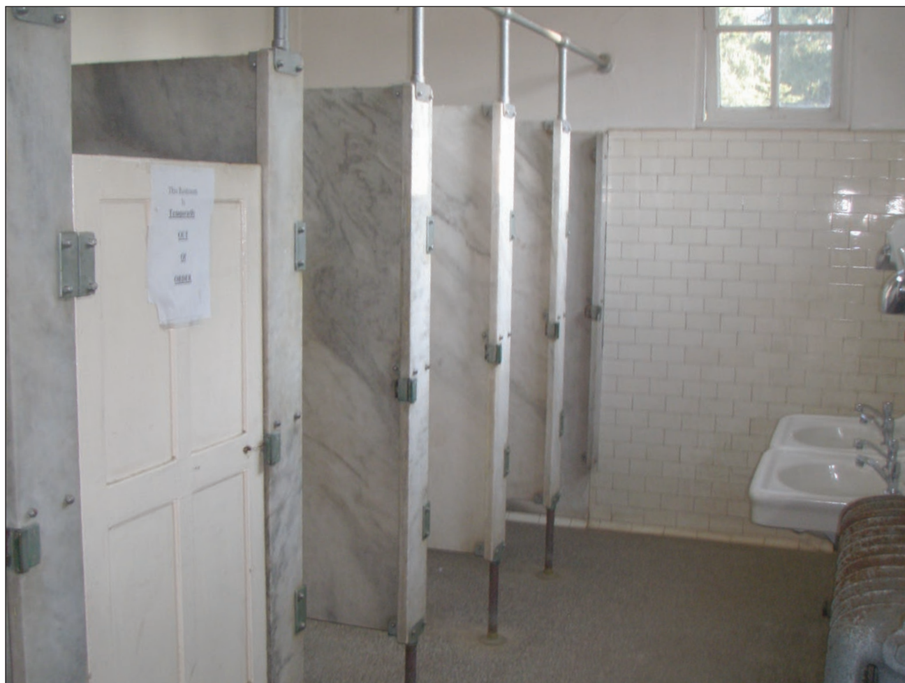
Figure 59. Women's toilet room in 1921 comfort station, 2009. ARHO Archives.
