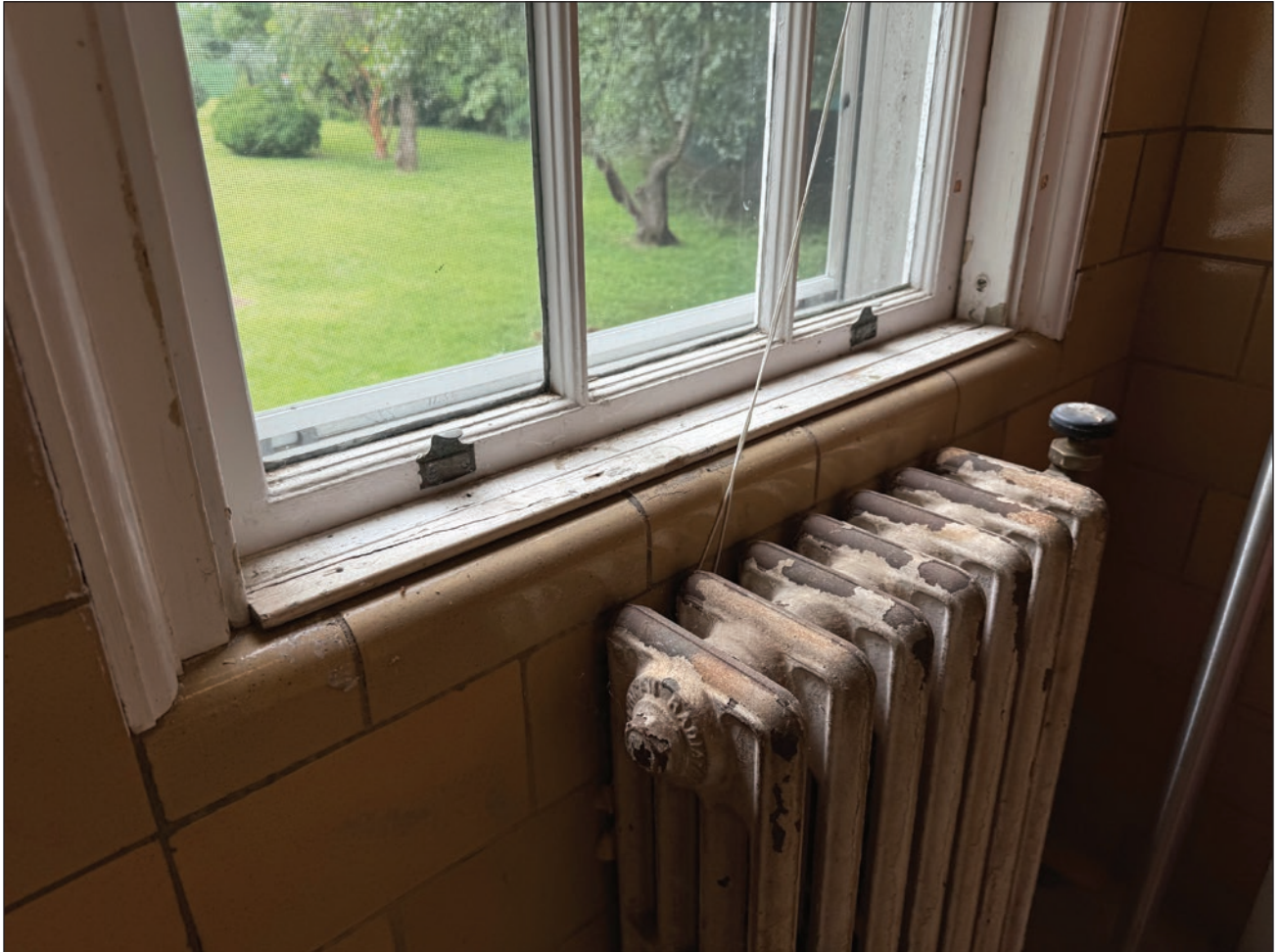
Figure 136. Radiator in first-floor vestibule. Building Conservation Associates, 2025.
