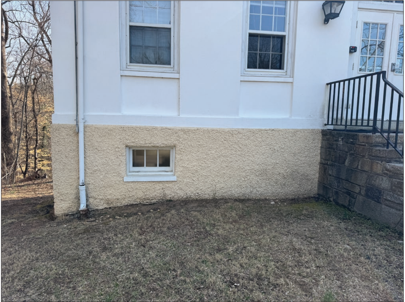
Figure 112. Building #313 west elevation showing exterior stucco finish with pebble dash at the lower register and smooth finish at the upper register and belt course. Building Conservation Associates, 2025.
