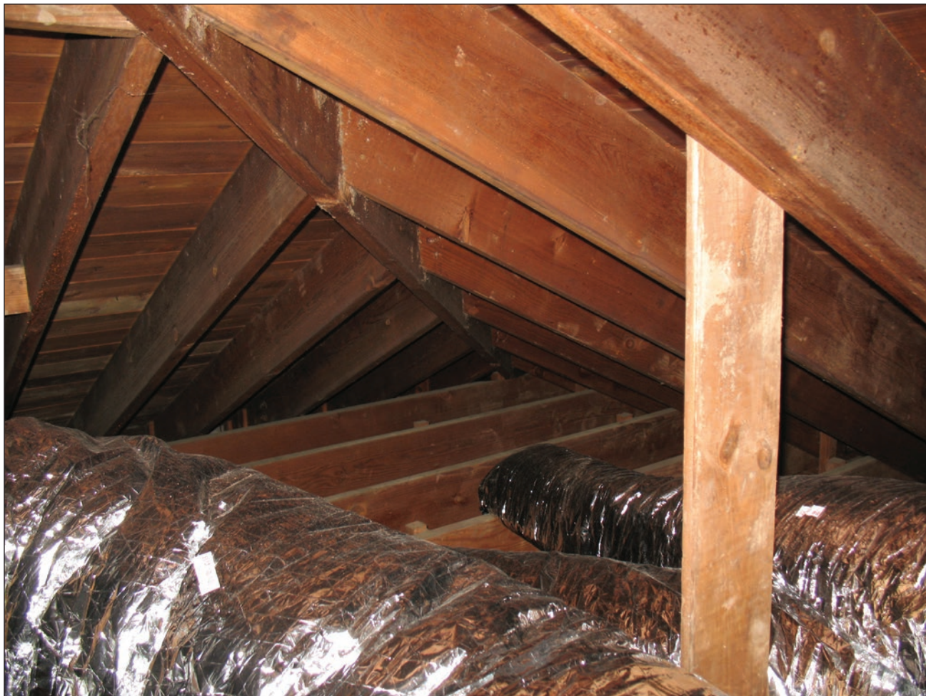
Figure 201. Exposed roof framing and ductwork in the attic. GWWO Architects, 2025.
