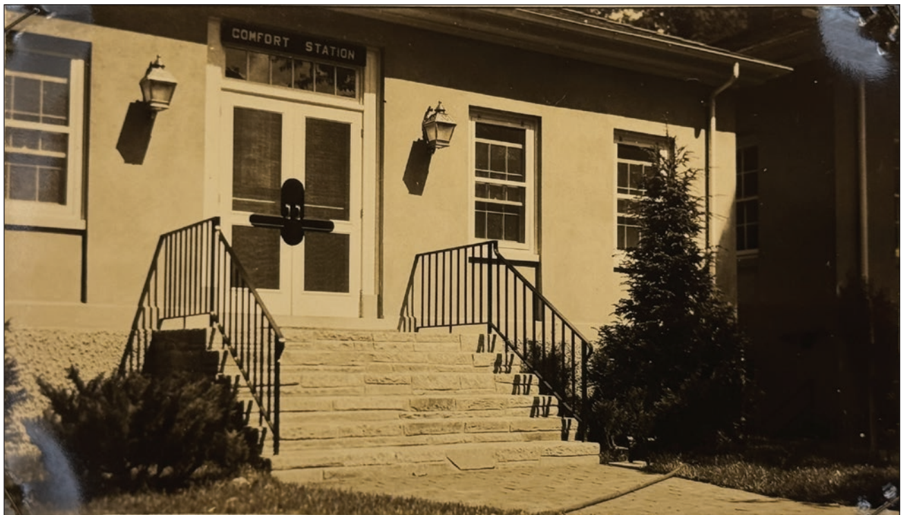
Figure 100. Building #313 main entrance, 1941. Nottingham, Completion Report, appendix.
