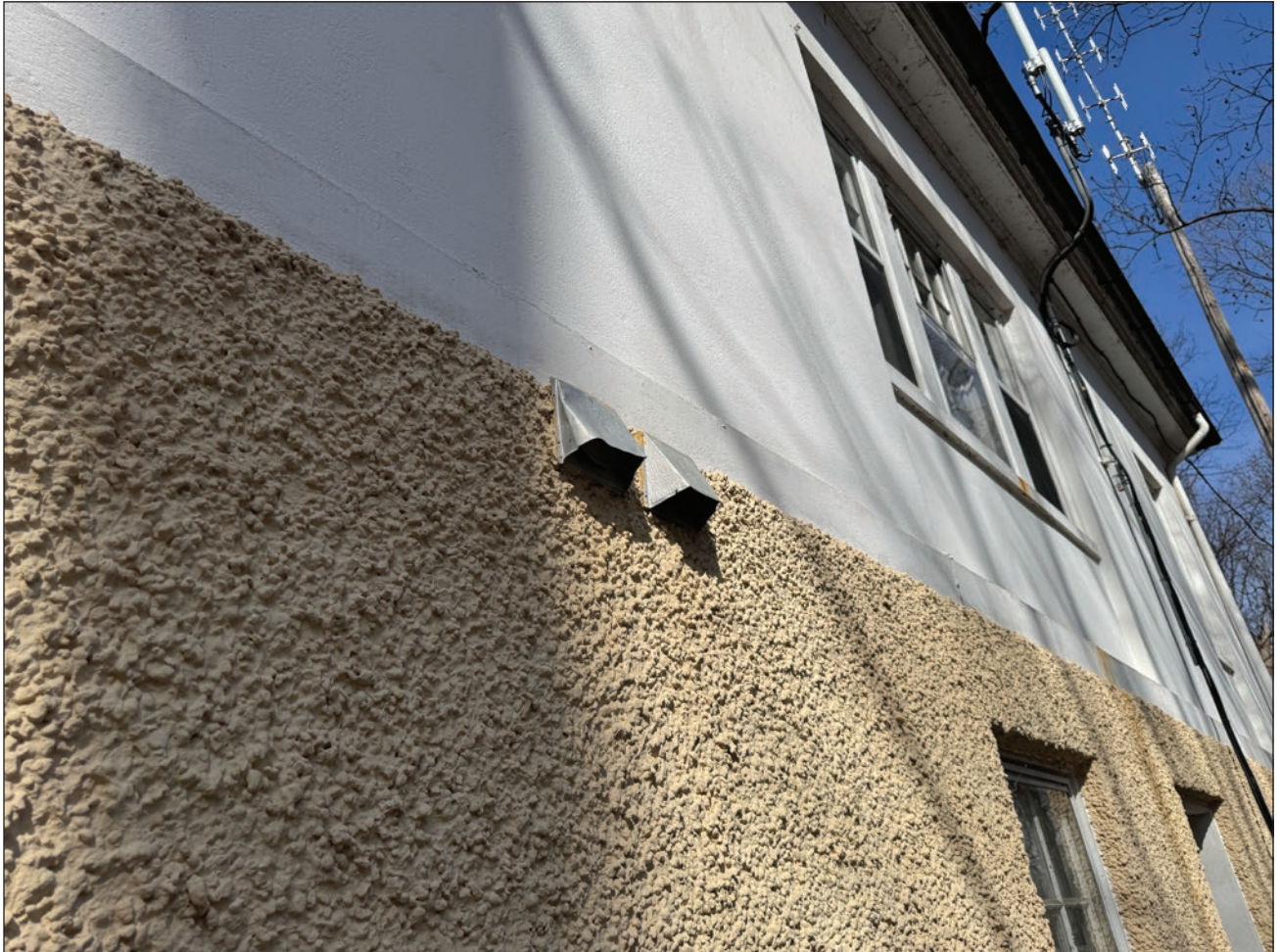
Figure 161. Small metal vents on east elevation. Building Conservation Associates, 2025.
