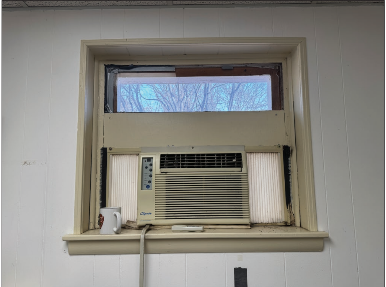
Figure 190. North window in north room. Building Conservation Associates, 2025.
