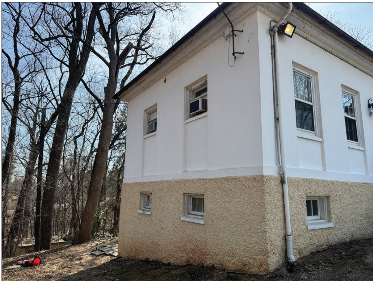
Figure 156. Northwest corner of Building #313. Building Conservation Associates, 2025.
