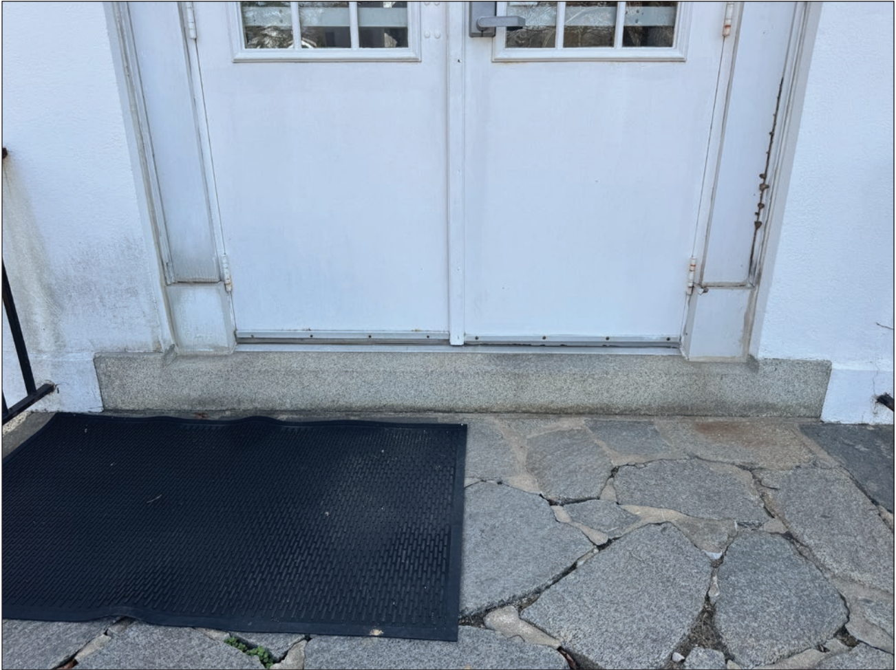
Figure 152. Rubble granite landing and carved granite sill at main (west) entrance. Also note the painted marble plinth blocks of the surround. Building Conservation Associates, 2025.
