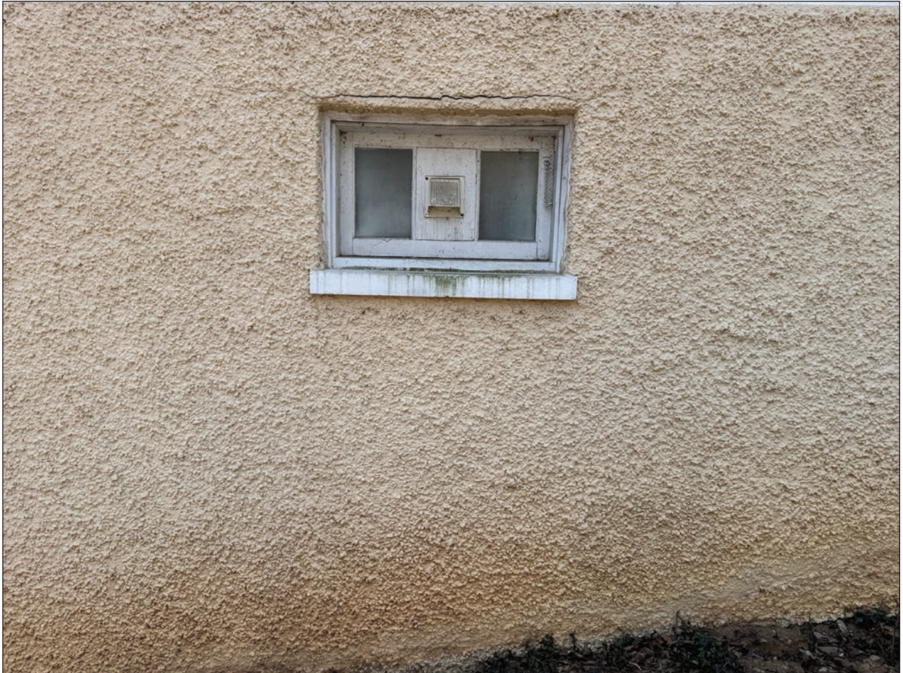
Figure 147. Modified basement window at the north elevation. Building Conservation Associates, 2025.
