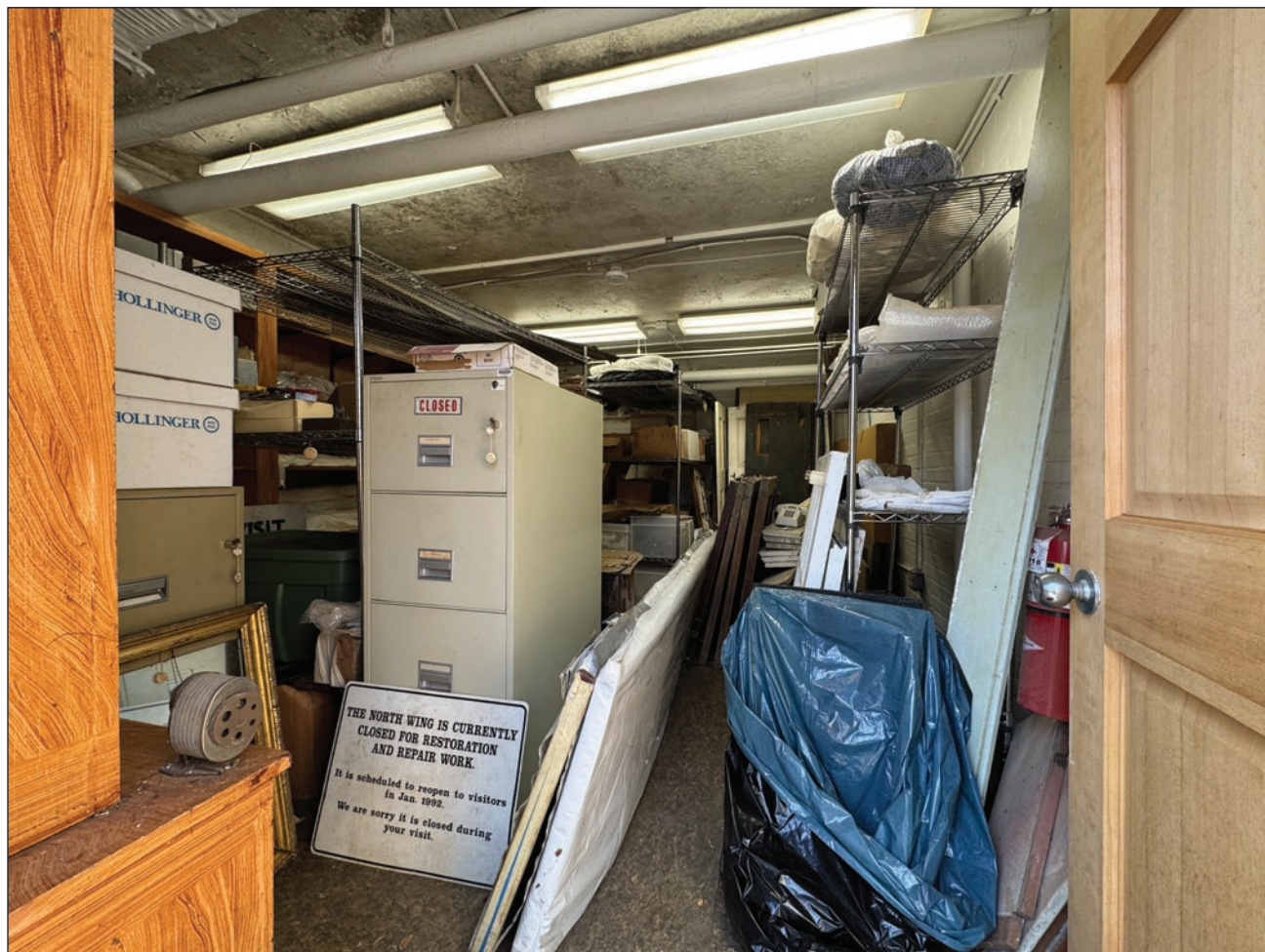
Figure 172. Center basement room. View looking west. Building Conservation Associates, 2025.
