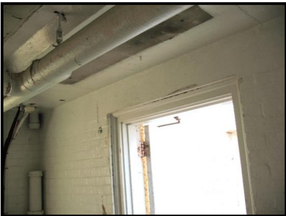
Photo P-13: First floor perimeter concrete beam and slab - southeast basement room
