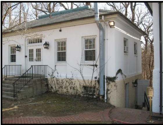
Photo P-1: Southwest building corner
