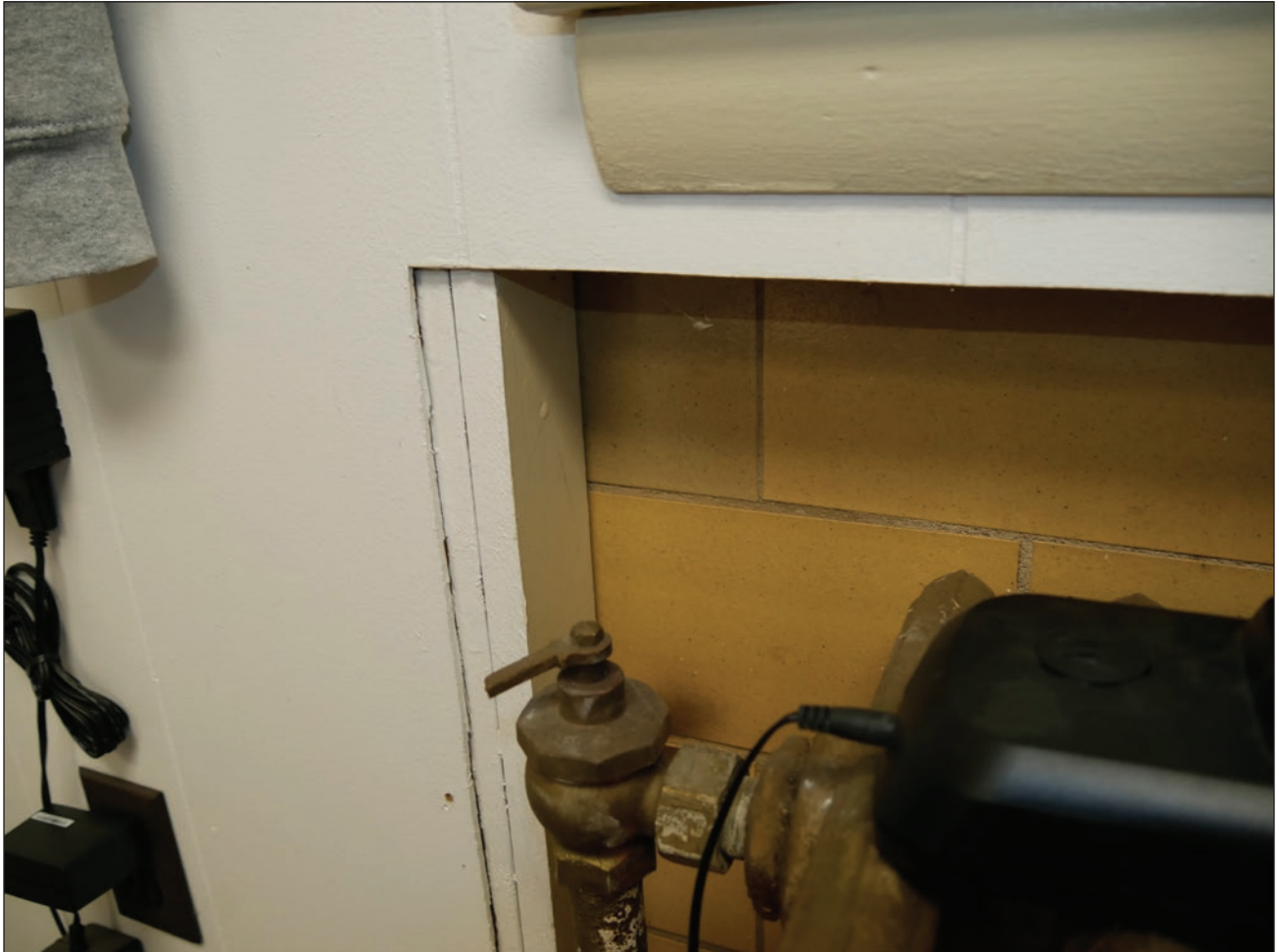
Figure 258. HDF paneling in north office. Building Conservation Associates, 2025.
