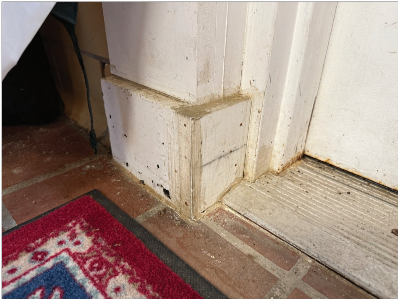
Figure 183. Painted marble plinth block at the main entrance door. Building Conservation Associates, 2025.
