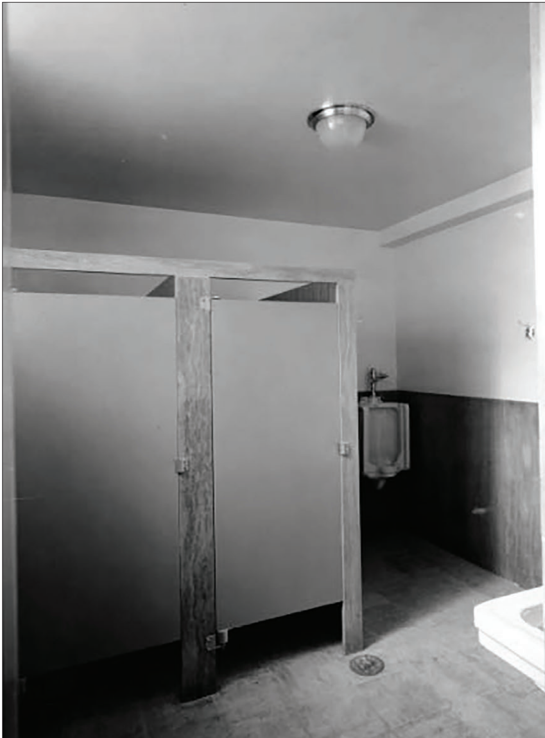
Figure 81. The interior of the white men's toilet room in the basement of the Administration Building at Fredericksburg and Spotsylvania National Military Park, 1936. "Men's Toilet: Administration Building," construction completion photograph, 14 April 1936, Chatham Manor Archives. Fredericksburg and Spotsylvania National Military Park, Fredericksburg, VA.
