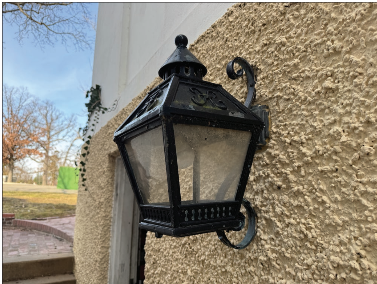
Figure 158. Detail of the lantern sconce on south elevation. Building Conservation Associates, 2025.
