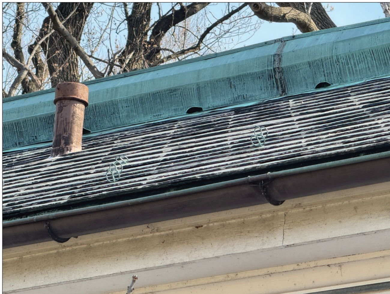
Figure 109. Copper gutter, copper wire snow guards, and cast-iron vent pipe. Building Conservation Associates, 2025.
