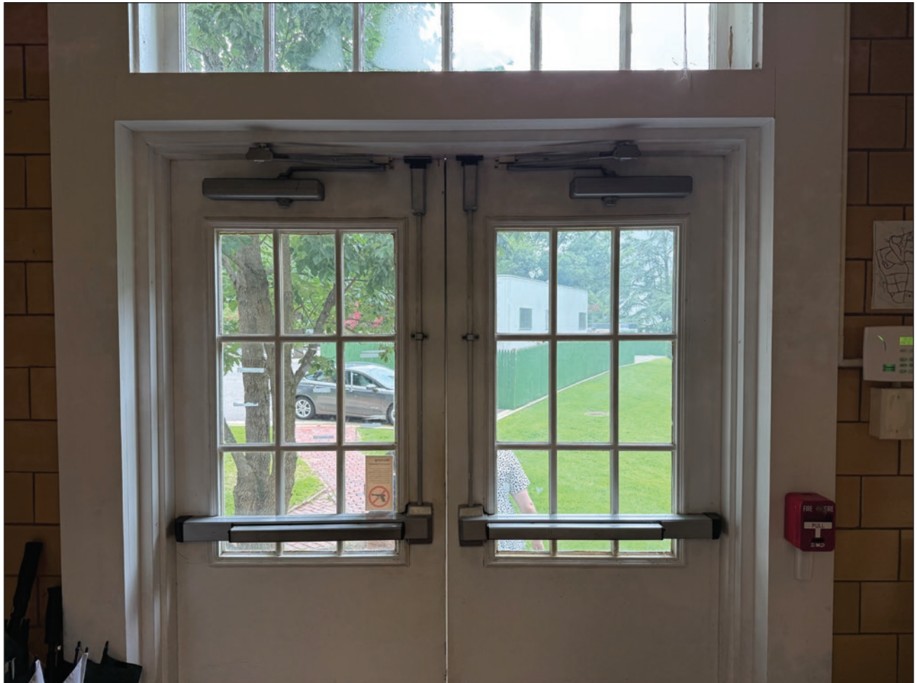
Figure 184. Main (west) entrance door. Building Conservation Associates, 2025.
