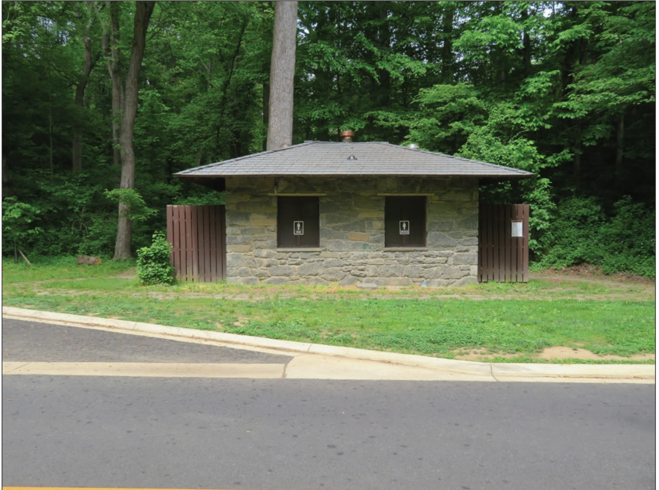
Figure 55. Comfort station at Picnic Grove 6 in Rock Creek Park, constructed in 1930. Building Conservation Associates, Inc., 2021.
