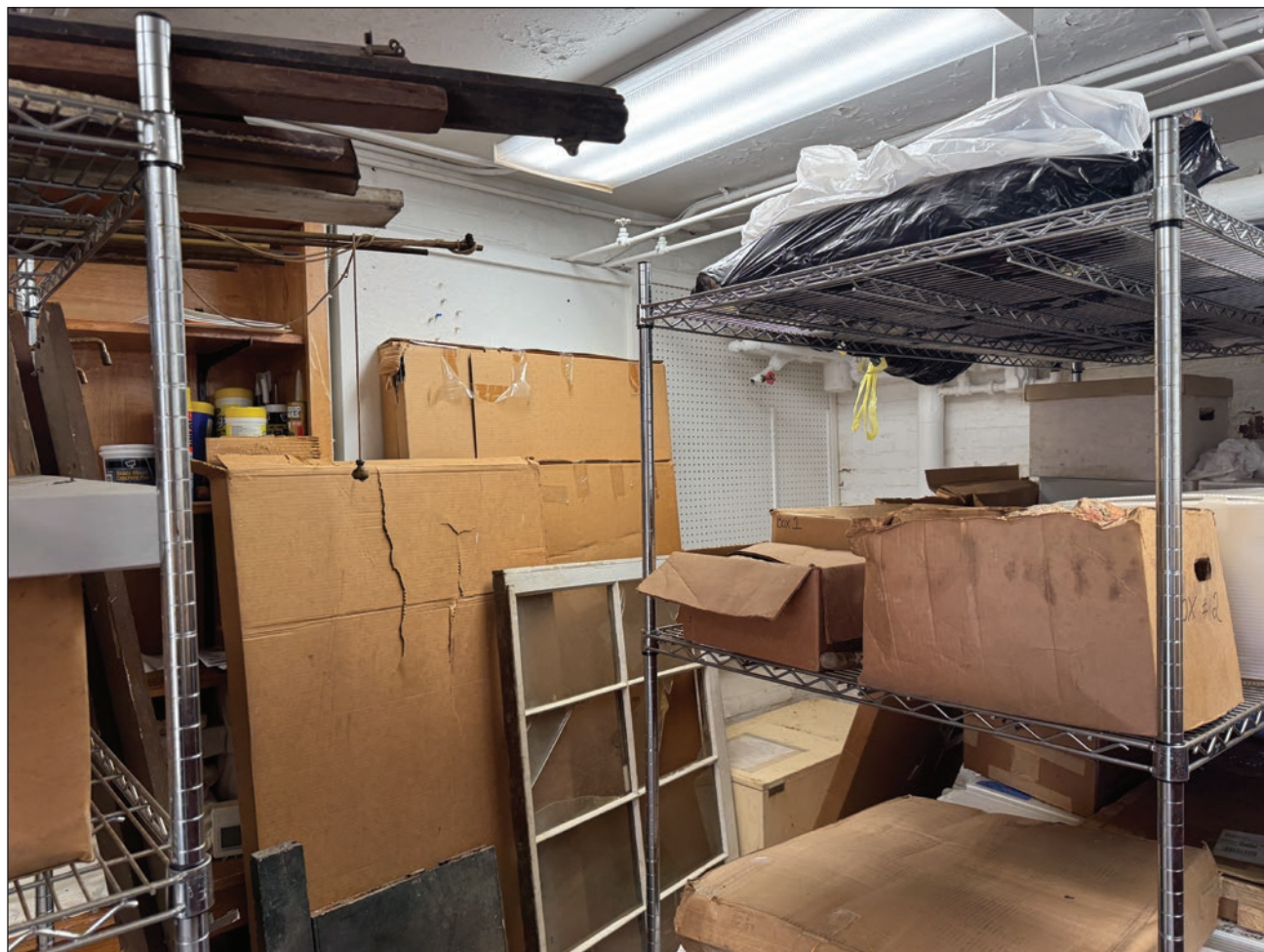
Figure 166. Former opening between the segregated women's restroom and toilet room blocked with peg board. View lookout southwest. Building Conservation Associates, 2025.
