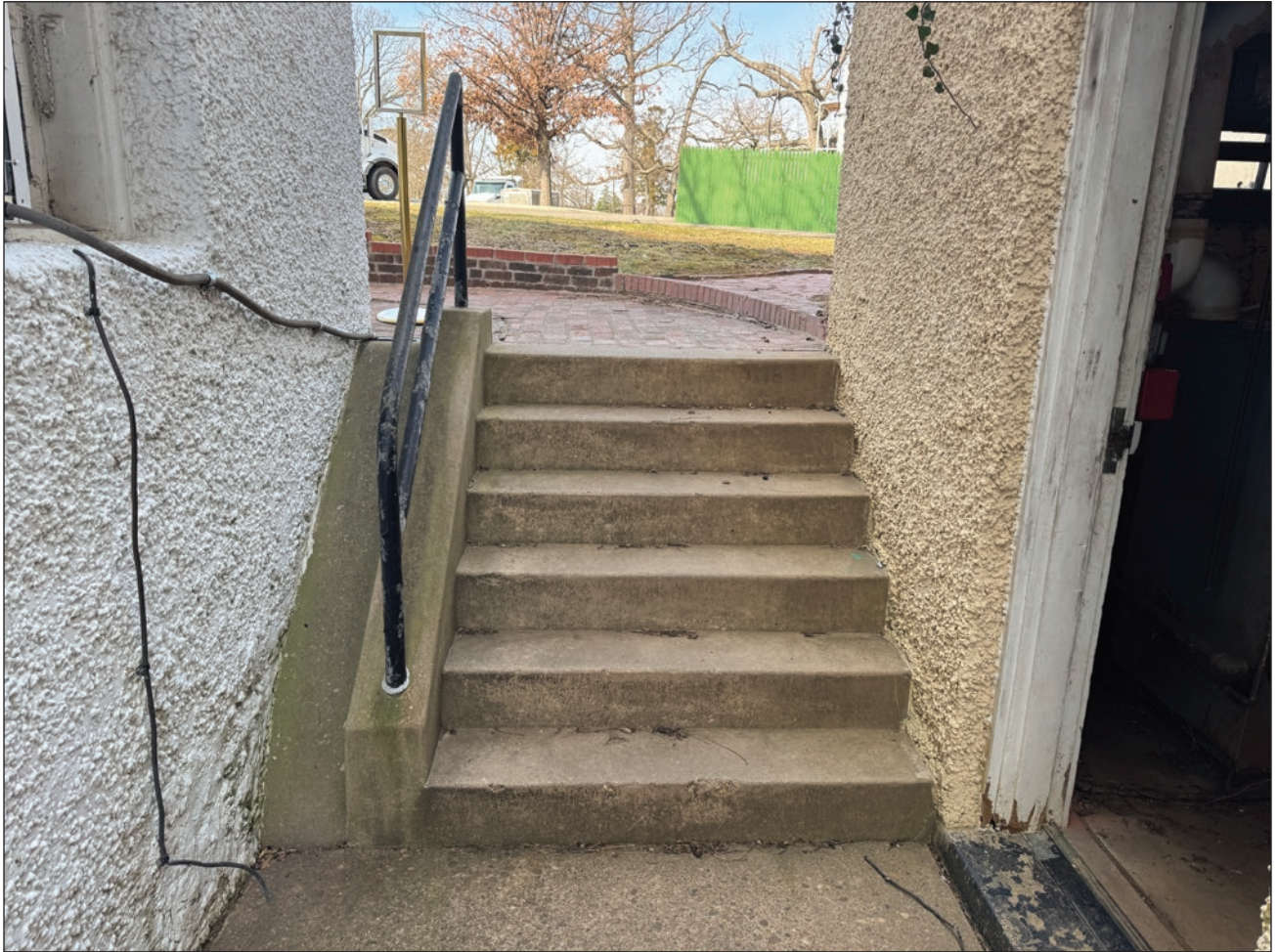
Figure 114. Concrete stairs with metal pipe railing leading to the alley on the south side of Building #313. Building Conservation Associates, 2025.
