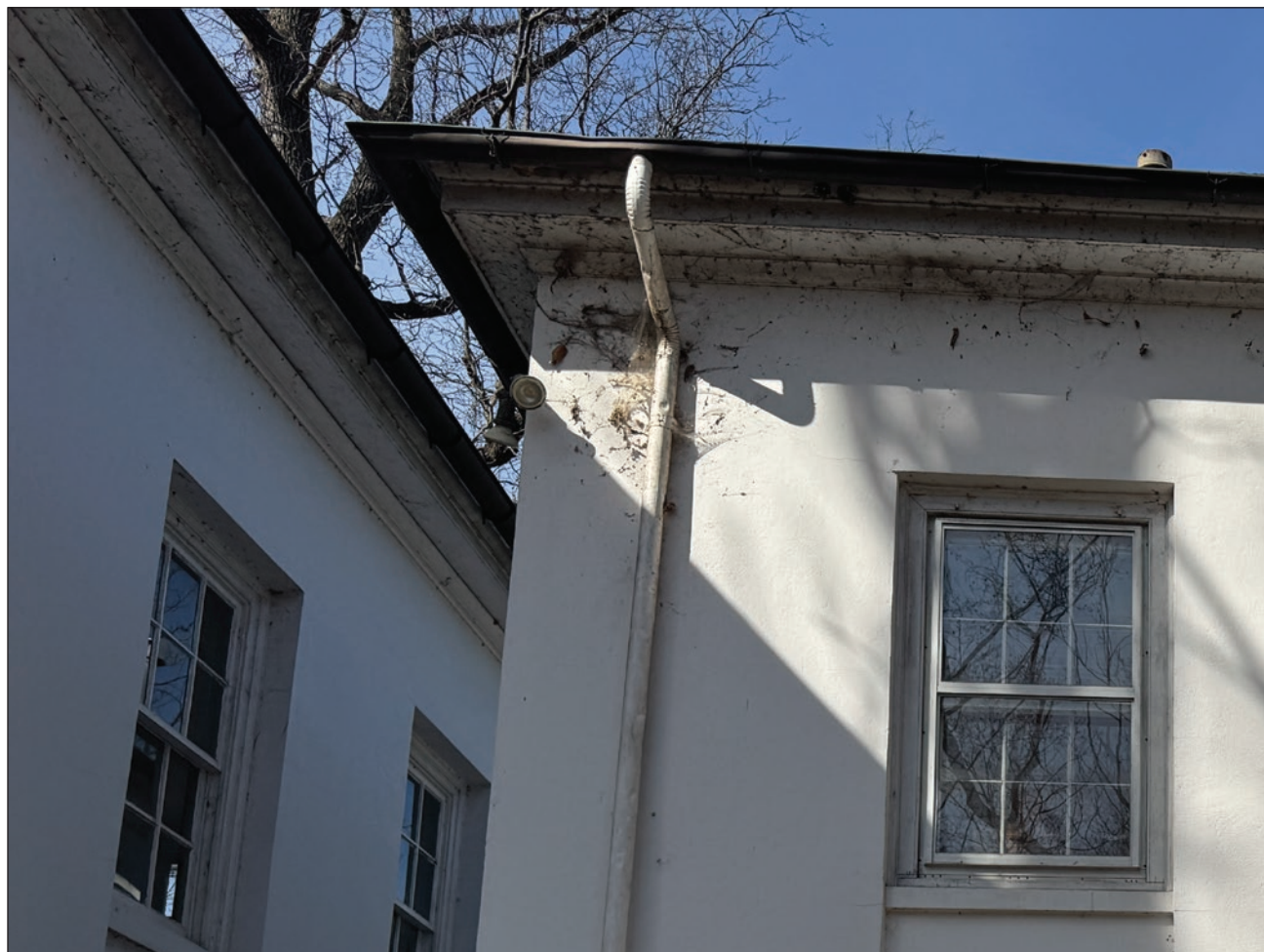
Figure 160. Small light fixture in upper southeast corner. Building Conservation Associates, 2025.
