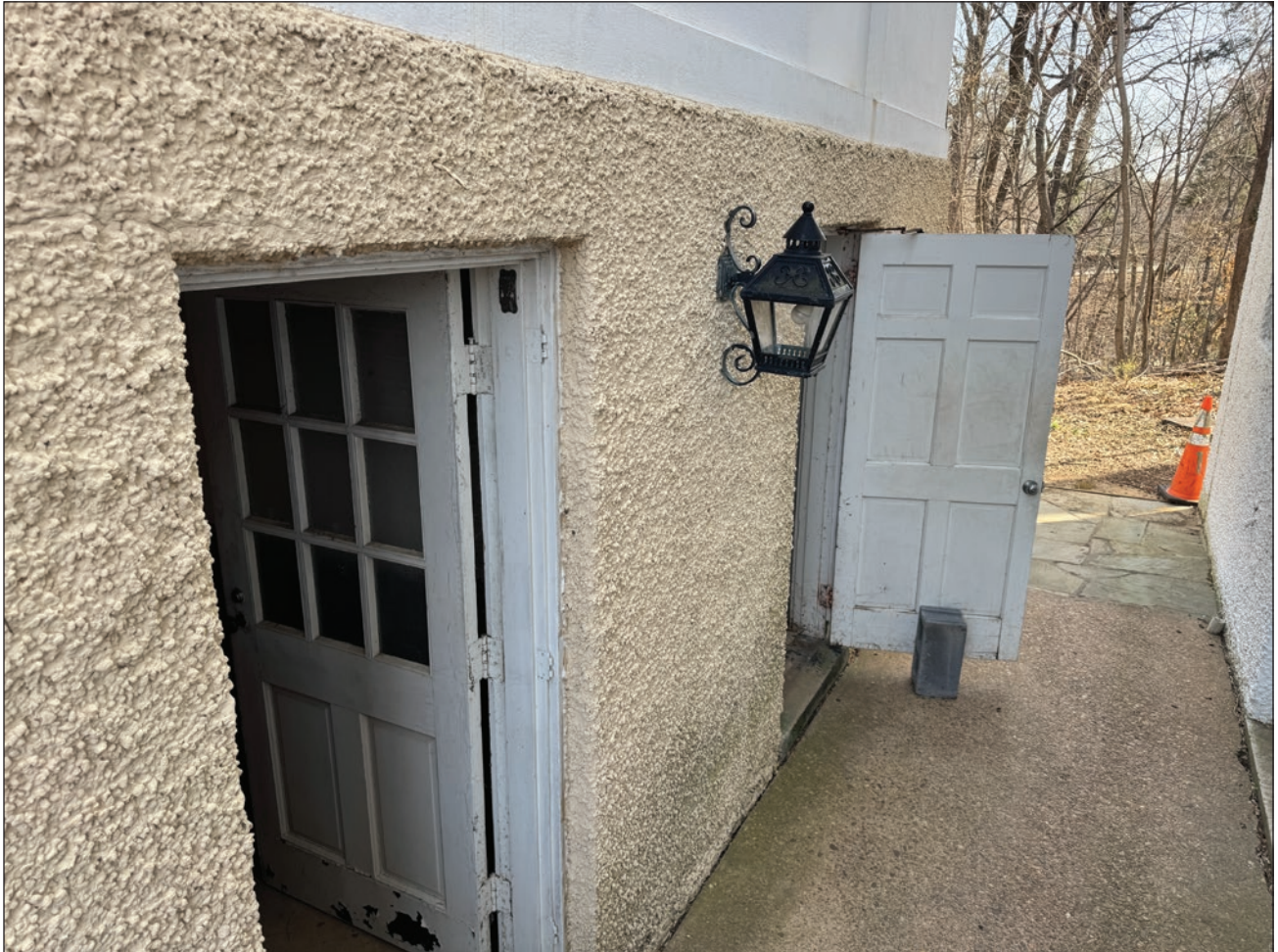
Figure 145. Entrances to the former segregated public toilet facilities in Building #313. Building Conservation Associates, 2025.
