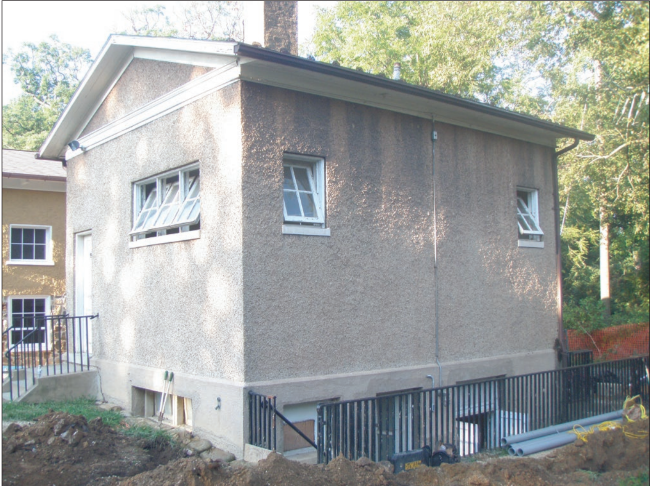
Figure 58. 1921 comfort station on grounds of Arlington House, 2009. View looking southwest. ARHO Archives.
