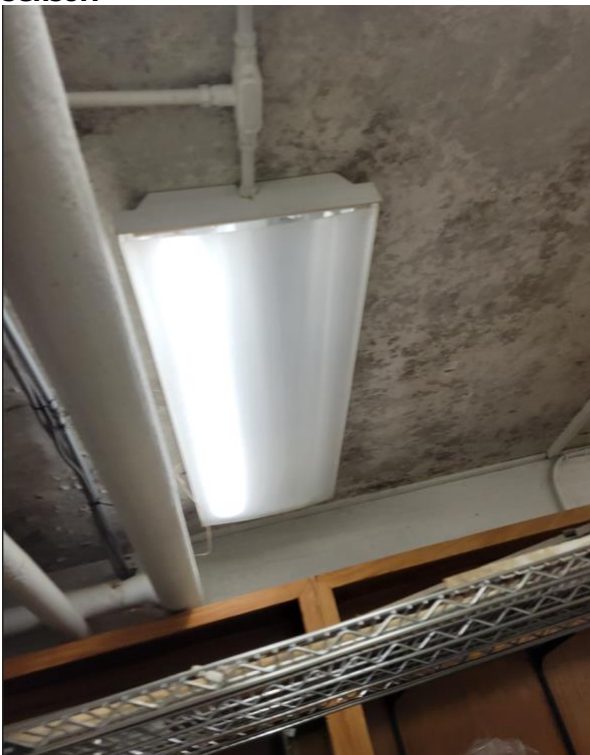
Photo E15: Storage area ceiling with rows of 1x4 fluorescent fixtures.
