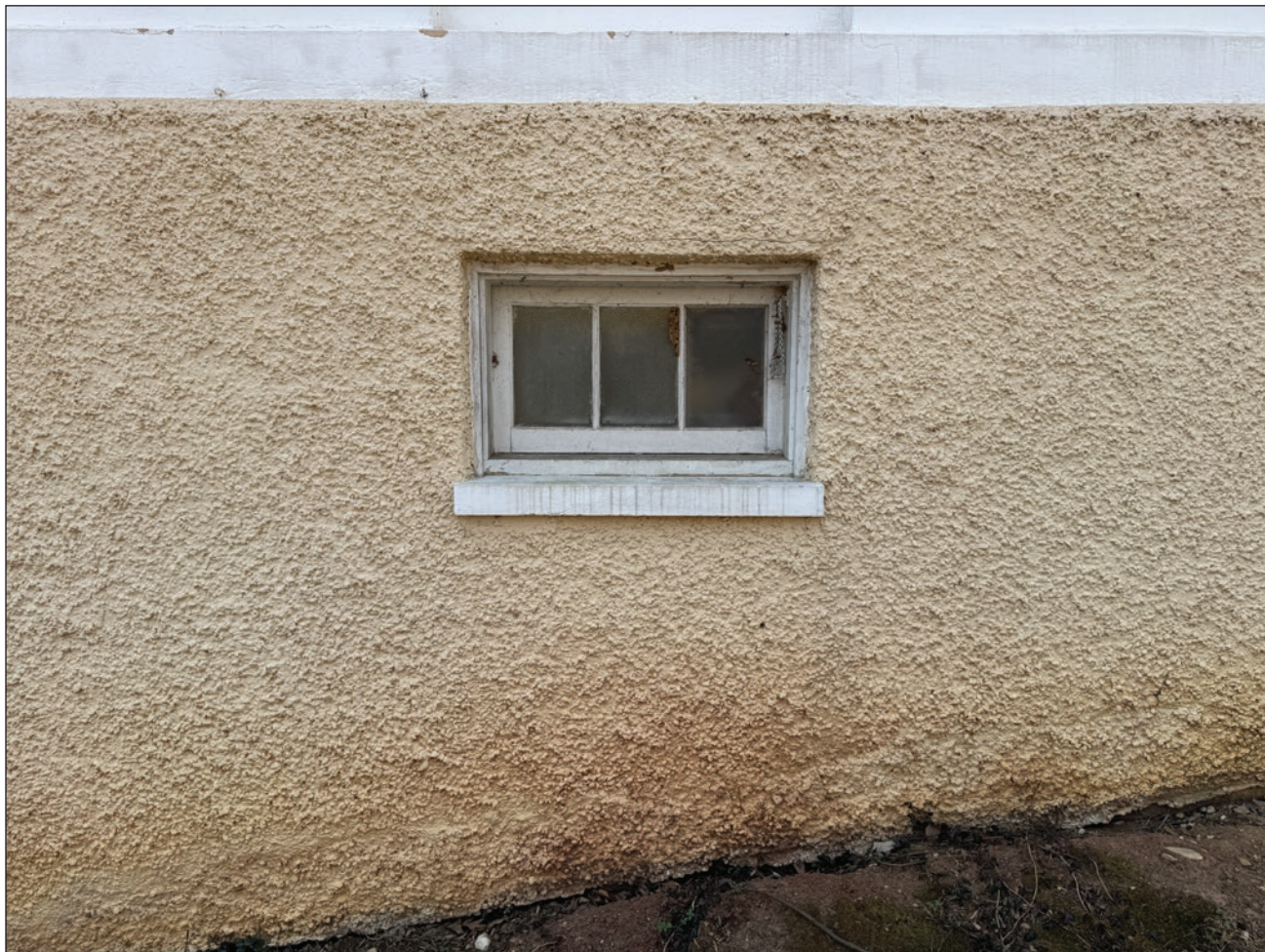
Figure 121. Basement window at north elevation. Building Conservation Associates, 2025.
