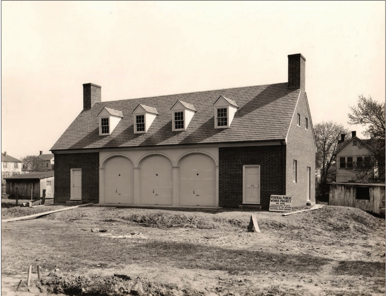
Figure 79. Service center at Fredericksburg and Spotsylvania National Military Park, 1936, showing entrances to segregated public toilet facilities. Courtesy of National Park Service, Fredericksburg and Spotsylvania NMP.
