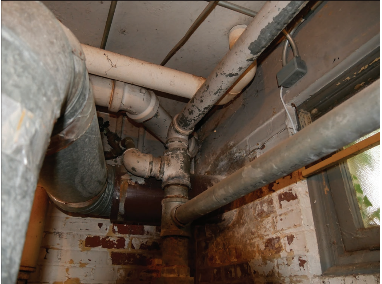
Figure 254. Cement patching at brick wall penetration in southwest basement room. Building Conservation Associates, 2025.
