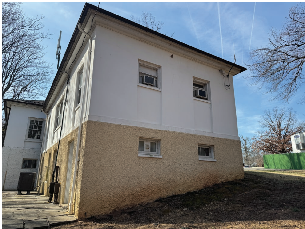
Figure 105. Building #313 north elevation. Building Conservation Associates, 2025.
