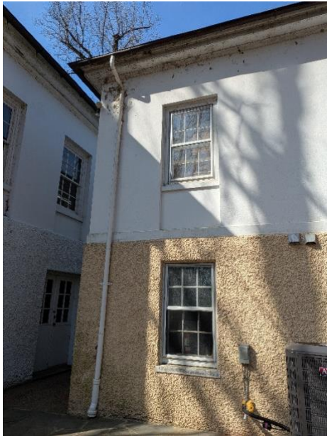
Photo P 007: Downspout
