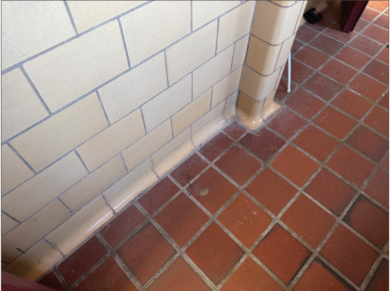
Figure 126. Glazed tile wall and quarry tile floor in first-floor vestibule. Building Conservation Associates, 2025.
