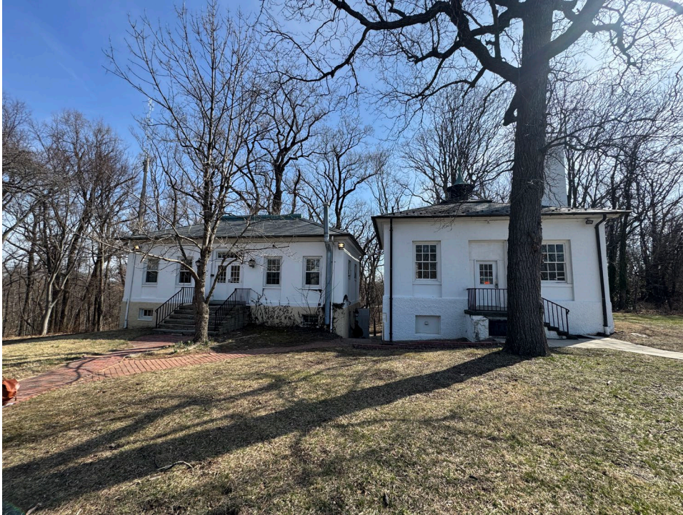
Figure 1. West elevation of Building #313 (left), next to the former Potting House (Building #314) (right). Note the similar hipped roofs, recessed windows, and two-colored stucco exterior walls.
