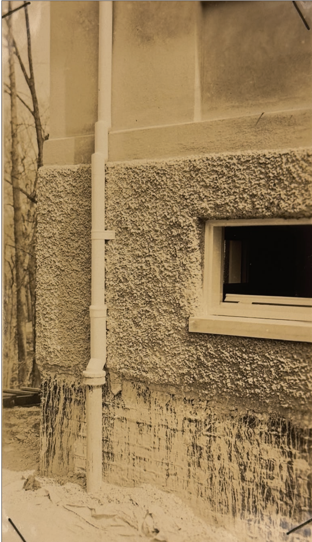
Figure 110. Painted copper downspout and cast-iron shoe, 1941. Nottingham, Completion Report, appendix.
