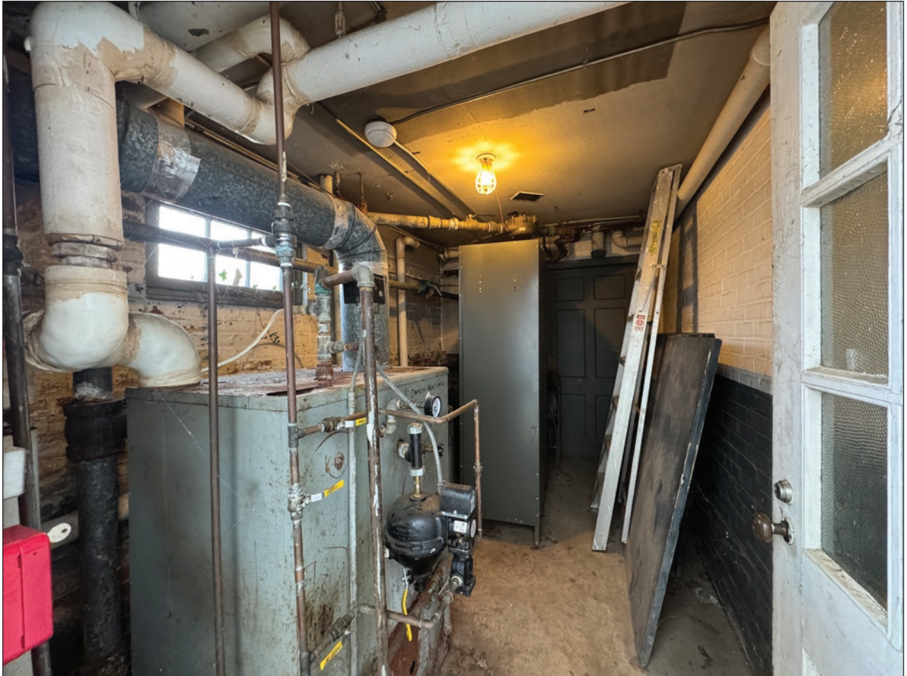
Figure 167. Southwest basement room. View looking north. Building Conservation Associates, 2025.
