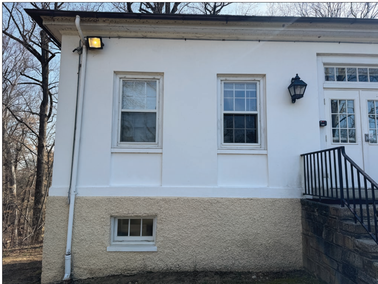
Figure 129. Double-hung first floor windows at west elevation. Building Conservation Associates, 2025.
