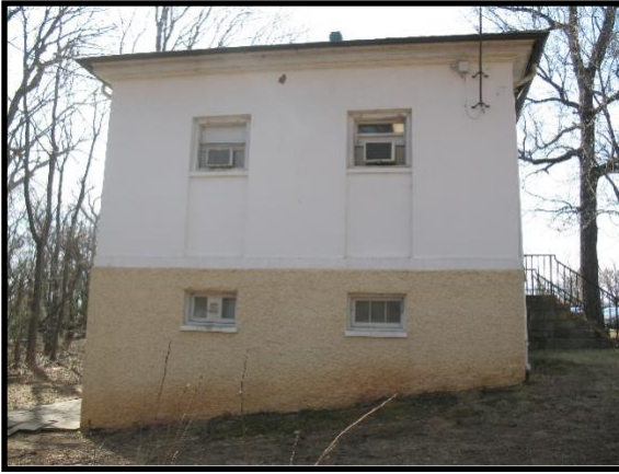
Photo P-3: North building elevation
