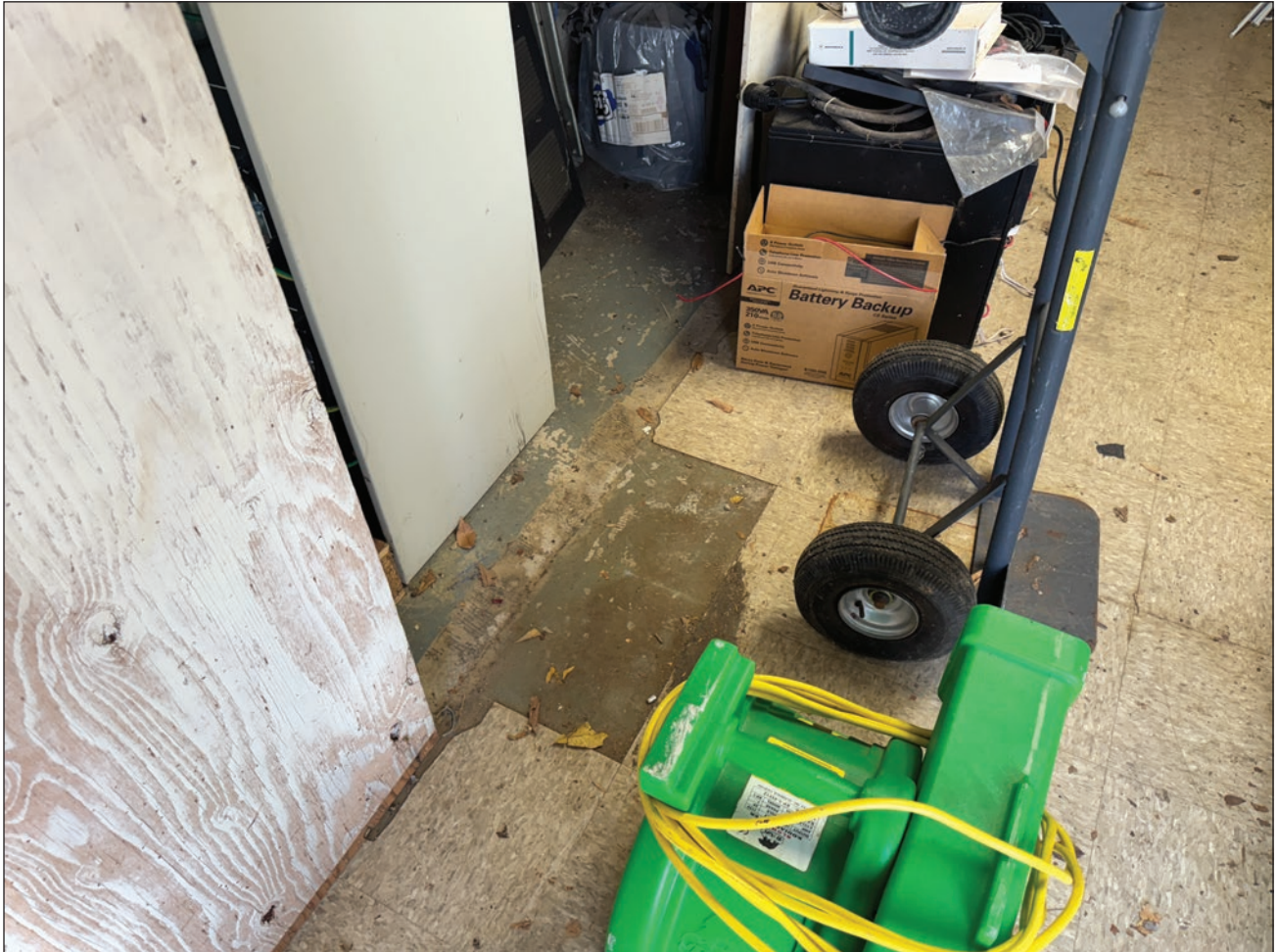
Figure 175. Concrete floor in the north basement storage room, partially covered with vinyl tiles. Building Conservation Associates, 2025.
