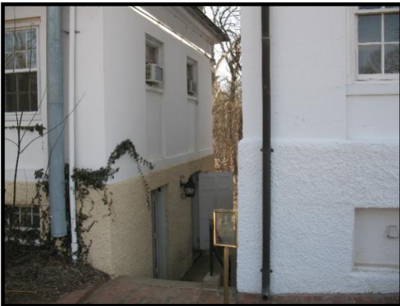
Photo P-5: Partial south building elevation
