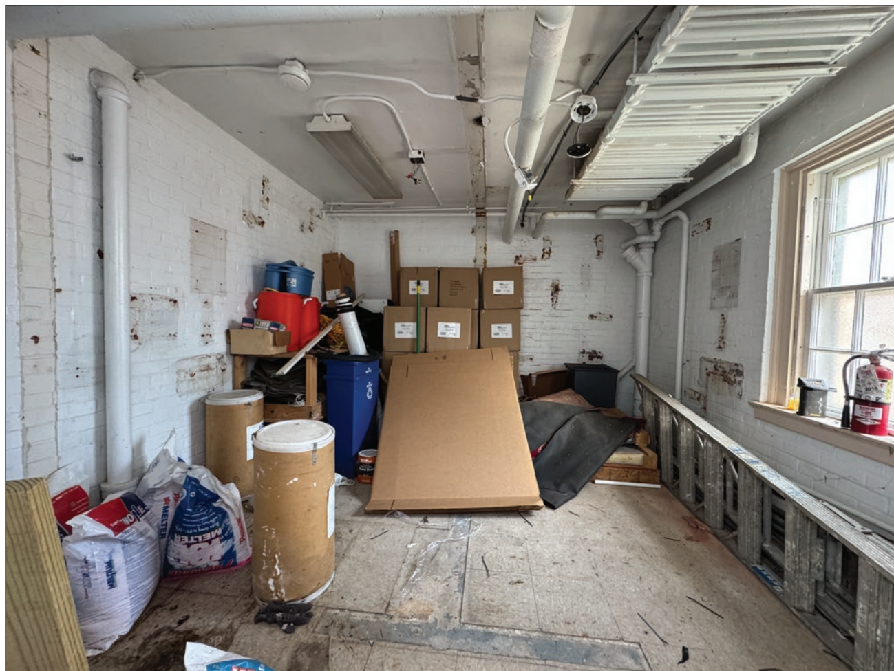
Figure 164. The former segregated men's toilet room, now used for storage. Building Conservation Associates, 2025.
