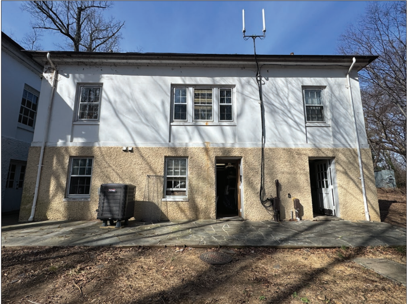
Figure 142. East elevation of Building #313. Note the center door that replaced an original window penetration. Building Conservation Associates, 2025.
