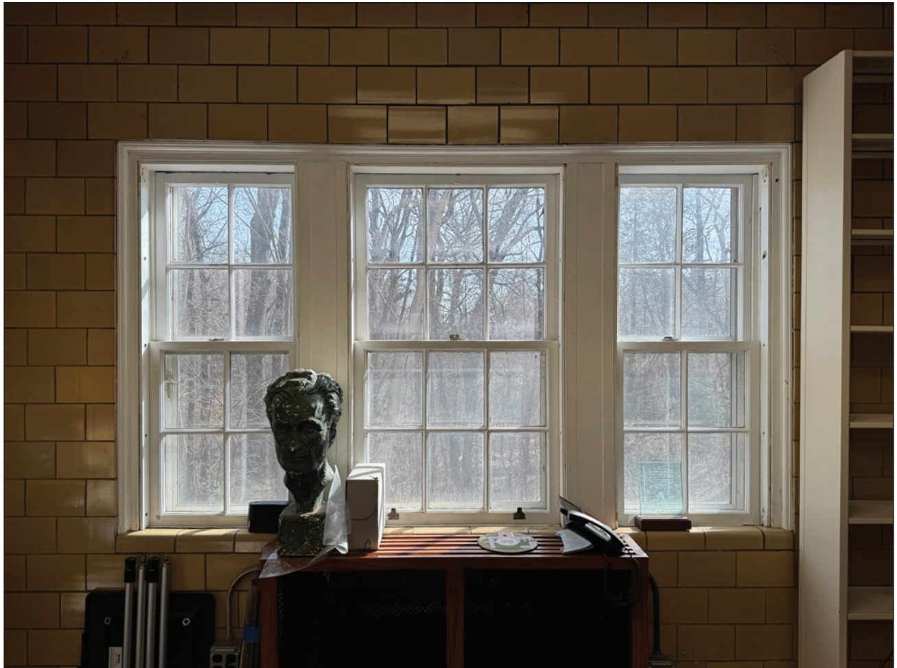
Figure 198. Tripartite window in east room. Building Conservation Associates, 2025.
