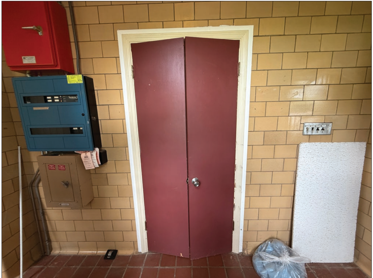
Figure 200. Double-leaf door at entrance to east room. Building Conservation Associates, 2025.
