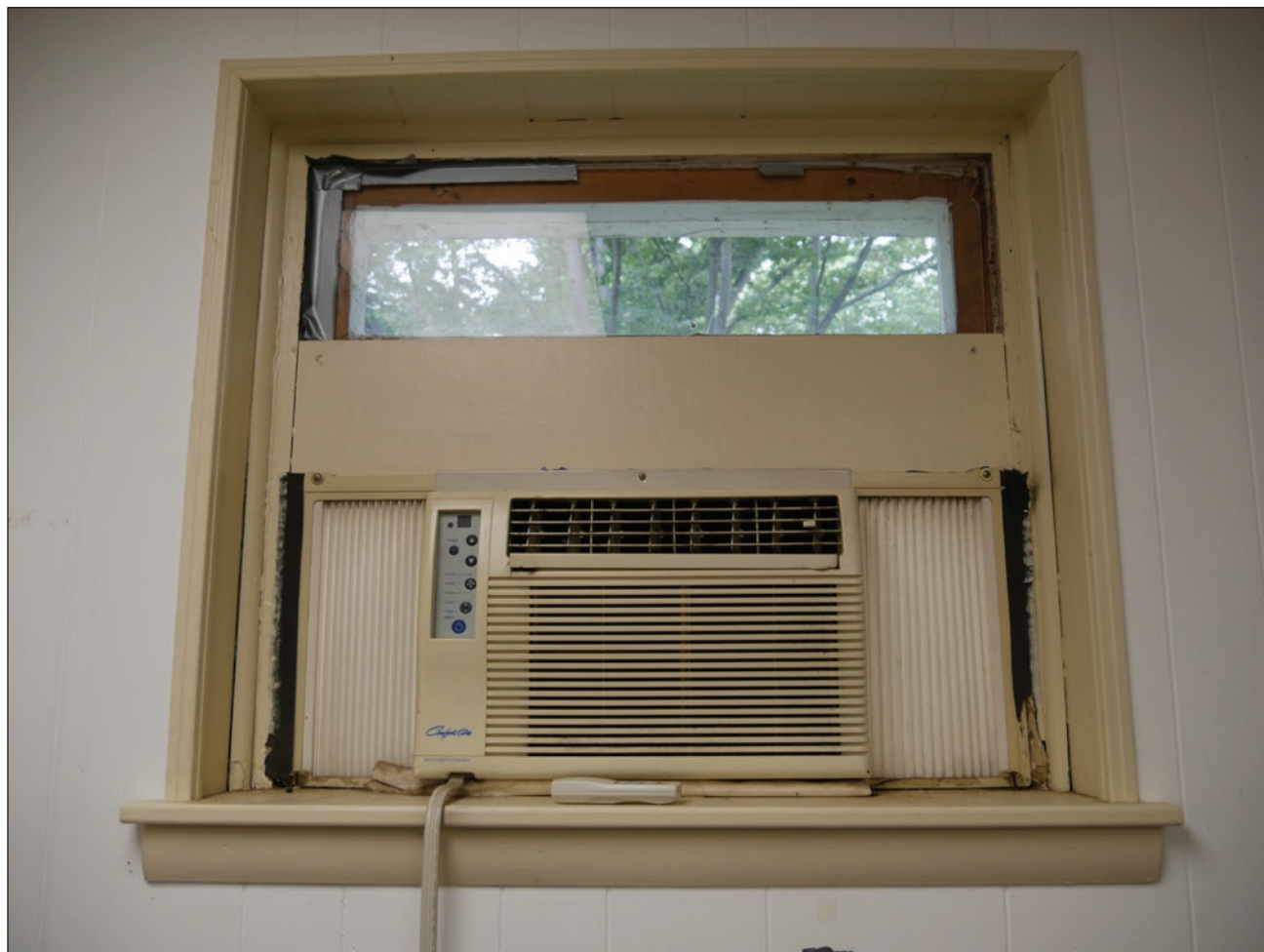
Figure 219. 2-over-3 sash window at north elevation modified for window A/C unit. Building Conservation Associates, 2025.
