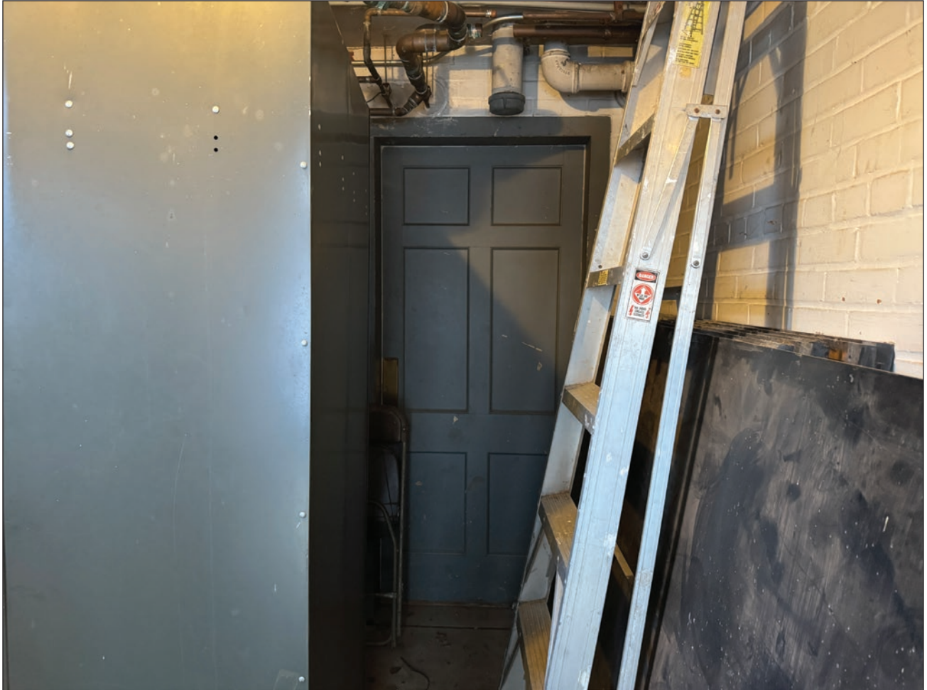
Figure 120. Paneled door separating southwest and center basement rooms. Building Conservation Associates, 2025.
