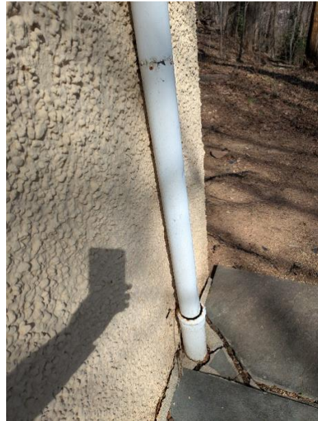
Photo P 008: Downspout
