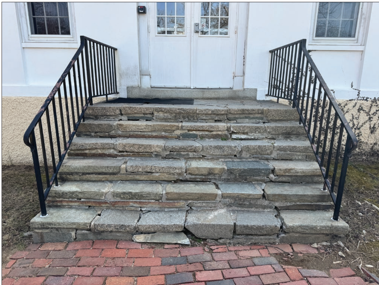
Figure 113. Granite stairs with wrought iron handrails at the main (west) entrance. Building Conservation Associates, 2025.
