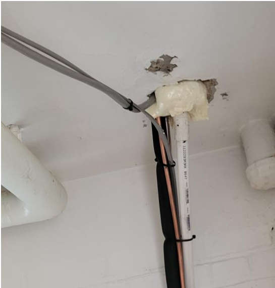
Photo E10: Electrical wiring improperly secured to building water pipe.
