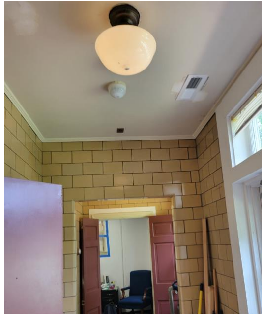
Photo E14: Vestibule area showing pendant-mounted luminaires.
