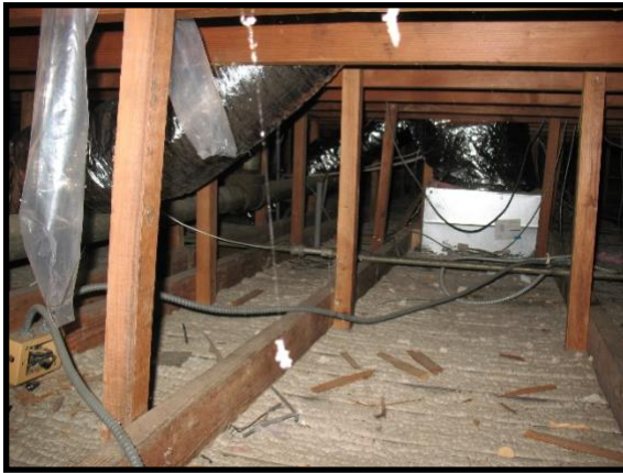
Photo P-11: First floor ceiling framing
