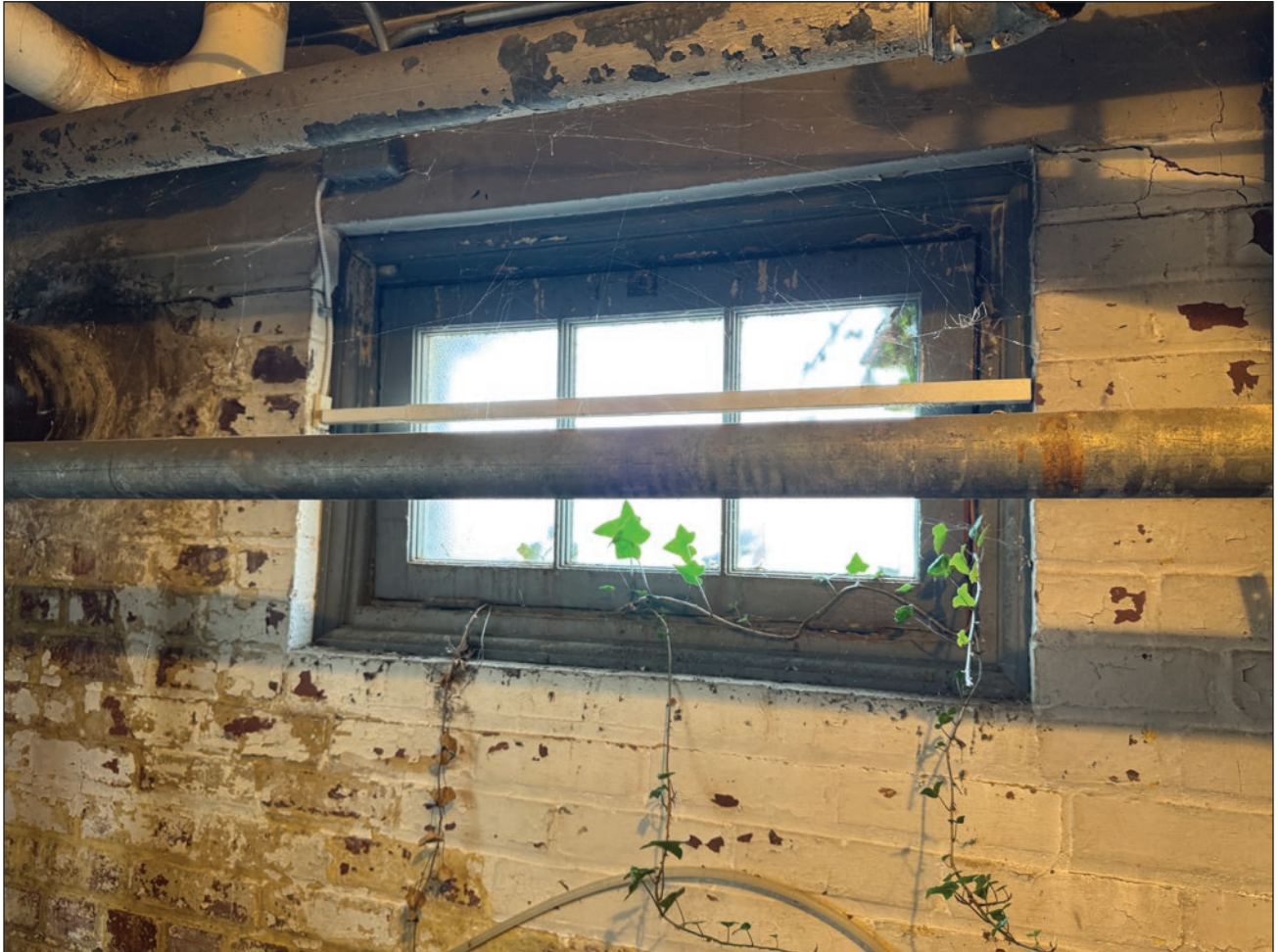
Figure 169. Obscured glass in the west hopper window of the southwest basement room. Building Conservation Associates, 2025.
