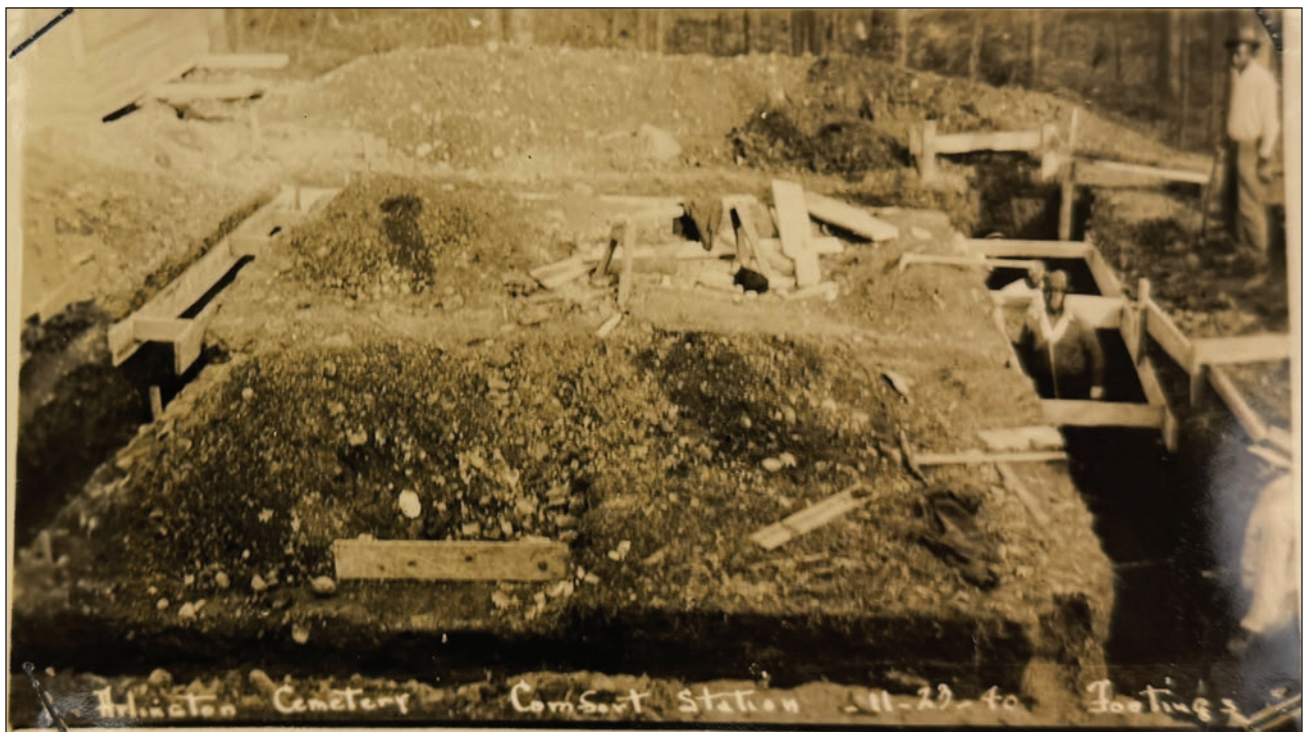
Figure 102. "Excavation for footings and foundations," 1941. Nottingham, Completion Report, appendix.
