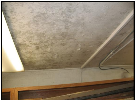
Photo P-14: First floor slab and interior brick bearing wall – east basement room
