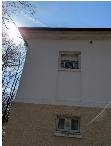
Photo M 018: Dryer Exhaust
