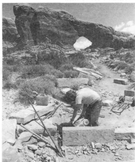
Trail work at North Window.
