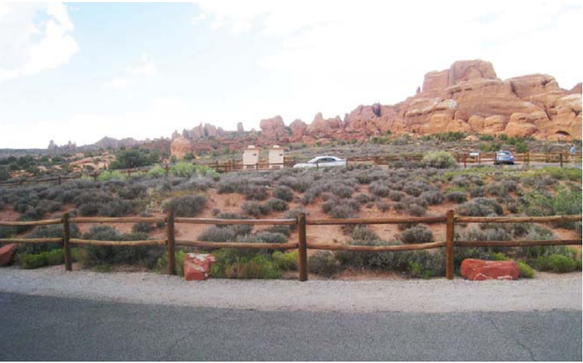
6 View to restrooms too prominent
