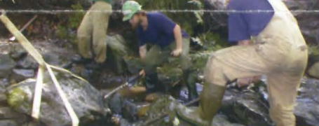
Volunteers repair a section of trail in Maryland.
