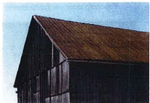
Standing seam roof.
