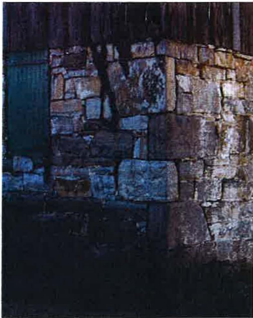
Northeastern corner of foundation.
