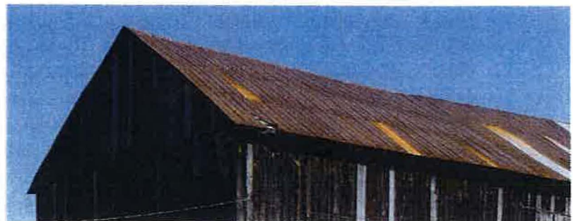
Metal seamed roof.
