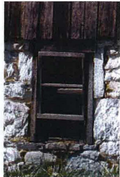
East elevation window.
