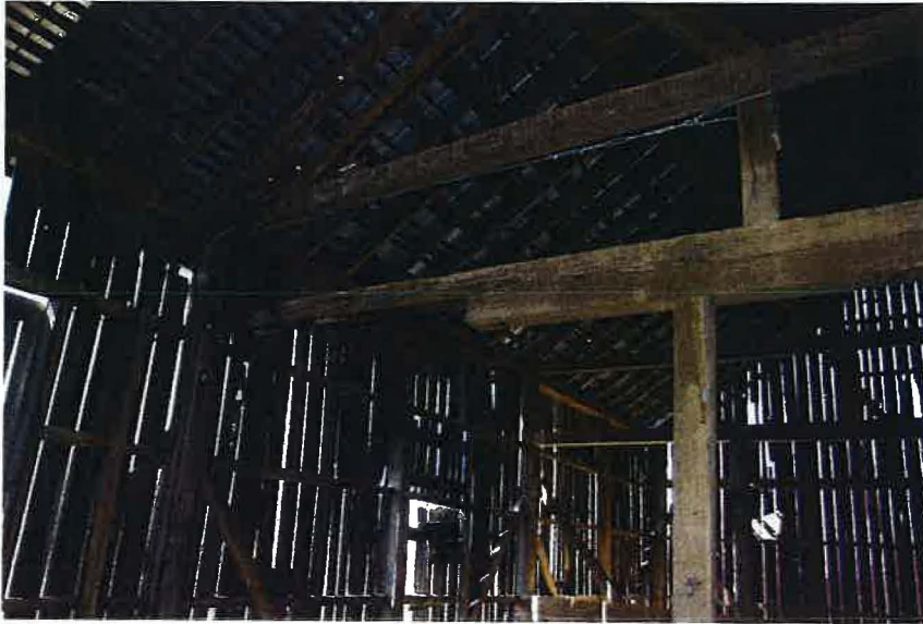
Deteriorated top sill plate and members.
