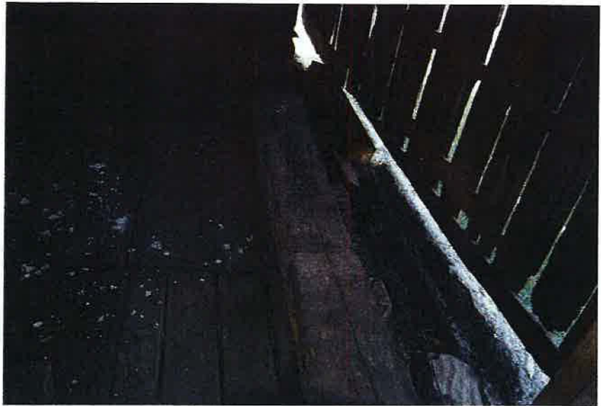
Deteriorated bottom sill plate.
