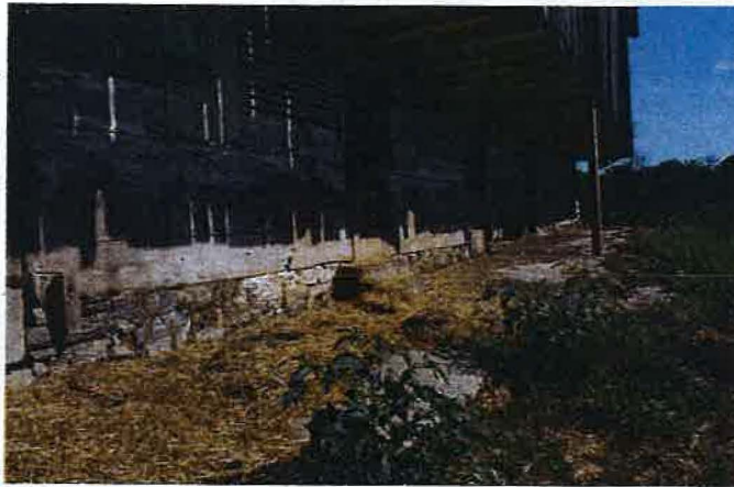
South elevation forebay.
