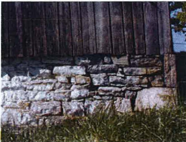
Foundation stones in north-east corner.
