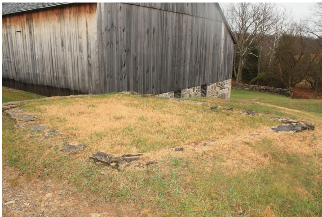
Trapezoid foundation north of the barn (NCR -CLP 2016).
