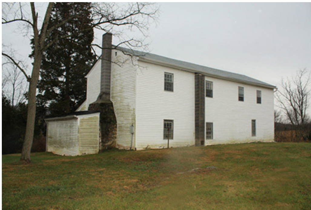
The Parks Farm main house from the rear elevation facing southeast (NCR CLP 2016).
