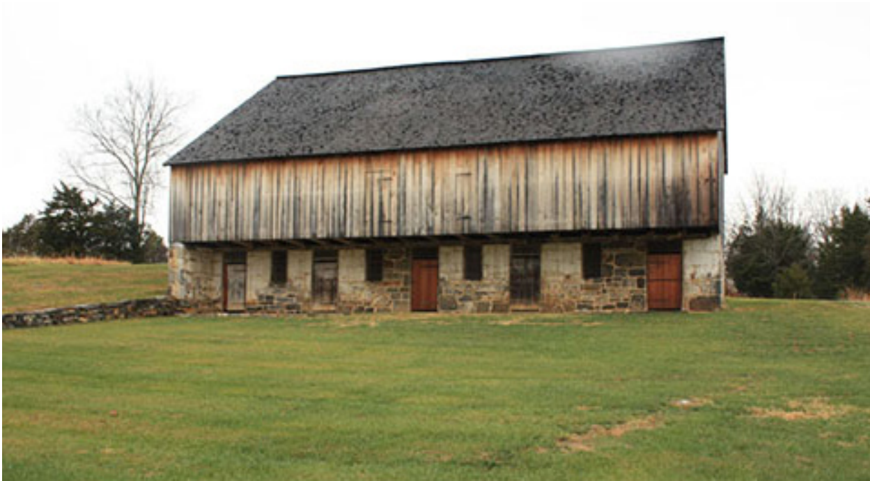
View of the south elevation of the Parks Barn after the rehabilitation (NCR CLP 2016).
