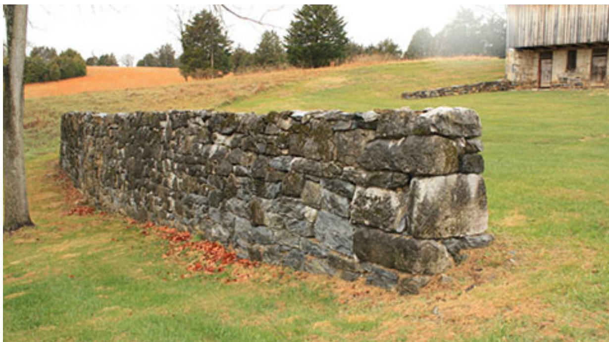
Barnyard Wall facing northwest (NCR CLP- 2016).
