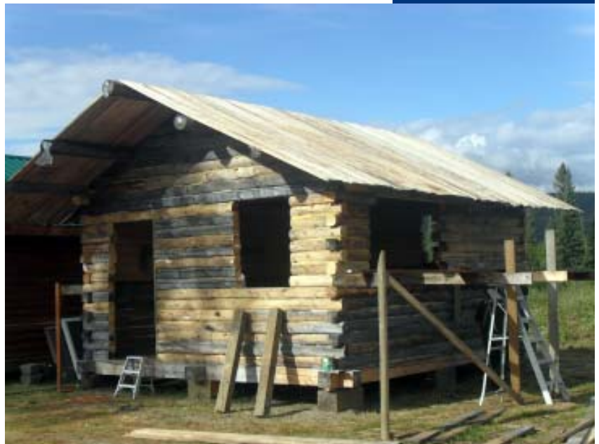
The maintenance team re-used some older logs for the new Fire Management office cabin in Eagle.
