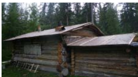
Washington Creek public use cabin received a new, temporary roof to prevent damage from rain and snow.
