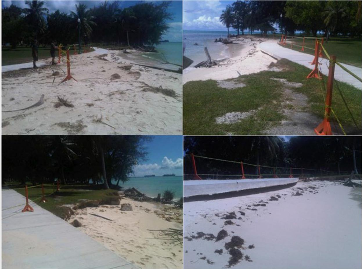
**Figure 25.** Photographs showing severe coastal erosion undermining a concrete walkway at the park. Stabilizing vegetation is all but destroyed along this section of the shoreline at the western edge of the park near the Japanese bunker site and Roseli Loop. Some threatened infrastructure was relocated inland. NPS photographs taken in 2012.
