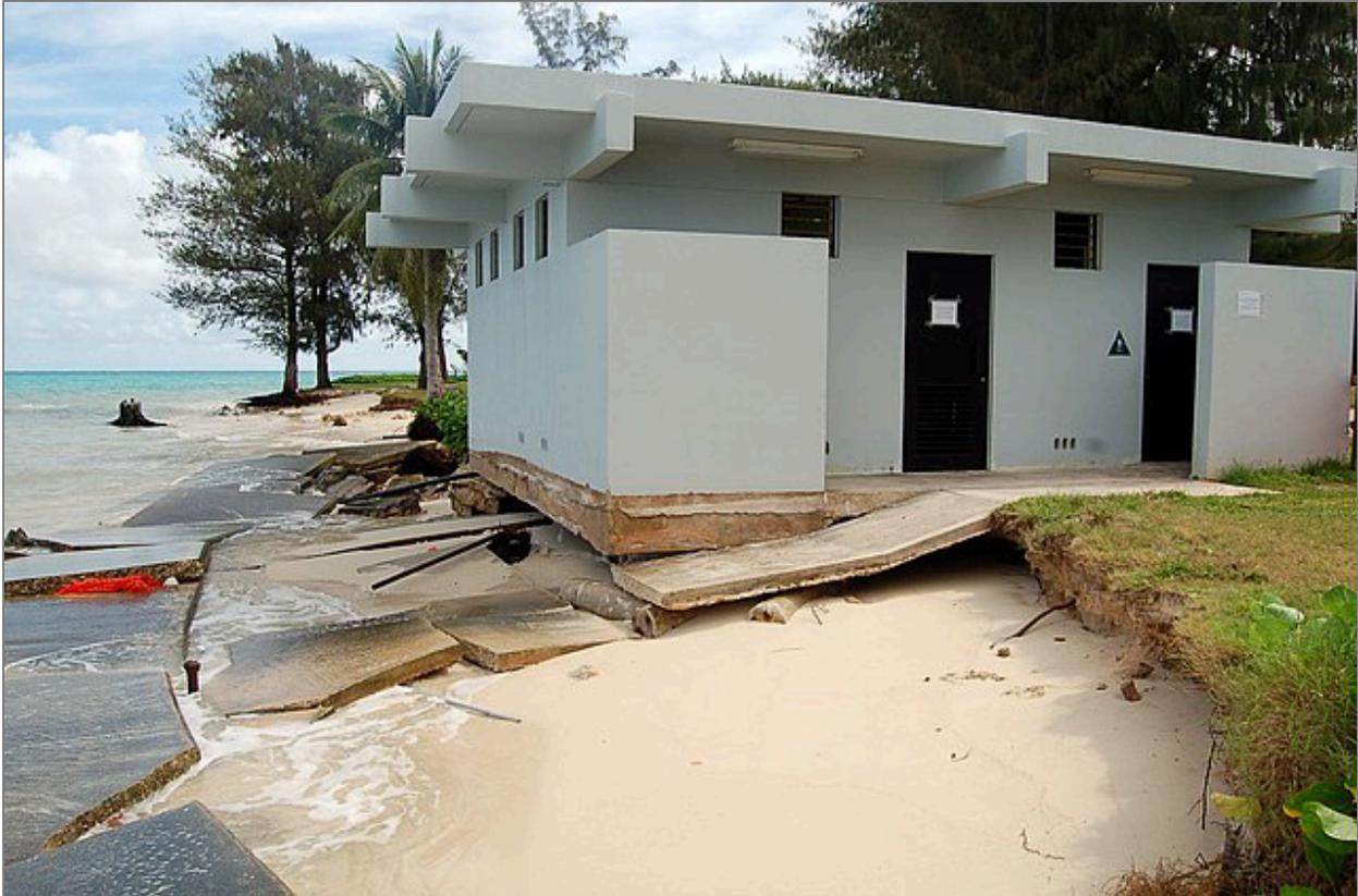
**Figure 24.** Photograph of storm damage at a park restroom. Many of the coastal areas along the western side of the park are eroding away due to high-energy wave impact. These facilities have since been relocated further inland, about 100 m (330 ft) away from the shoreline along Wedelia Avenue. NPS photograph taken in 2007.
