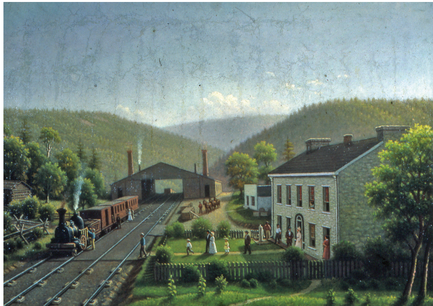
The Allegheny Portage Railroad was divided into segments referred to as levels and planes. The levels were relatively flat portions through which the rail cars were drawn initially by horses and later by locomotives. Stationary steam engines used ropes to haul railroad cars carrying boat sections and passengers up the planes or to let them down. A rail car at the top of one such plane can be seen entering the rear of the trainshed, circa 1900.
