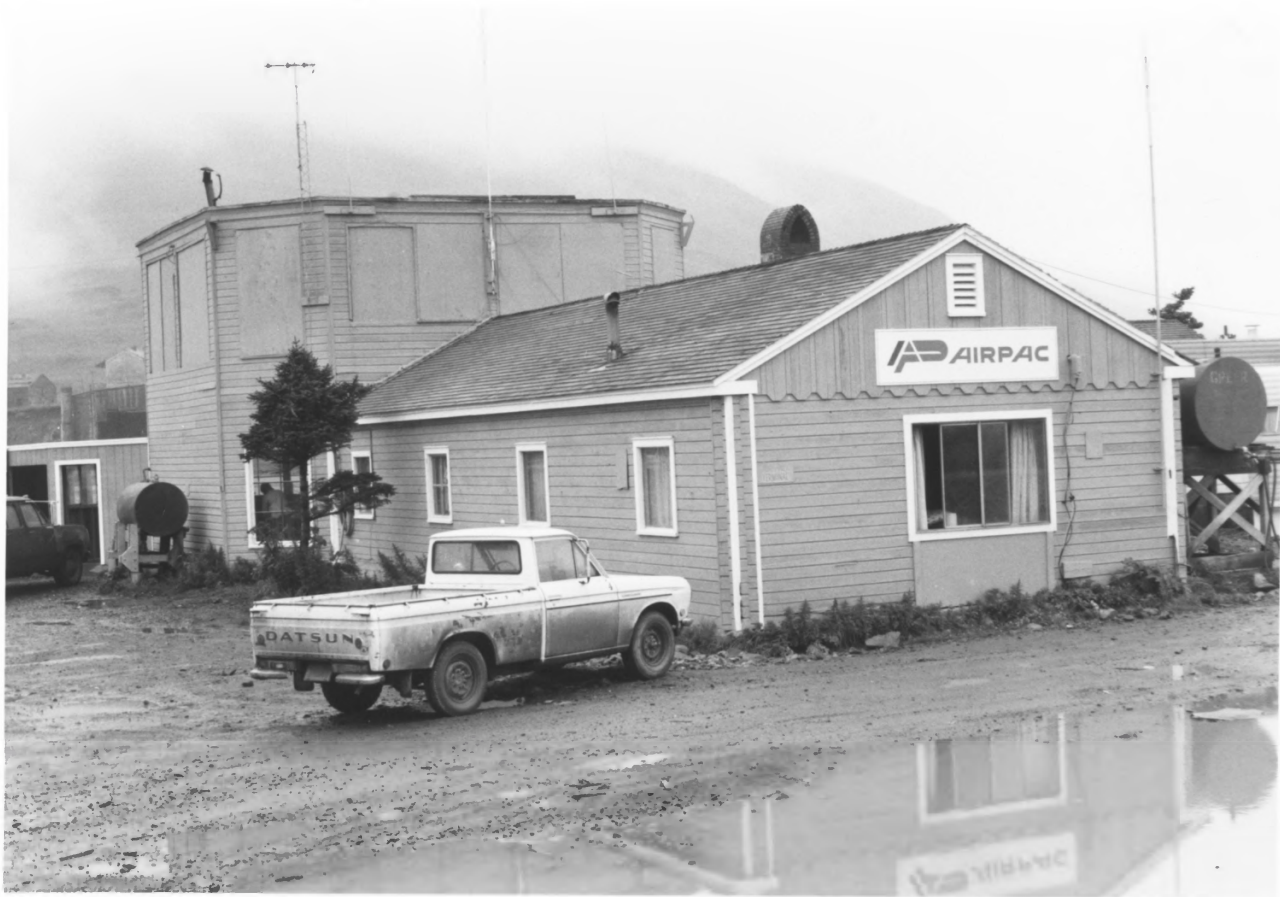
11. Navy's aerology (weather) and operations building at the airfield, Dutch Harbor. It presently serves as an airline terminal. On the floor of the waiting room is a handsome inlaid seal of the Naval Air Transport Service.
