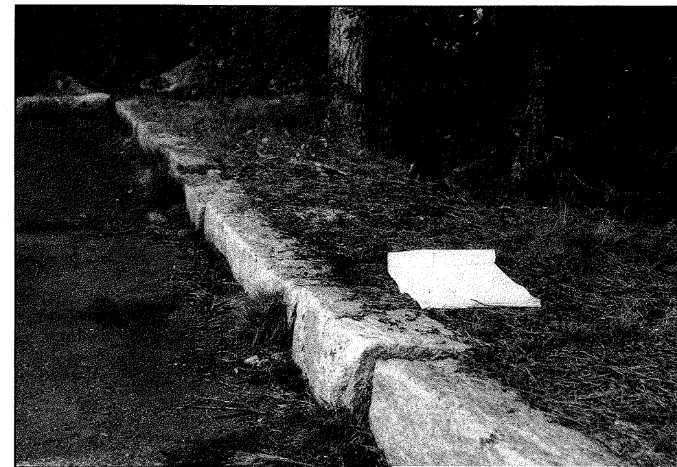
Figure 66 Granite curbing, typical of the Ocean Drive parking lots, station 375+00, 1993. Photograph by OCLP.
