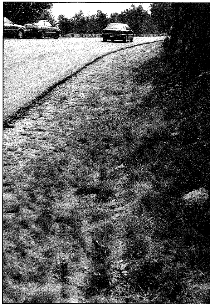
Figure 92 Existing rubble masonry waterway which is in poor condition, station 188+00, 1993. Photograph by OCLP.
