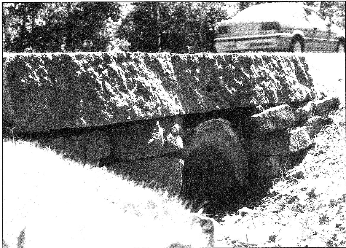
Figure 61 Reinforced concrete pipe culvert, dry-laid stone headwall, station 114+00, Paradise Hill Road, 1993. Photograph by OCLP.
