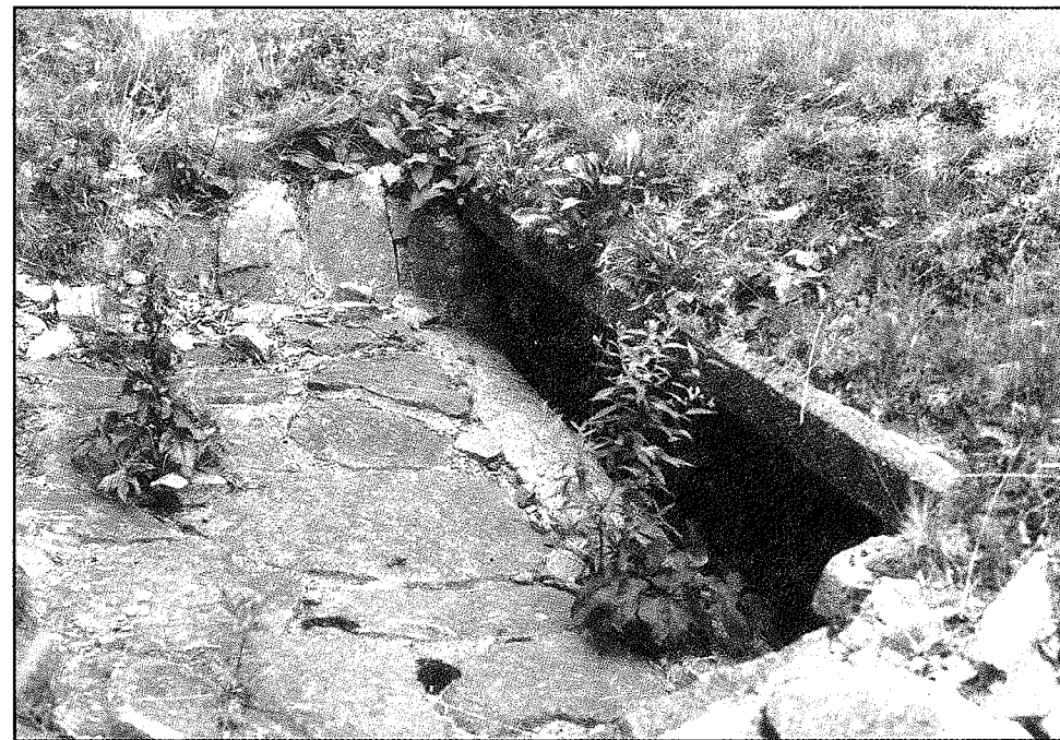
Figure 64 A post-1940 brick drop-inlet, BPR Project 4A2, station 196+00, 1993. Photograph by OCLP.
