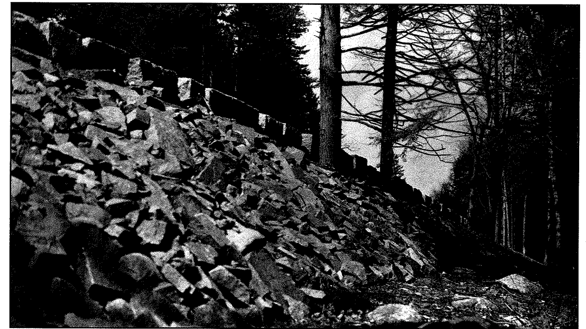
Figure 52 Kebo Mountain Road, hand-placed riprap embankment, 1938. Photograph from BPR, Progress Views .
