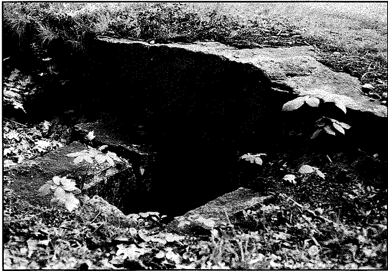
Figure 62 A dry-laid stone drop inlet, station 56+90, 1993. Photograph by OCLP.
