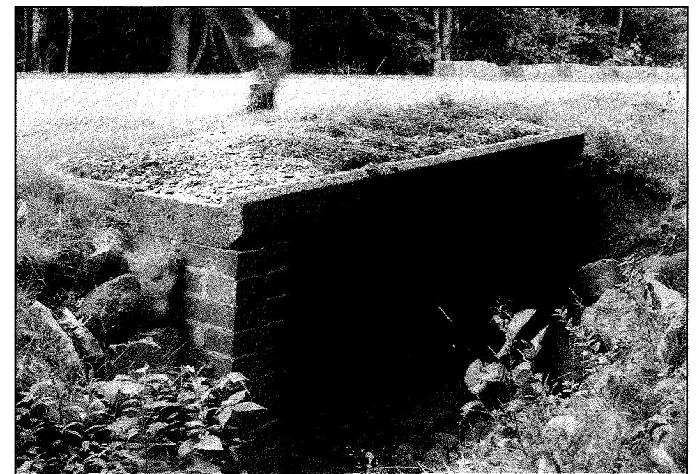
Figure 91 One of the two failing brick headwalls to be replaced, station 228+50, 1993. Photograph by OCLP.
