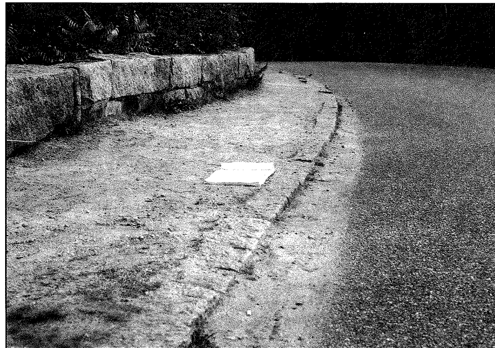
Figure 88 Historic curb reveal is threatened by additional bituminous overlay, station 365+50, 1993. Photograph by OCLP.
