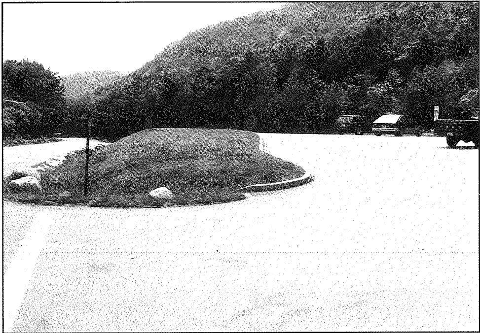
Figure 67 Concrete curbing, circa 1958, Precipice parking lot, station 240+00, 1993. Photograph by OCLP.
