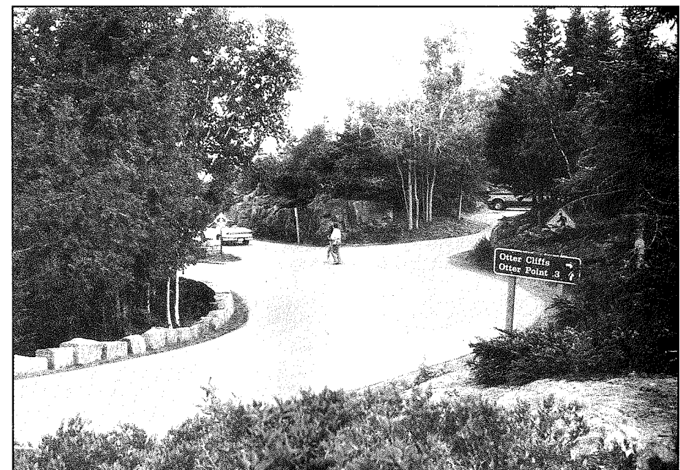
Figure 55 Coping stones of pink granite, Otter Cliff Road, station 392+00, 1993. Photograph by OCLP.
