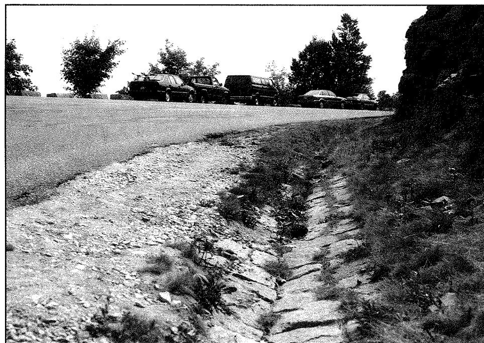
Figure 89 A steepened shoulder, caused by repeated overlay of bituminous material, station 188+00, 1993. A shoulder which is too steep is difficult to maintain. Photograph by OCLP.
