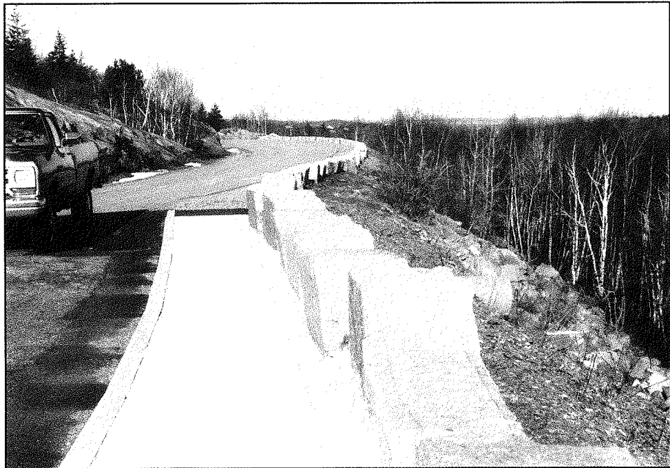
Figure 68 Champlain Mountain overlook, station 203+00, 1993. This highly finished granite curbing replaced concrete curbing installed in the 1950's. Photograph by OCLP.
