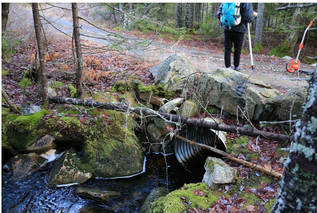
Figure 19. A substantial headwall/guardwall protects this culvert on the Loop Road. (OCLP 2016, IMG_0216)
