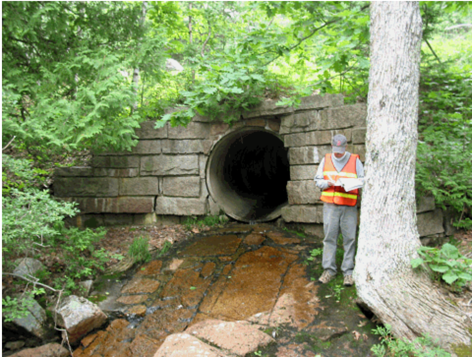
Figure 23. View of one of the historic motor road system's larger culverts and stone headwalls. Some of the most impressive structures are on Jordan Pond/Eagle Lake Road. (Acad0012_3.920_Out(1), OCLP 2005)
