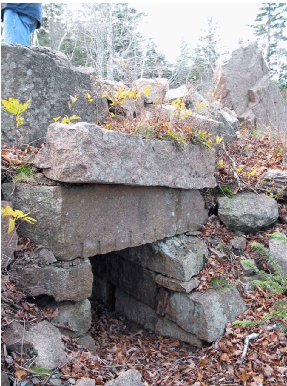
Figure 24. Stone box culverts are among the oldest drainage structures on the historic motor road system. This picture shows the stone work of an outlet on Cadillac Mountain Road. (Acad0013_0.920_Out, OCLP 2005)
