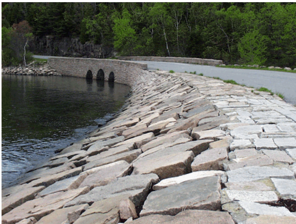
Figure 20. View of the curved causeway and bridge at Otter Cove. Unlike other bridges on the historic motor road system, this one is entirely masonry in construction. (Otter Cove Causeway 2, OCLP 1998)
