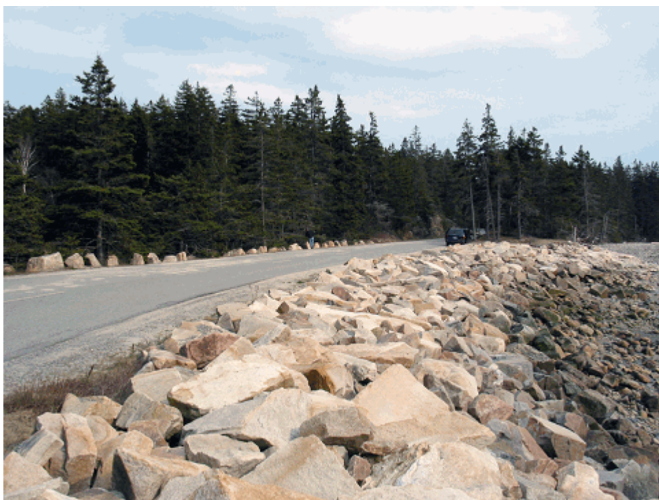
Figure 25. One of eighteen riprap embankments along Schoodic Loop Road. (Acad0301_2.430, OCLP 2005)
