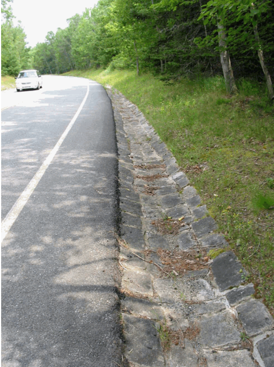
Figure 22. Mortared rubble waterways can still be found along the historic motor road system, such as this one on Jordan Pond/Eagle Lake Road. (Acad0012_4.801, OCLP 2005)
