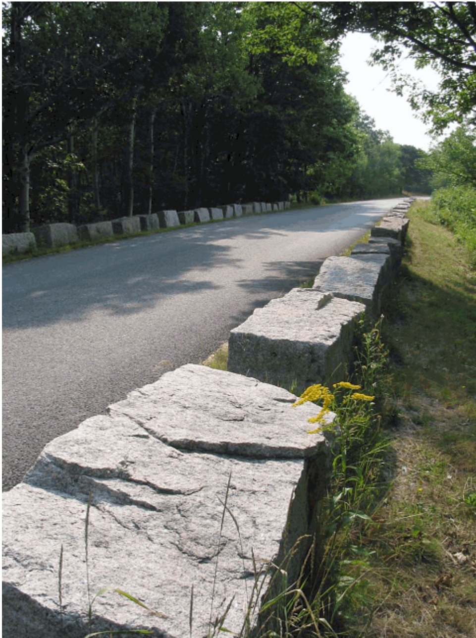
Figure 27. Guardwalls along Kebo Mountain Road feature rectilinear quarried stones. (Acad0300_1.723(2), OCLP 2005)
