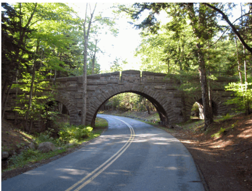
Figure 20. View of the curved causeway and bridge at Otter Cove. Unlike other bridges on the historic motor road system, this one is entirely masonry in construction. (Otter Cove Causeway 2, OCLP 1998)
