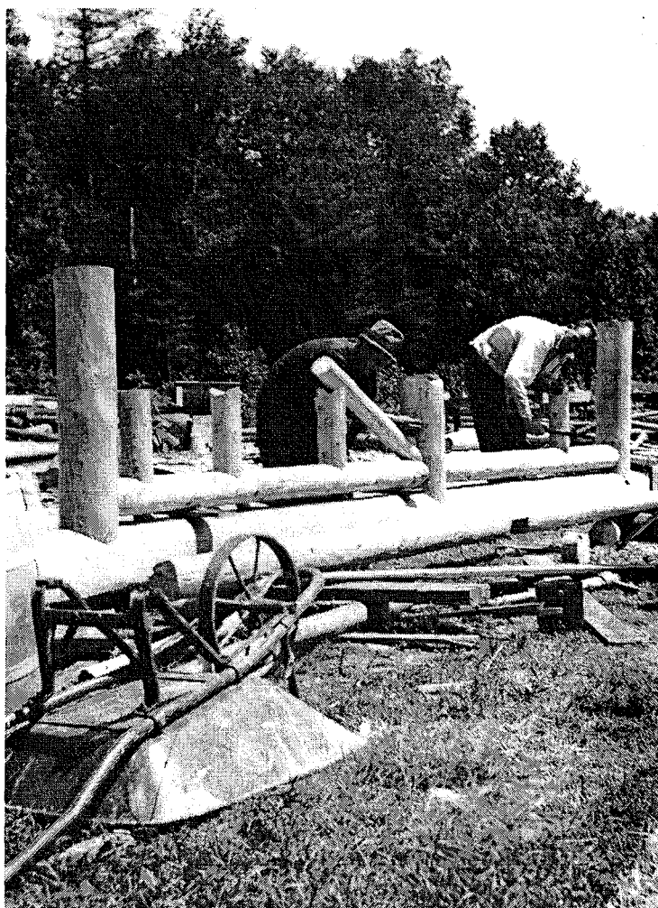
Figure 138: With the frames in place, decking was installed on site. (NARA Photo, Project scan number 312)
