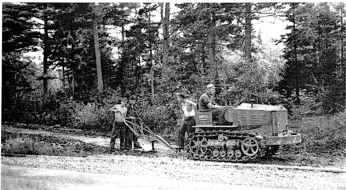
Figure 155: Ellsworth crews tearing up old pavement with an ordinary plow. Note the man standing on the shaft of the plow to keep the share from riding up out of the track. (NARA Photo, Project scan number 59)
