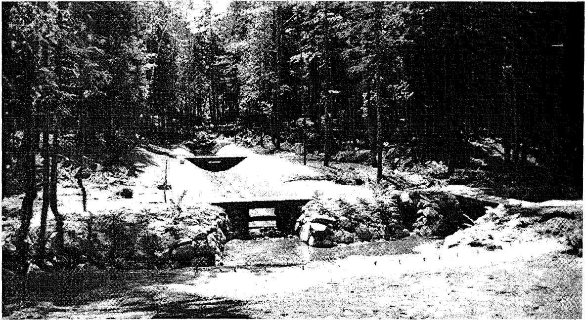
Figures 103 and 104: Project designers didn't always get it right the first time (or even the second). The above image documents the reconstruction in 1934 of fish rearing pools on Cold Brook, which had been built originally in 1933. The banks of the first pools were too steep and eroded quickly. The image below, taken in 1935, indicates that still further work was required to protect the banks of the pools. (NARA Photos, Project scan numbers 200 and 314)
