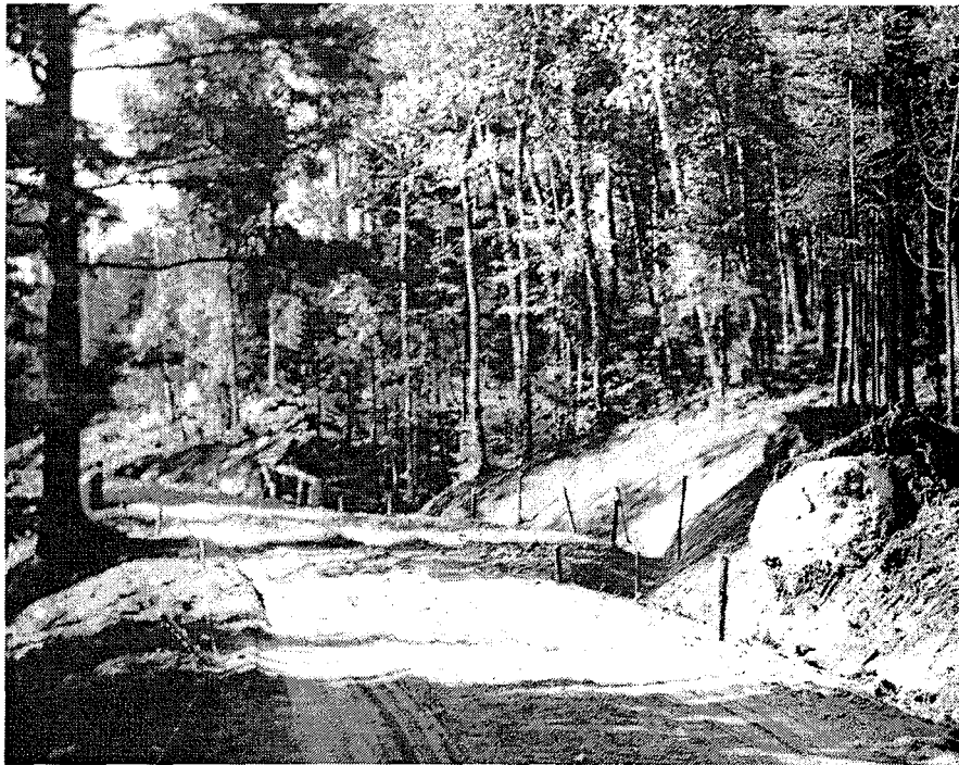
Figure 133: On the narrow roads, “turn- outs” were necessary at periodic intervals. Left, a turn-out on a Canada Hollow truck trail, under construction in 1935. (NARA Photo, Project scan number 298)
