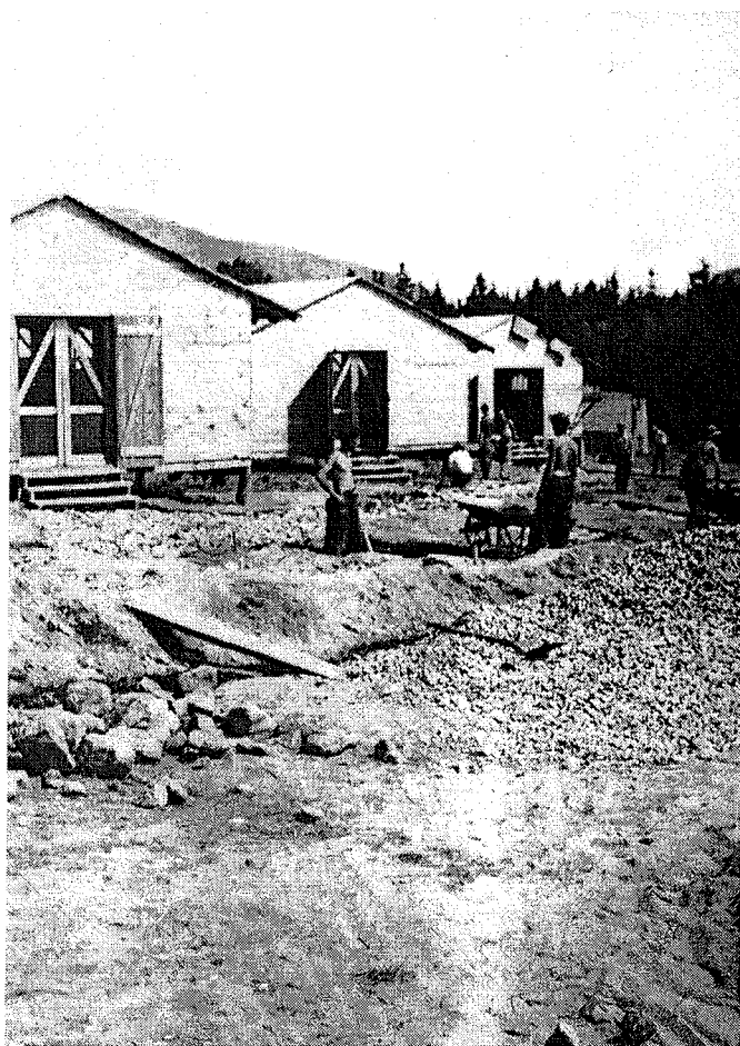
Figure 11: (Top) Barracks at the McFarland camp had to be built on posts to accommodate the contour of the hill. Initially, there was a concern that the buildings would not be habitable in winter, as a result. (Courtesy of John Parsons, NAFOH P8494)
