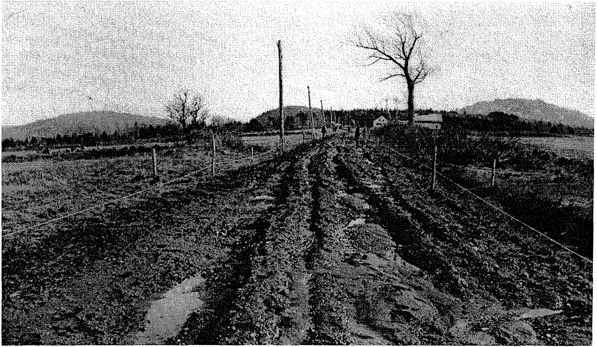
Figures 147 and 148: In the winter and spring of 1934, crews from the CWA and NP-2 filled and resurfaced the road leading to Beech Cliffs. These images give a “before and after” view of the same stretch of road. (NARA Photo, Project scan number 206)
