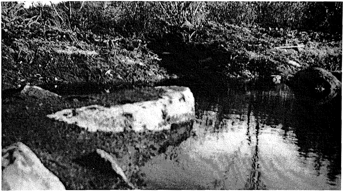
Figure 97: Stream improvement on Duck Brook. A channel has been cut through an abandoned beaver dam, clearing the way for fish to migrate upstream. (NARA Photo, Project scan number 287)
