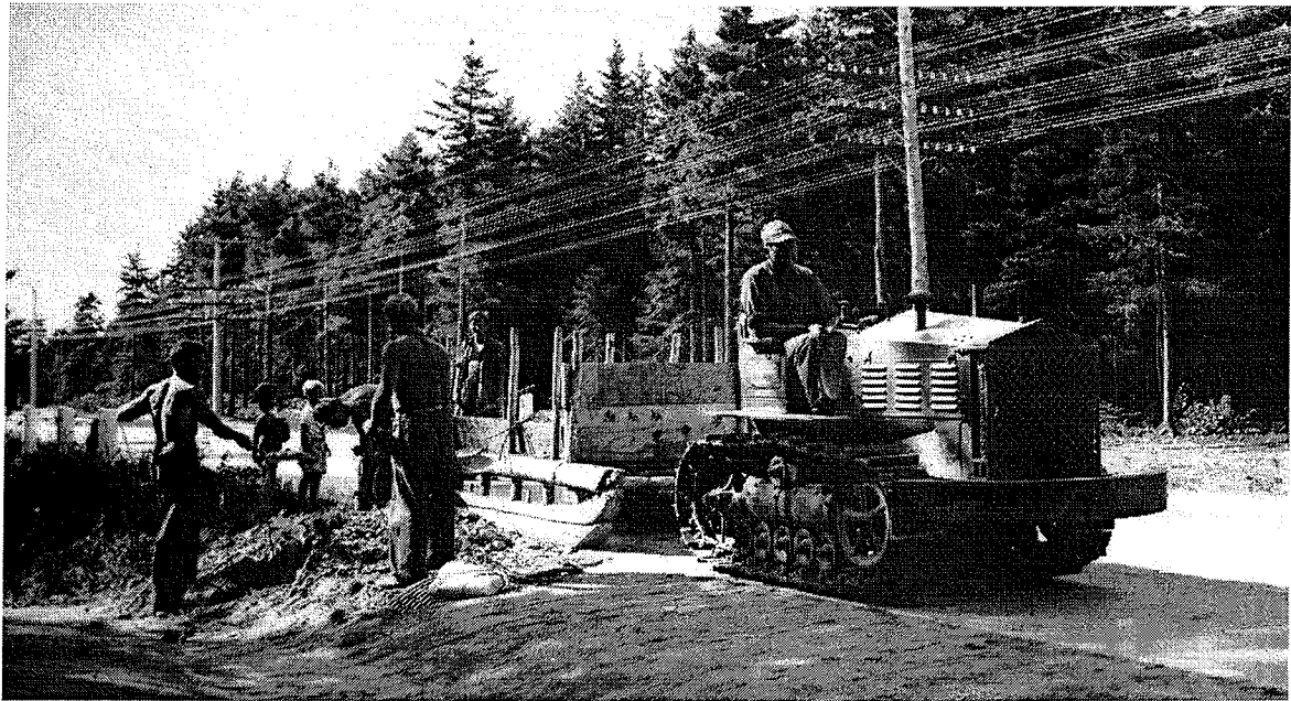
Figure 154: This small “Cletrac” tractor was the workhorse of the CCC at Acadia, one of the few pieces of “heavy” equipment available. For “accessories,” crews often had to improvise. Above, a sled is used to haul debris from the project site. (NARA Photo, Project scan number 91)
