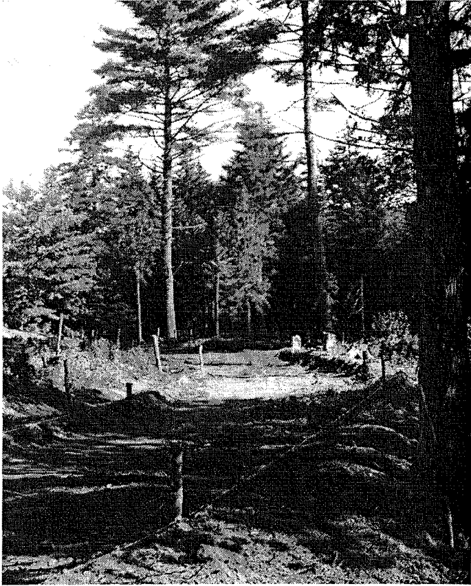
Figure 130: Marshy areas required a substantial base to stabilize the road. Here NP-1 crews prepare the foundation for a road at Sieur de Monts Spring (NARA Photo, Project scan number 375)
