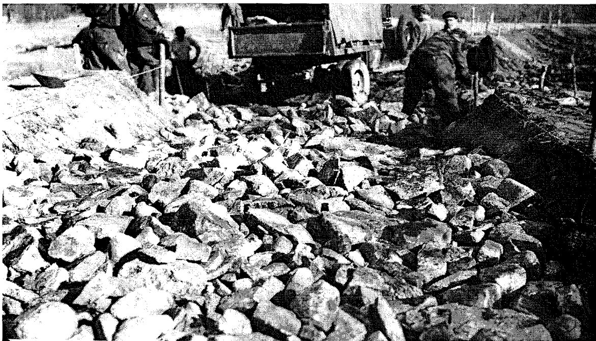
Figure 131: A layer of coarse stone is spread over a boggy section of the truck trail on the Schoodic Mountain Road. Part of the work performed by the SP-1 side camp on the Schoodic Peninsula in 1937. (NARA Photo, Project scan number 224)
