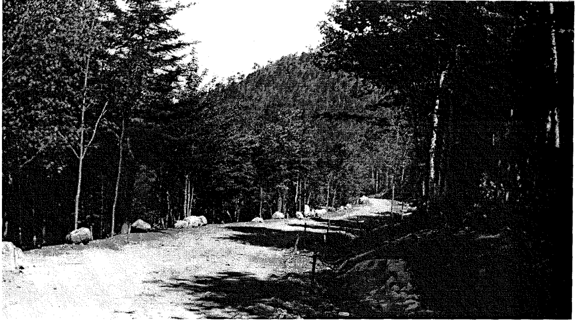
Figure 127: Most roads built by the CCC at Acadia were single-lane fire trails, intended primarily to move equipment and men to a problem area, and to provide access to nearby water supplies. Above is the Great Pond fire trail (NARA Photo, Project scan number 300)
