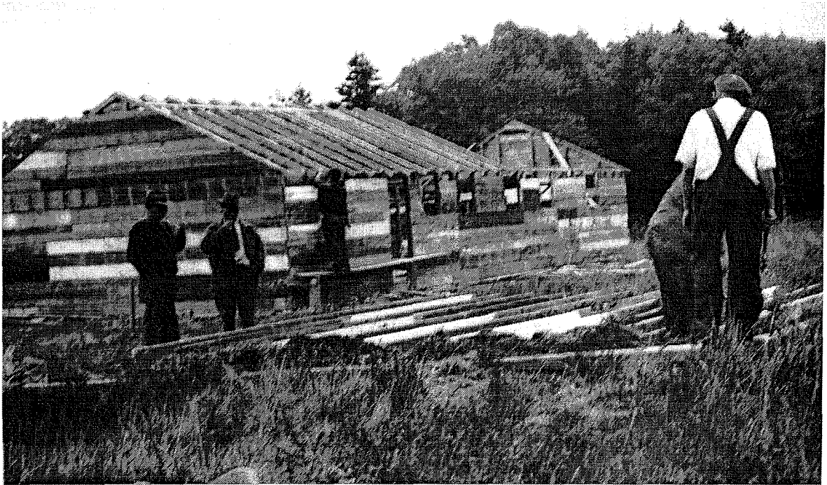
Figure 24: Construction of kitchen and mess hall at the Schoodic side camp ca. 1936. Building materials were salvaged from structures razed during cleanup operations at other work sites. (NARA Photo, Project scan number 138)
