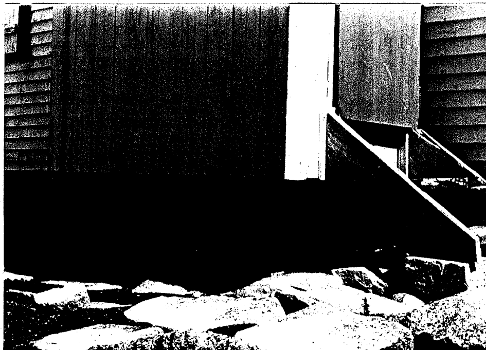
Figure 13. Foundation settlement at southwest corner. (BCB)
