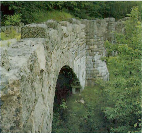
Sixteen stone bridges connect the carriage roads. The first hand-cut granite bridge was built in 1917, the last in 1933.
