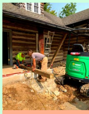
Front Porch replacements at the Knob Creek Tavern.
