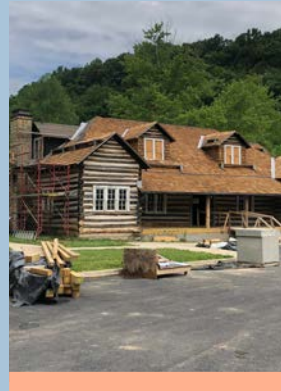
Lincoln Tavern Rehabilitation
