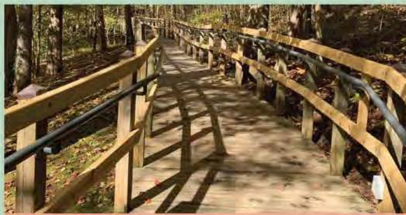
Birthplace wooden boardwalk with newly replaced handrails
