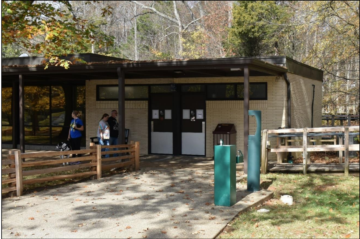
Photograph 3. Restroom at the east end of the Visitor Center, Abraham Lincoln Birthplace National Historical Park, facing northwest.
