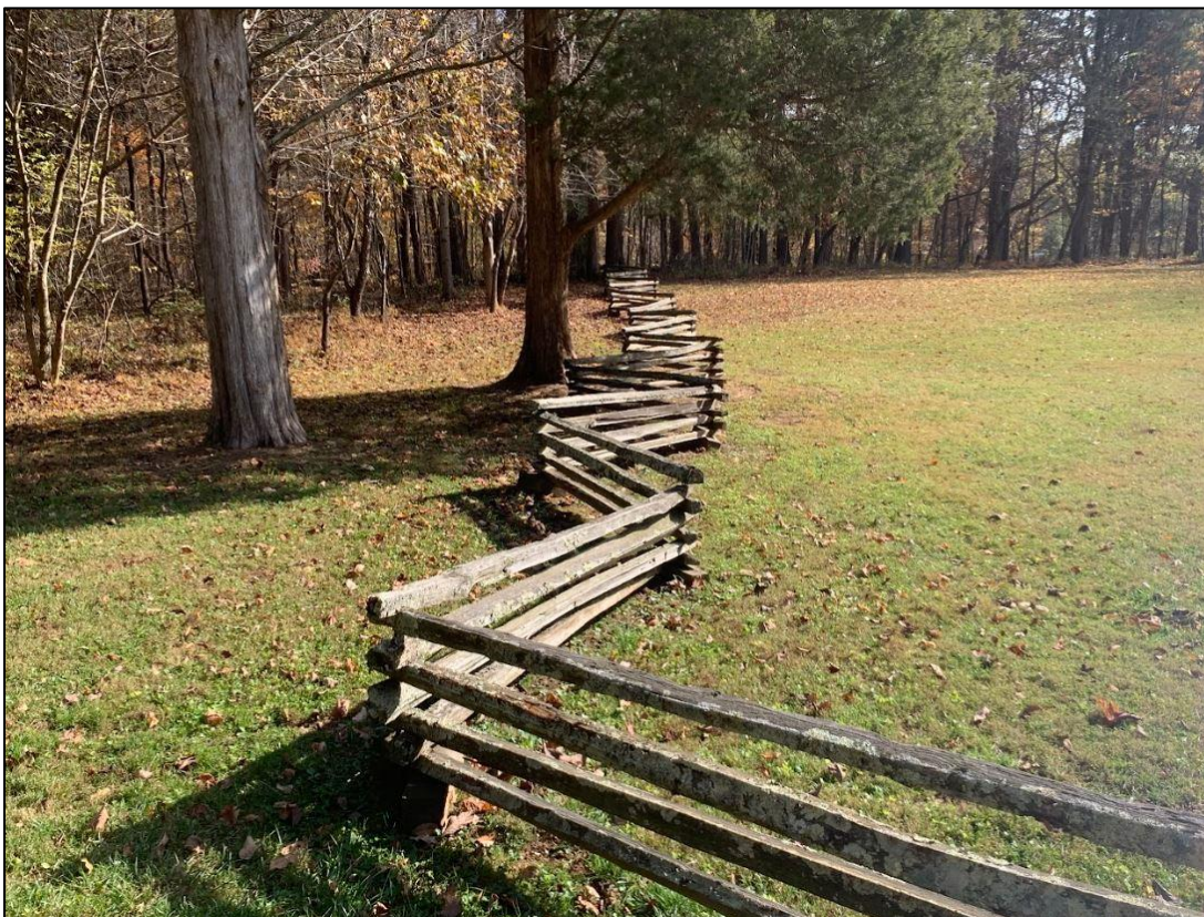
Photograph 4. Current photograph of the split-rail boundary fence, facing northeast.
