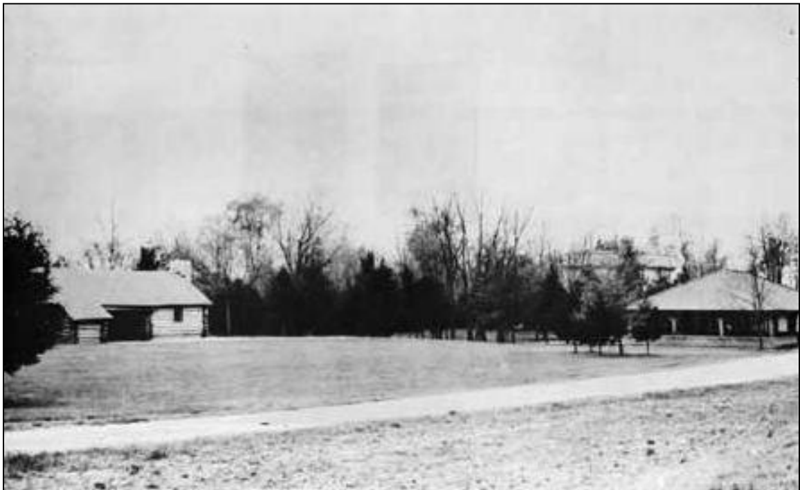
Figure 6. View of restroom and picnic pavilion constructed to the rear (northeast) of the Memorial Building, ca. 1939 (Image courtesy of Peterson 1968).
