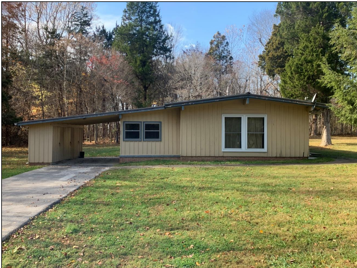
Photograph 2. Current photograph of the three-room residence, showing infilled screen porch and modern window replacements, facing west.
