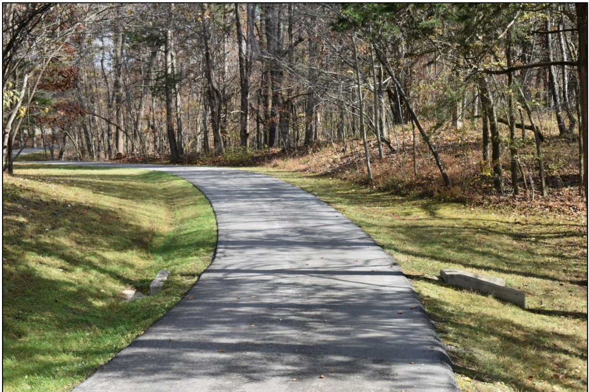
Photograph 8. Overview of the service road, showing concrete culverts along the north and south shoulders, facing east.
