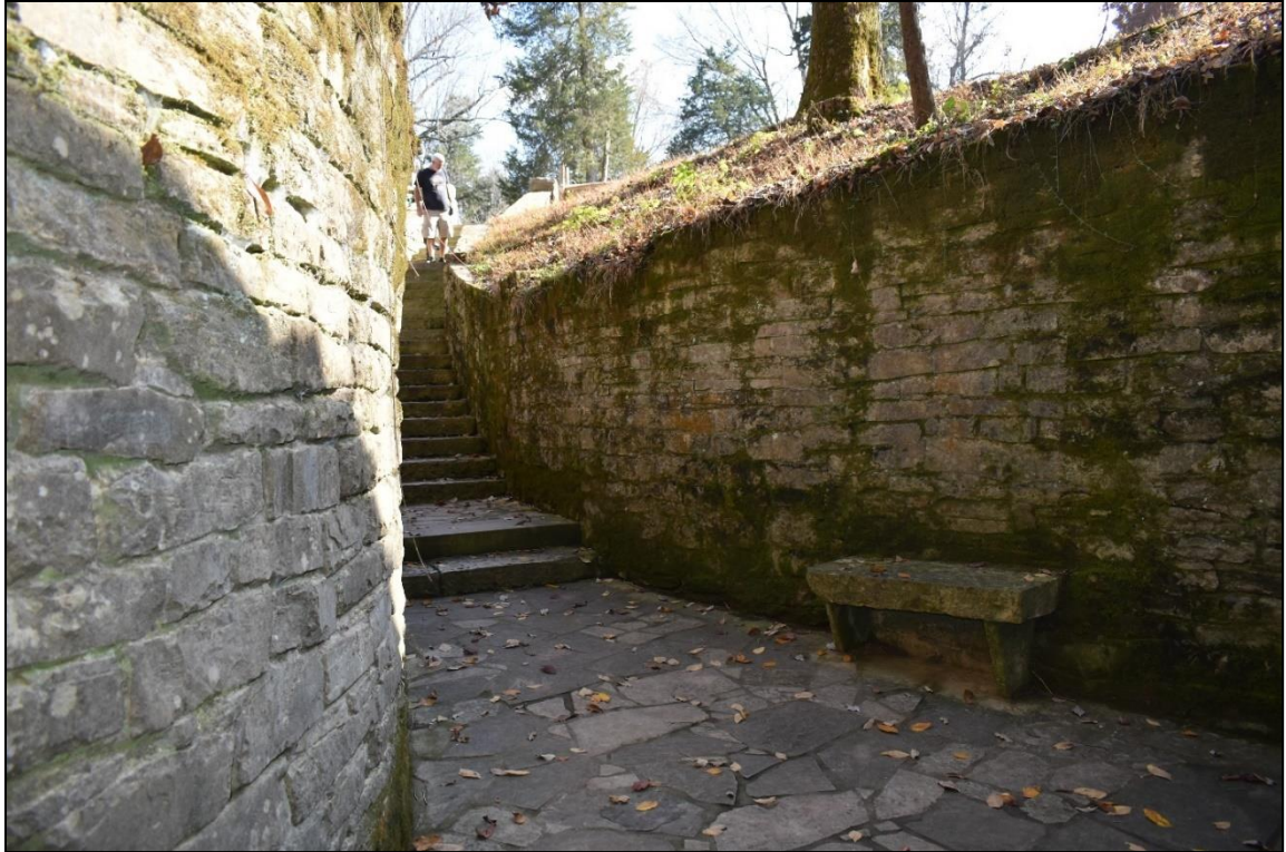
Photograph 21. Stone retaining walls, stairway, and bench at Sinking Spring, facing southeast.
