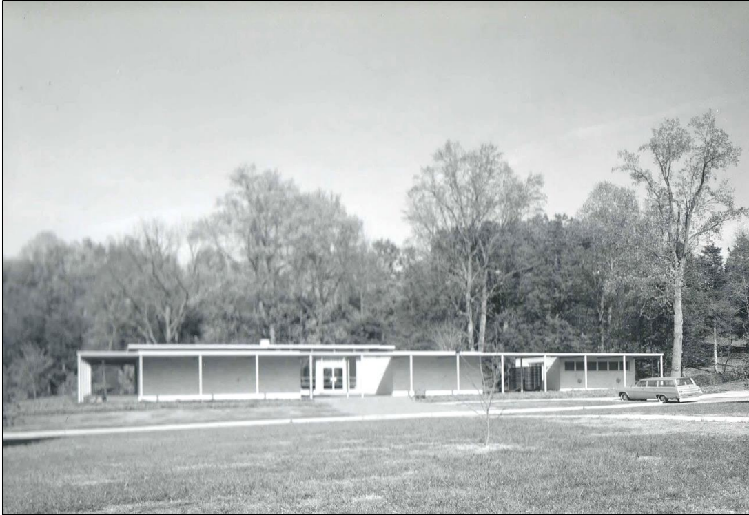
Figure 14. Primary (south) façade of the Visitor Center, ca. 1950s (Image courtesy of the NPS, Denver Service Center [ETIC no. 885373-ABLI_338_P19_0001_of_0001]).
