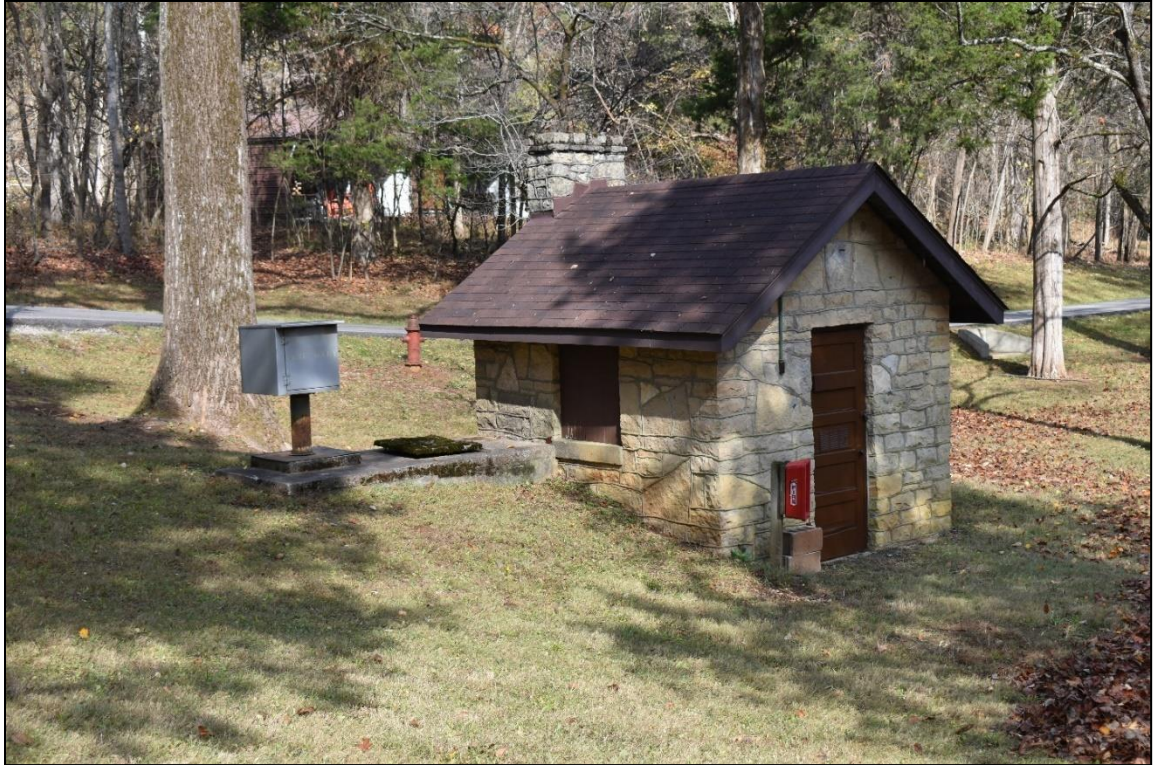
Photograph 7. Pump house located in the service area to the northwest of the Visitor Center, facing north.
