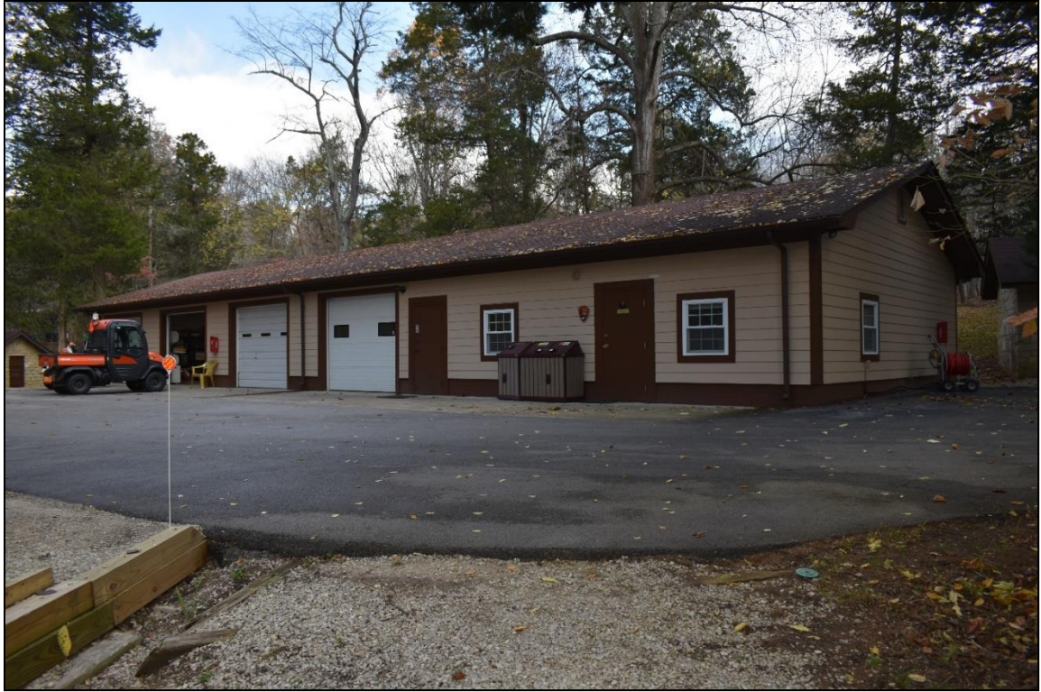
Photograph 5. Maintenance building in the service area to the north of the Visitor Center, facing northeast.
