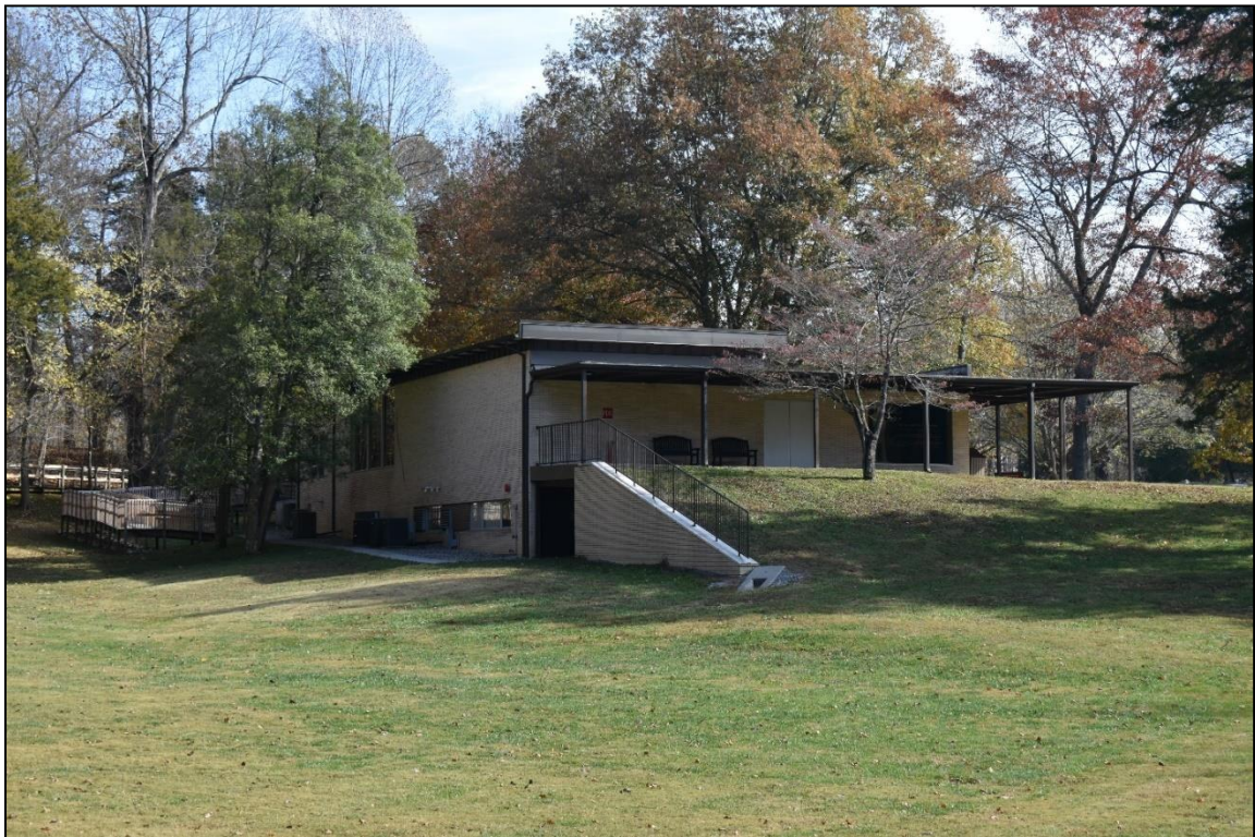
Photograph 4. North (rear) and west facades of the Visitor Center, facing east.
