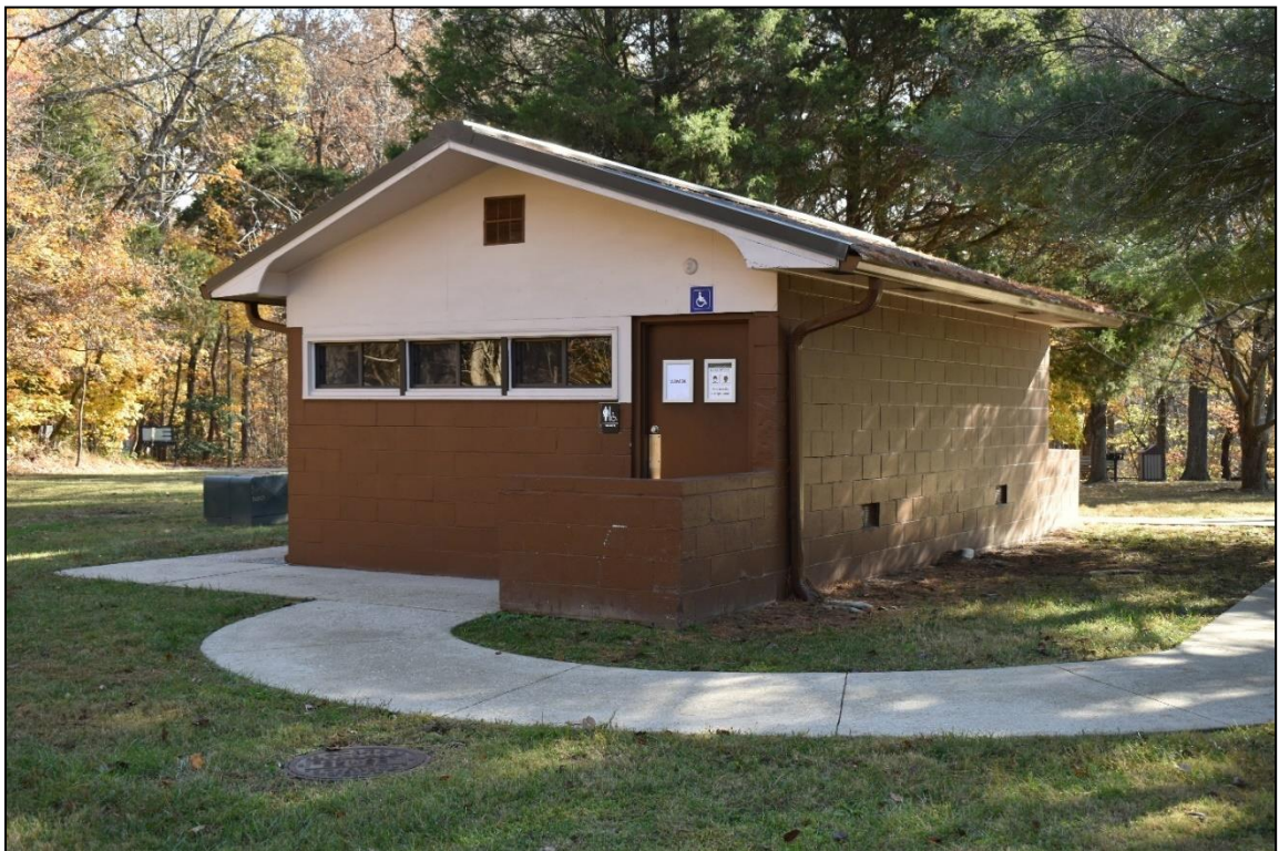
Photograph 31. North and west facades of the Picnic Area Comfort Station, facing southeast.
