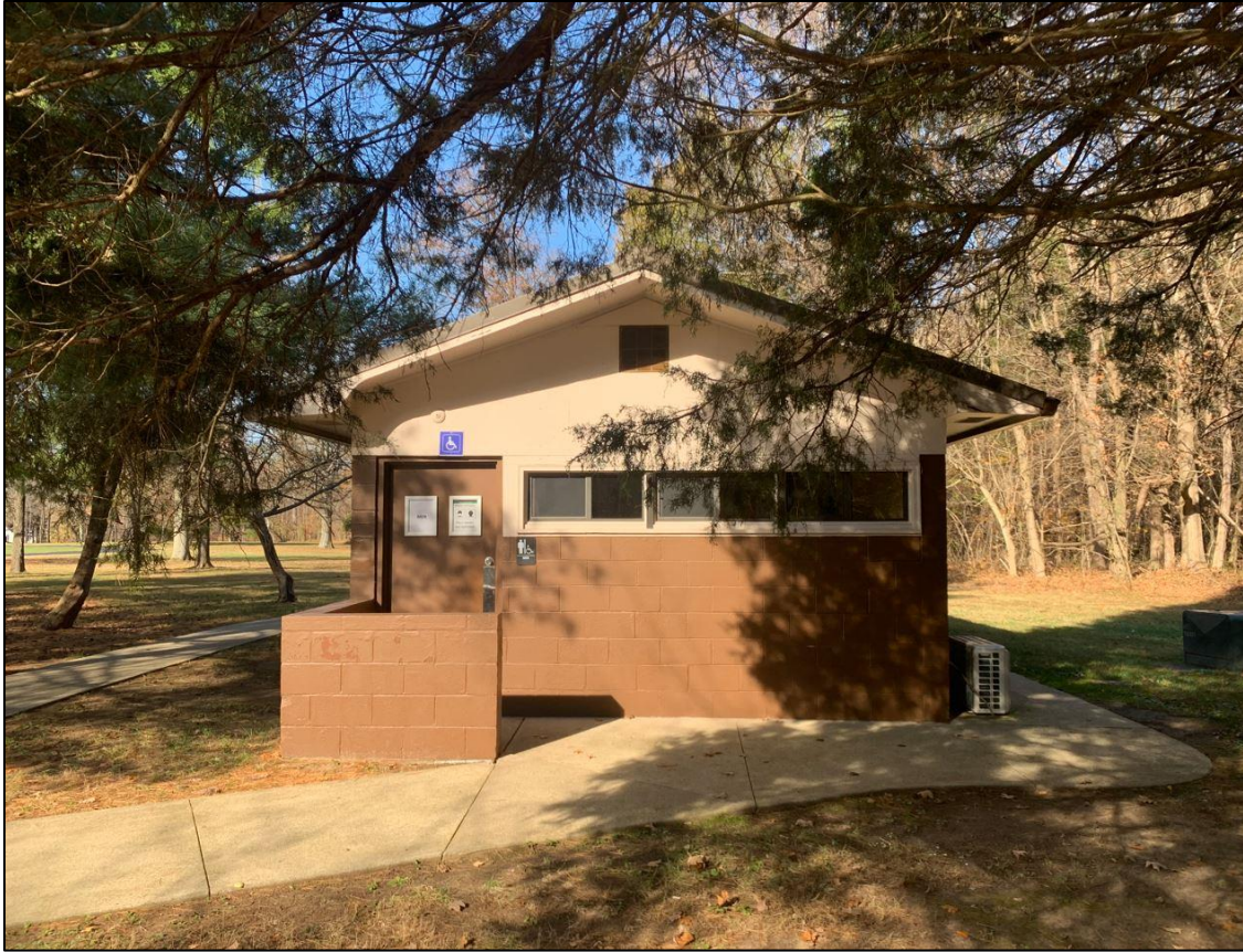
Photograph 3. Current photograph of the picnic area comfort station, facing north.
