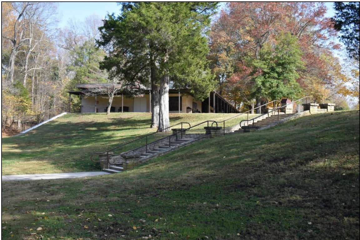
Photograph 24. Paved walkway and stairway leading from the Visitor Center parking area to the Memorial Building, facing northeast.
