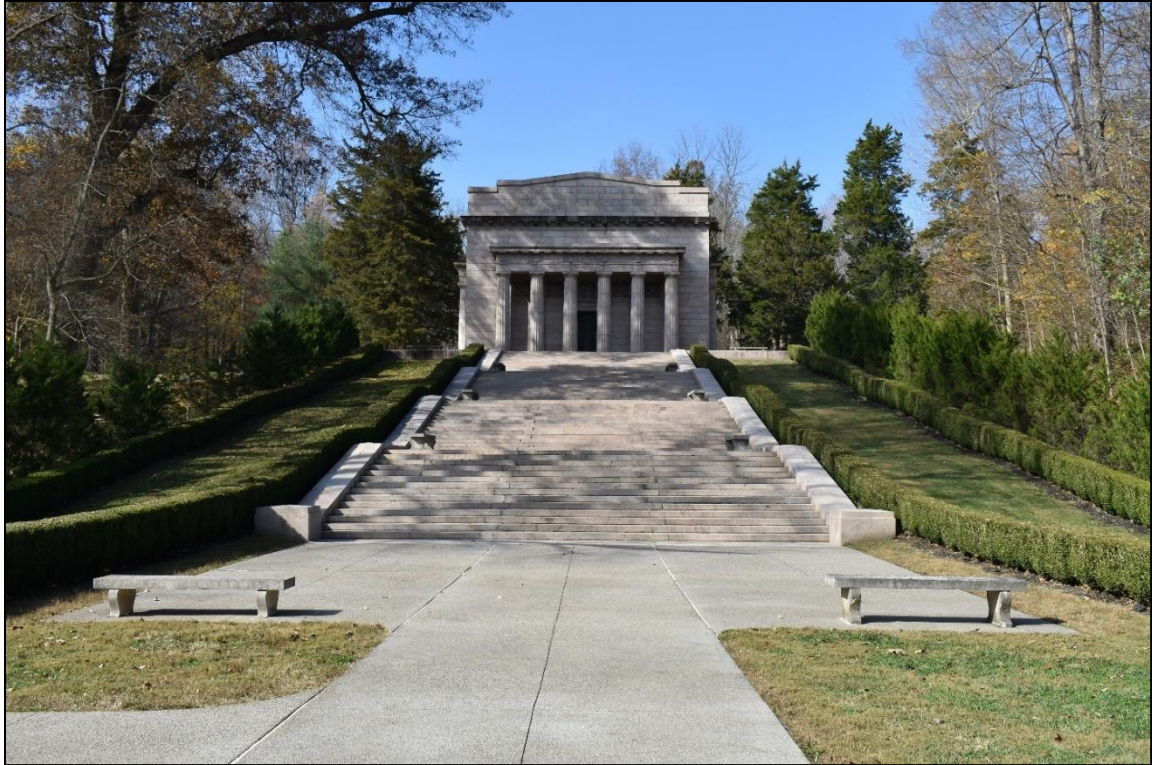
Photograph 23. Overview of the Memorial Building, showing stairway, landscaping, and stone benches, facing northwest.
