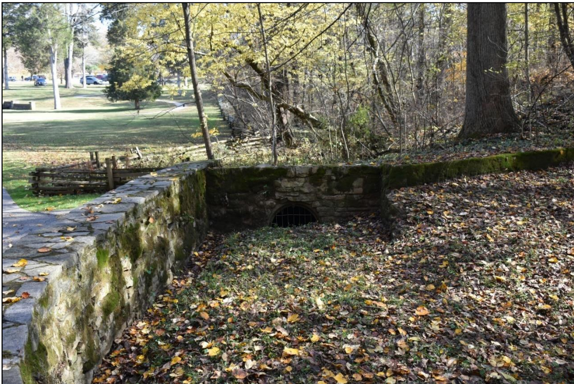
Photograph 18. Overview of the location of the Boundary Oak tree, showing stone retaining wall and culvert and earthen dam, facing west.
