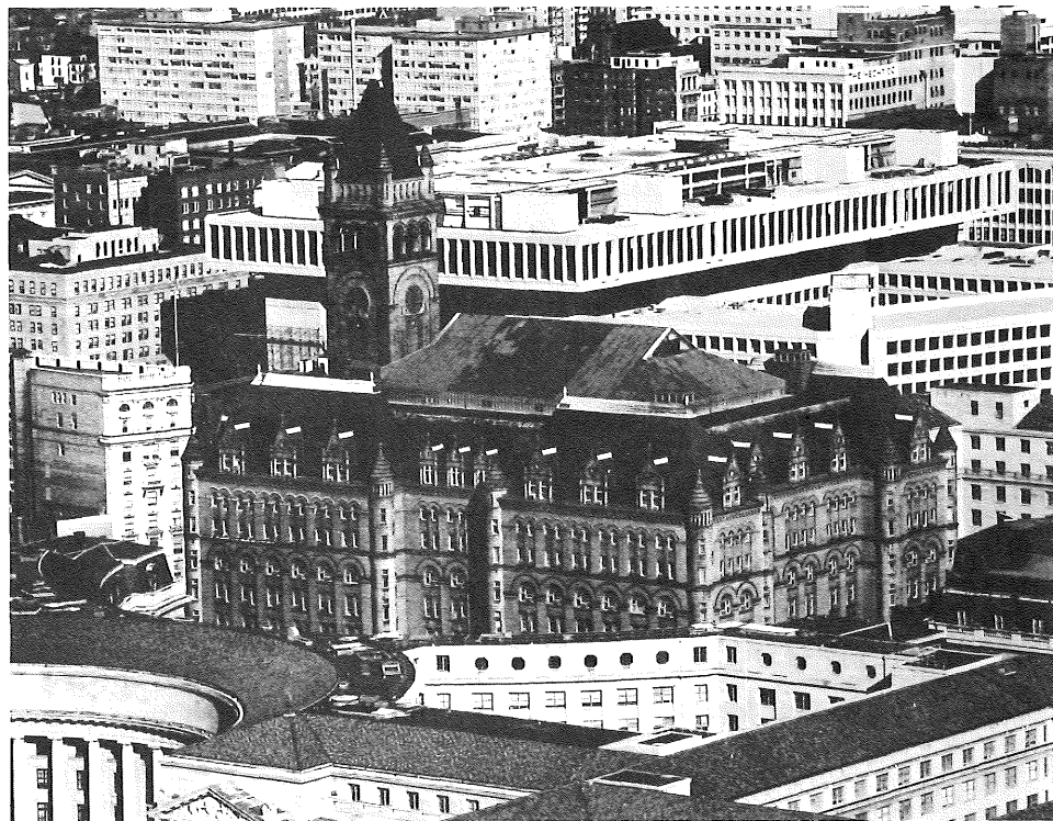
The heavy masonry walls of many of the public buildings constructed in the late 19th century improve the structures' thermal performance. Old Post Office and Clock Tower, Washington, DC.
