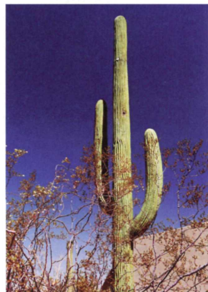
This tower is a saguaro cactus replica designed to blend into the landscape.
