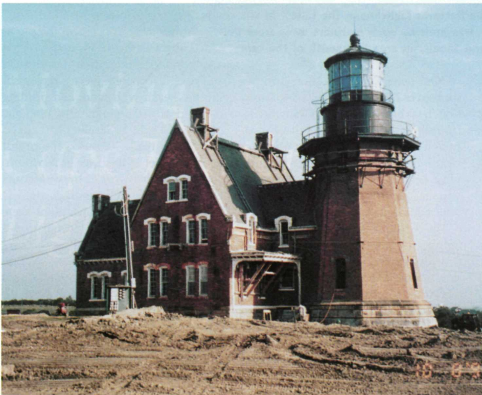
International Chimney and Expert House Movers successfully relocated the 120-year-old Southeast Light on Block Island, Rhode Island, in 1993.
