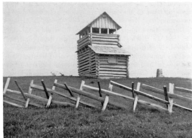
Another type of construction resulted in the "stake-and-bunk" fence, seen directly above on the Blue Ridge Parkway in southern Virginia. At the observation tower on Ground Hog Mountain in southern Virginia a "pitch-pole" fence stands in the foreground.
