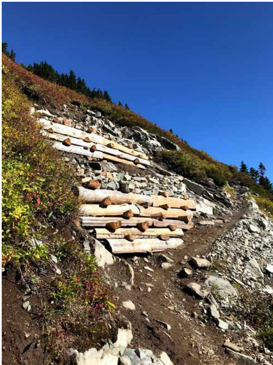
Two timber/rock crib retaining walls now permanently mar the formerly pristine meadows on the slope of Sahale Arm. —PHIL FENNER PHOTO
