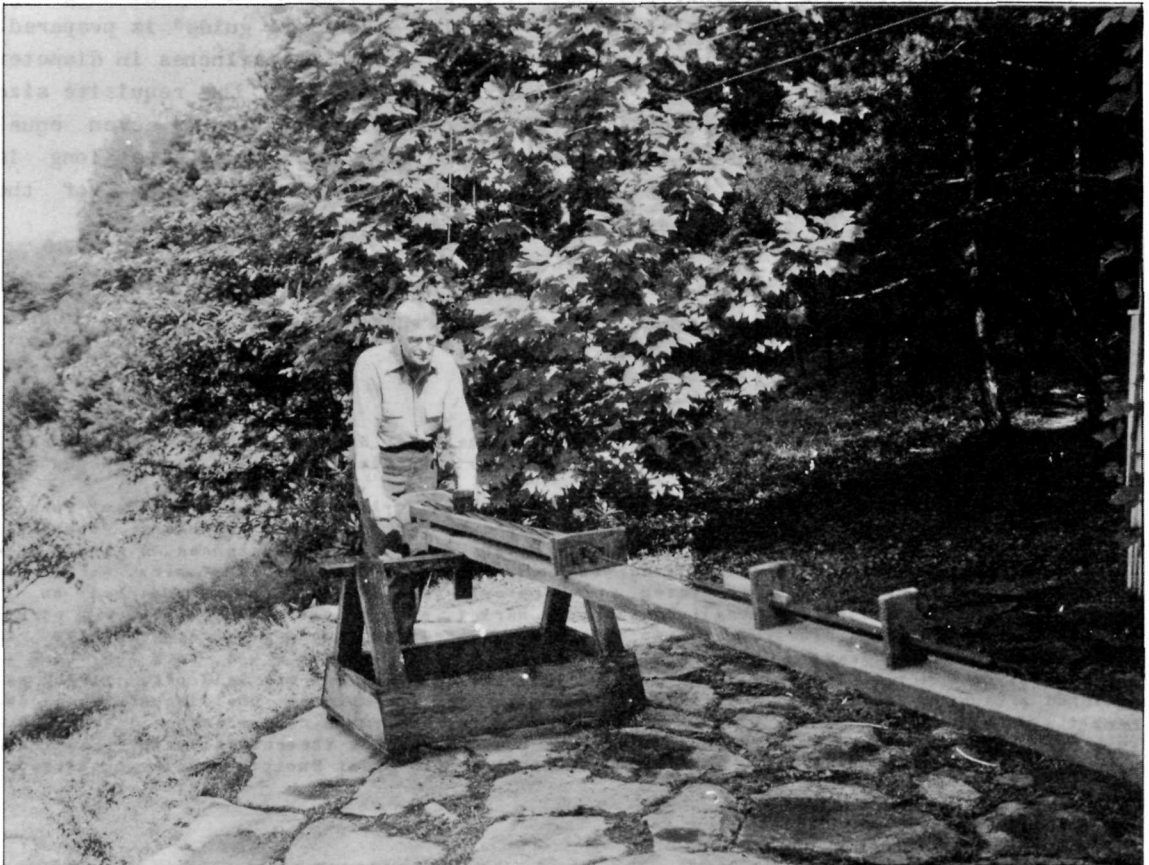
Complete assembly for rifling a gun. Left to right: rifling guide, head block, rifling rod and barrel of rifle.
