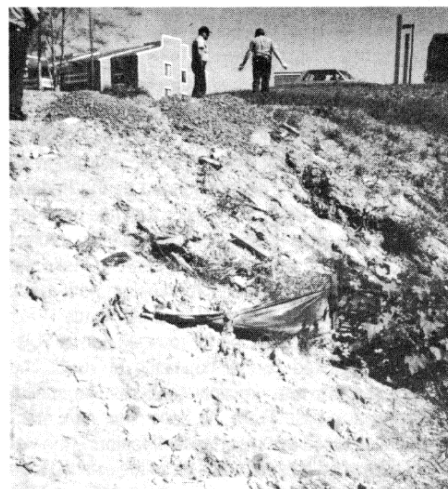
Figure 2. Housing construction can cause erosion, which flows as sediment downstream during storms. This eroded site is only about 100 meters from the park boundary at Richmond National Battlefield Park.
