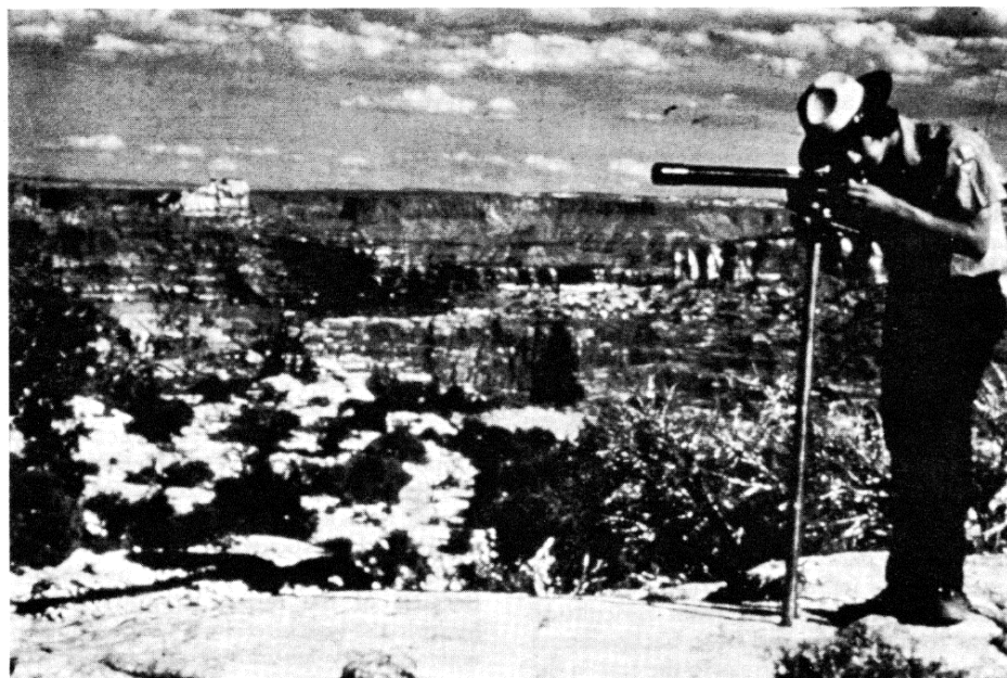
A ranger at Canyonlands NP takes visibility measurements with a teleradiometer.
