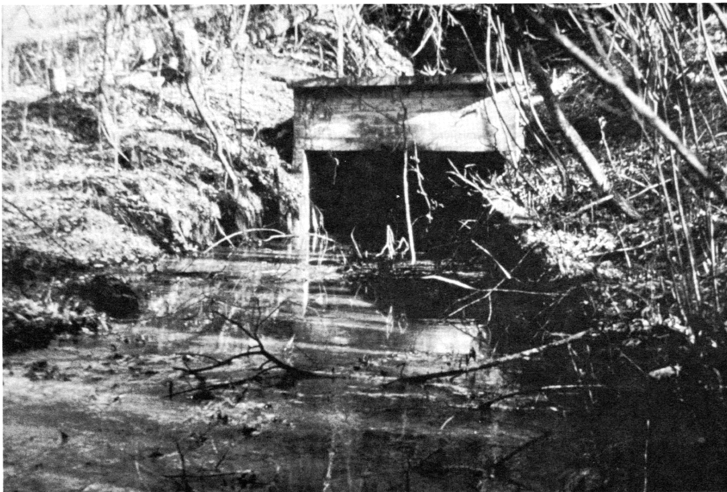
An abandoned mine opening in the Big South Fork NRR produces acid drainage that contaminates nearby streams. This is a widespread problem in the central Appalachians.
