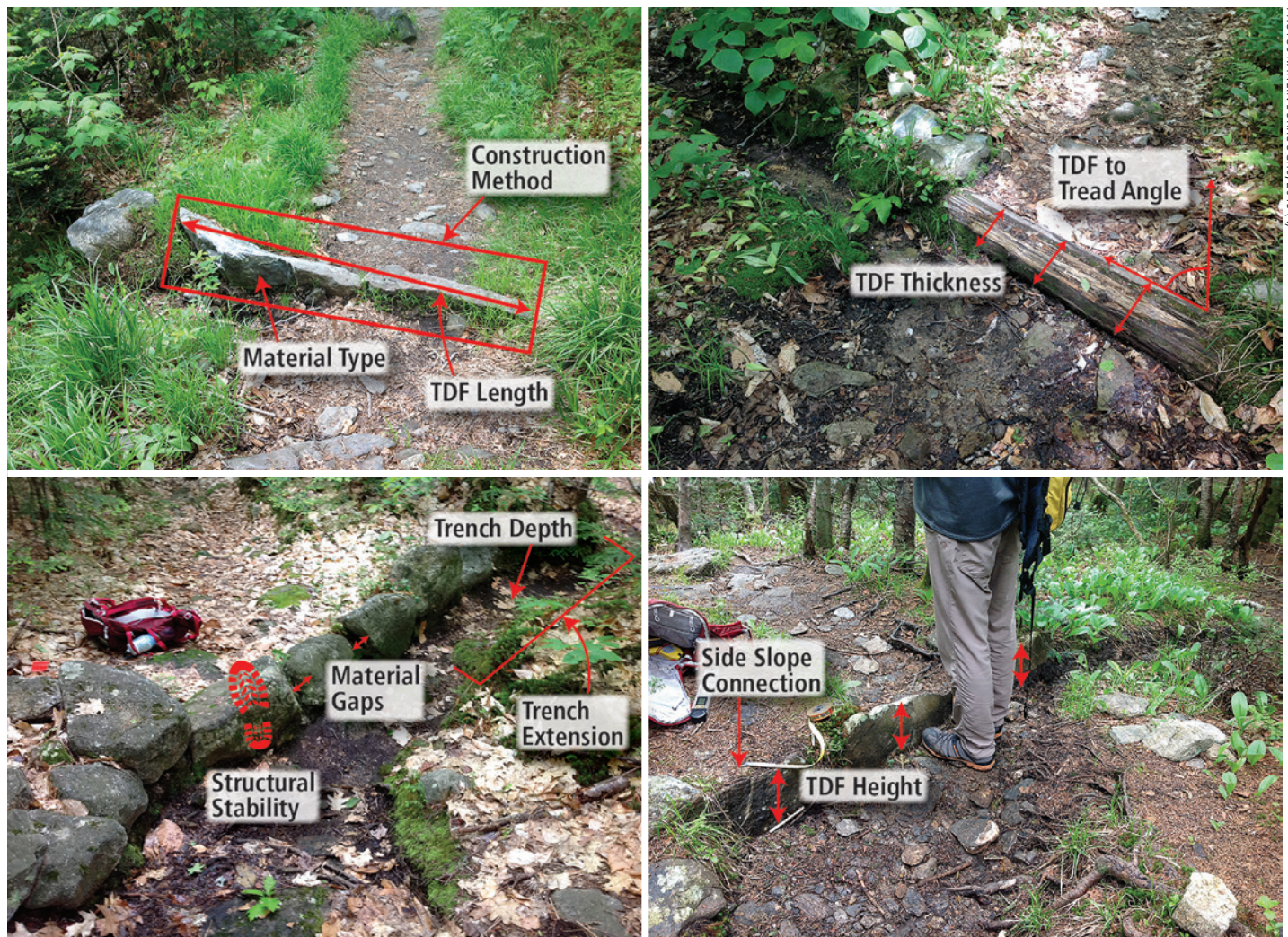
Figure 4. The photo diagram illustrates examples of measurements from the trail drainage feature assessment.
