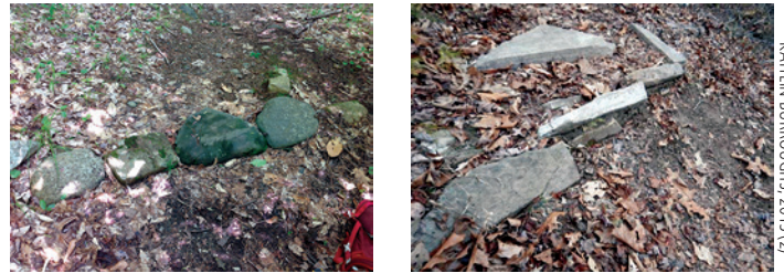
Figure 2. Rock waterbars are often constructed using different methods. Shown here are flush (left) and stacked under (right).
