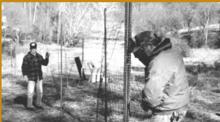
Figures 3 (left) and 4. Project staff construct enclosures to protect woody vegetation planted in 20- and 40-foot-diameter clusters so that they will not be eaten by deer. Riparian vegetation stabilizes the soil and increases infiltration of storm water runoff. It also provides food and habitat for aquatic and terrestrial animals.
