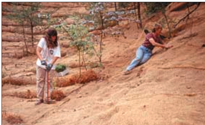
Figure 1. The site at Oxon Run was stabilized with coconut "bio-logs" and matting.
