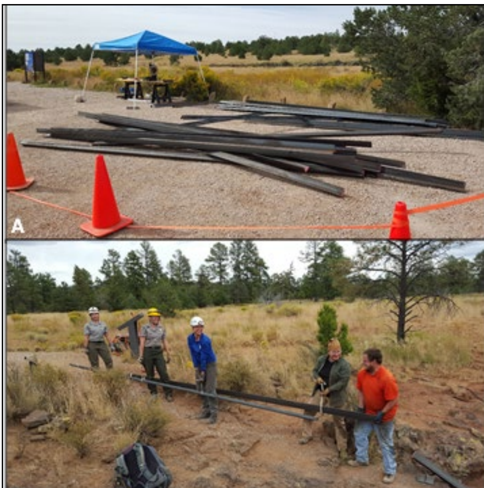
A) Four tons of steel was delivered to the El Calderon parking area for the construction of the bat gate. This consisted of 20ft beams weighing between 200 to 800 pounds. B) NPS Staff Melisa Bishop, Laura Baumann, and Nikki Woodward carrying a 20ft beam to the cave entrance, and Lydia Hernandez and Graham Schindel getting ready to help carry another beam into the entrance. Photos courtesy of Dave Decker.
