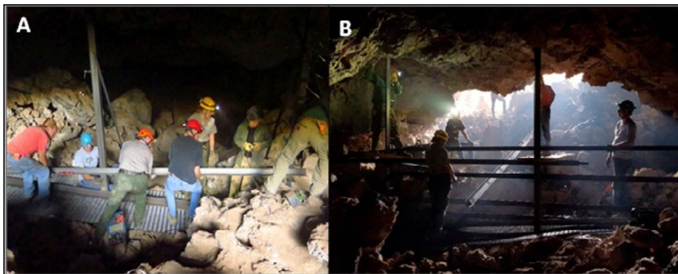
A) The crew lowering one of the 200 pound steel beams during the early stages of the bat gate construction. From left to right: Jim Kennedy, Dave Decker, Eric Weaver, Scott Christenson, Laura Baumann, Lydia Hernandez, and Kevin Lorms. B) Another steel beam was carried into the cave for the upper section of the gate. From left to right: Kevin Lorms, Laura Baumann, Scott Christenson, Jim Kennedy, and Dave Decker. Photos courtesy of Melisa Bishop (A) and Dave Decker (B).
