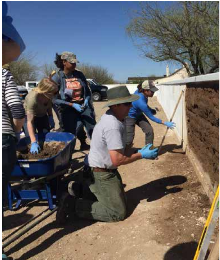
Figure 3. Participants from TICRAT 2016 repair an adobe wall with mud infill prior to replastering (NPS photo 2016).
