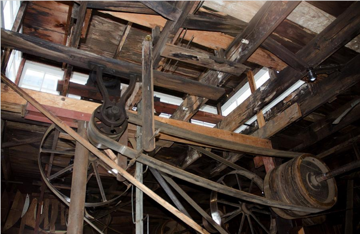
Kregel Windmill Company Factory NHL, Nebraska City, Nebraska. (Photograph by David Calease.)
