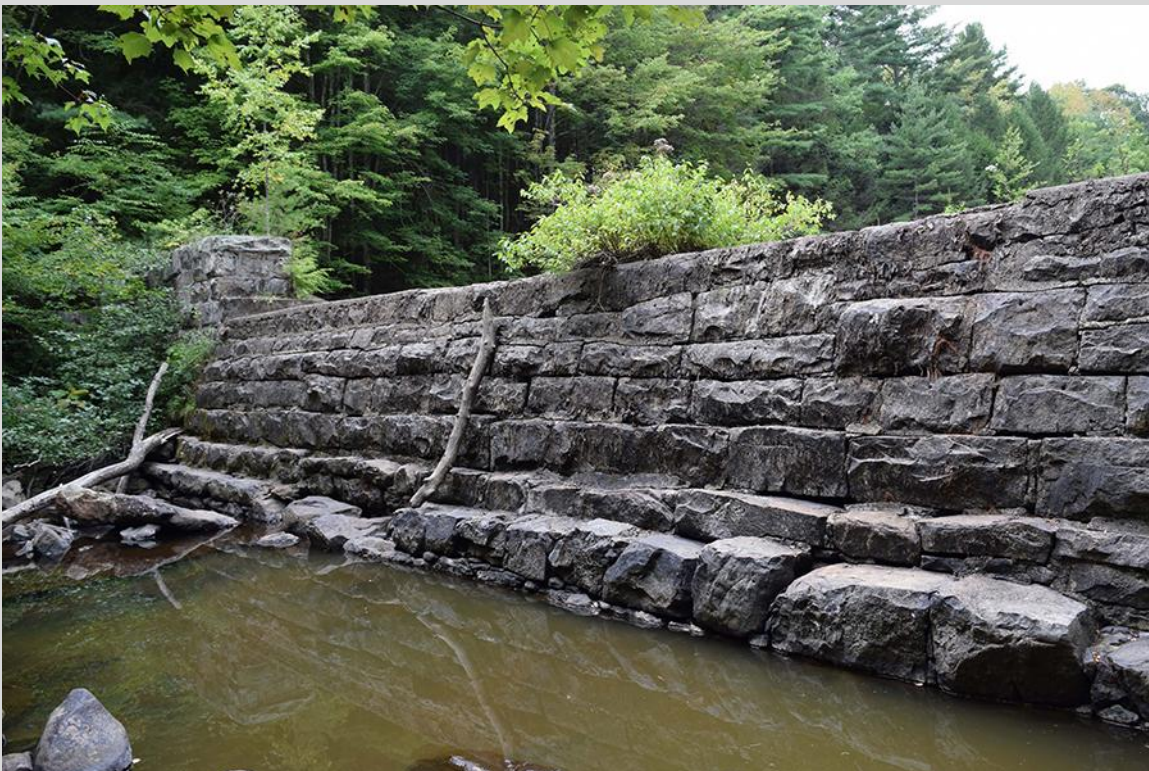
Winsted Water Works, Mad River Diversion Dam, Winsted, Connecticut. (Photograph by Gretchen Pineo, John Daly.)
