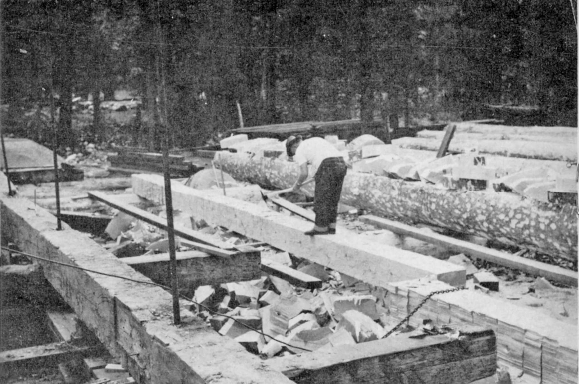
Timbers were shaped by hand.
