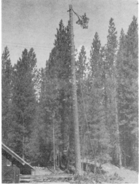
Topping tree for bridge supports.
