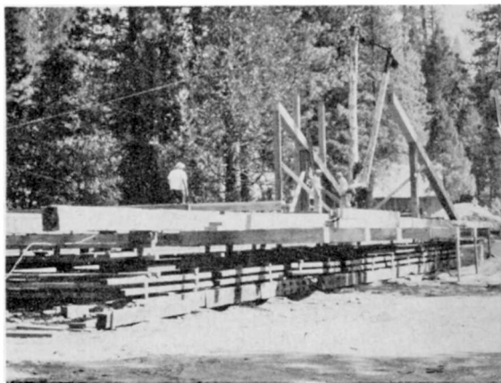
Replacing the timbers called for special skills.
