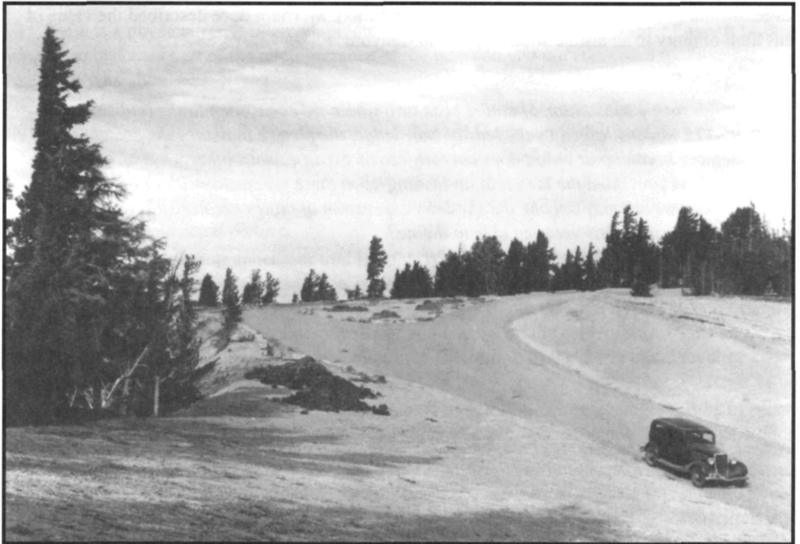
Reflection Point, a substation on the east Rim Drive.
