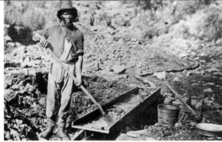
A black placer gold miner shovels paydirt at Auburn Ravine in 1852. BANCROFT LIBRARY
