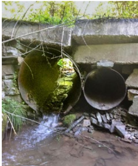
The original fish passage structure on a tributary to Blue Lick Run was decaying and ineffective. The larger opening allows for fish passage and a bridge over the stream safe for vehicular traffic. (PHOTO BY TROUT UNLIMITED)
