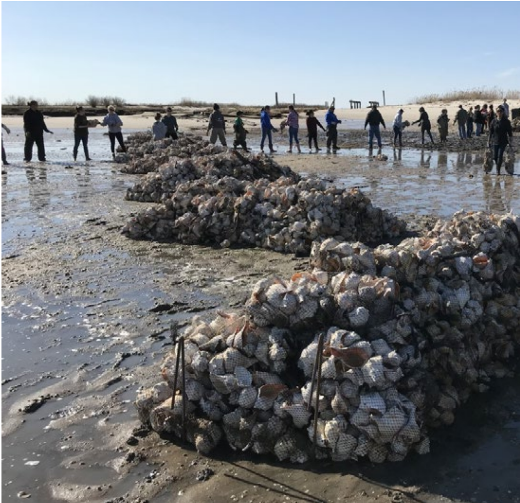
(Above) Over 25,000 shells were bagged by locals, partners, and the Service, to make breakwaters in an effort to stabilize the sand. (PHOTO BY DANIELLE MCCULLOCH PROSSER/USFWS)
